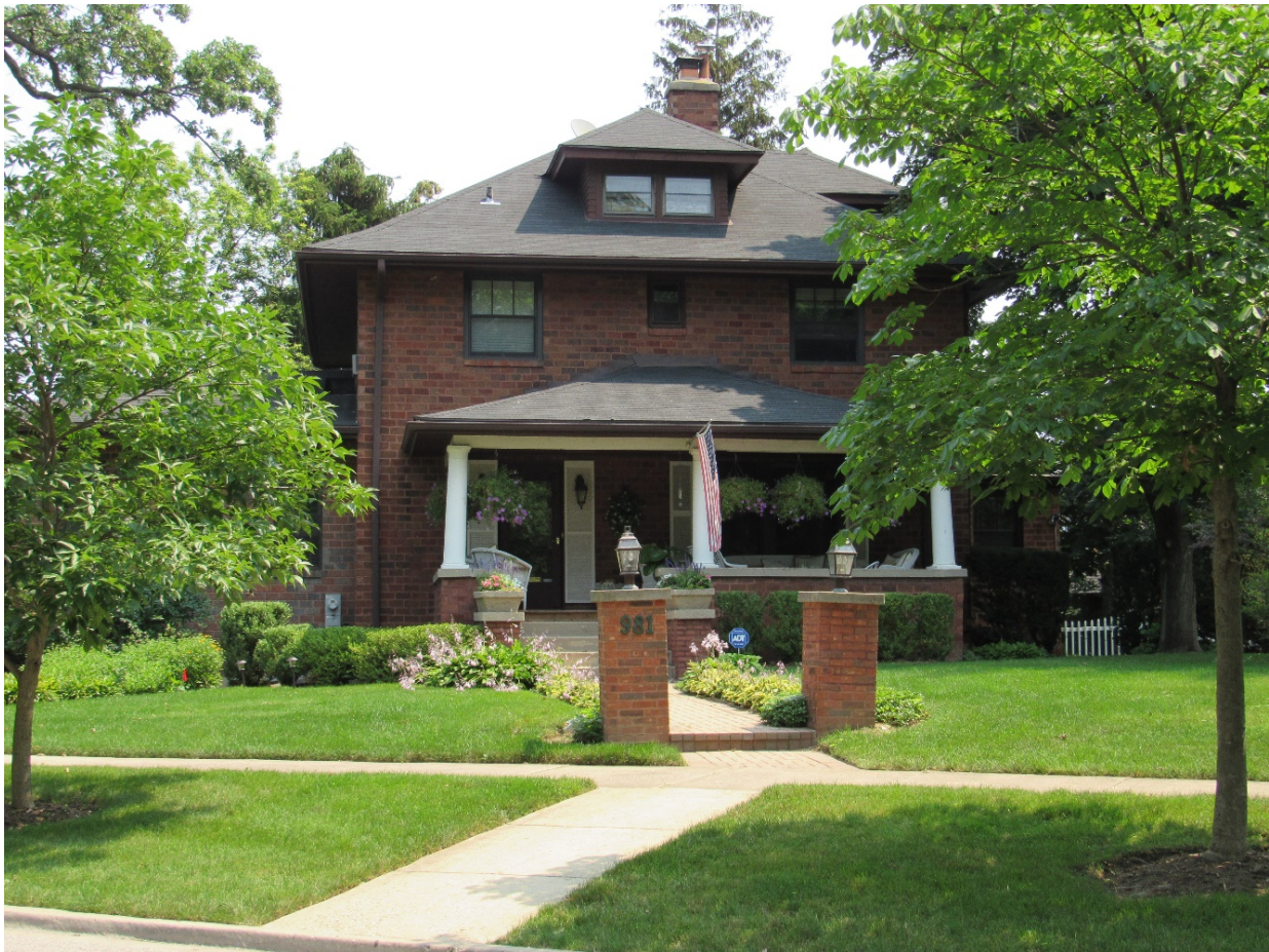
Figure 3 – Subject Property – Front Elevation (Gordon Terrace)
