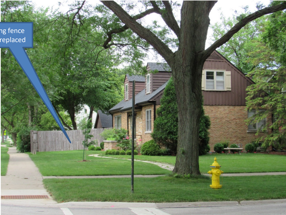
Figure 3 – Subject Property – South Elevation (Ash Street)
