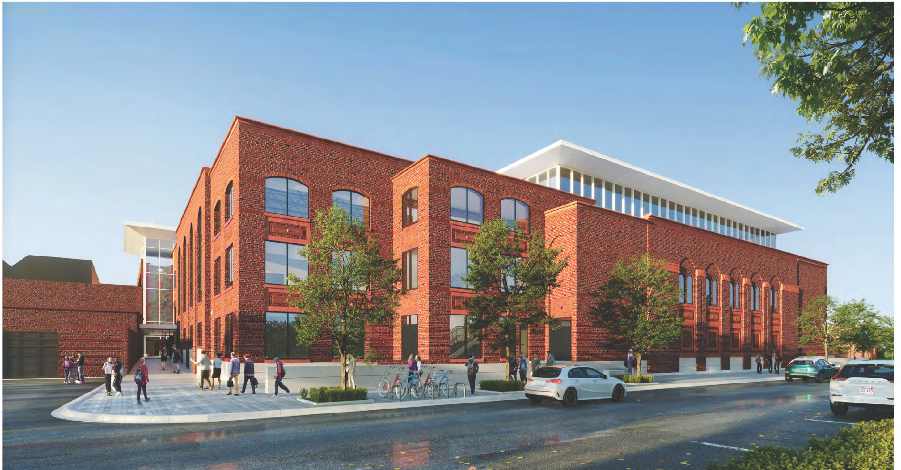
EAST ELEVATION LOOKING WEST FROM ESSEX
