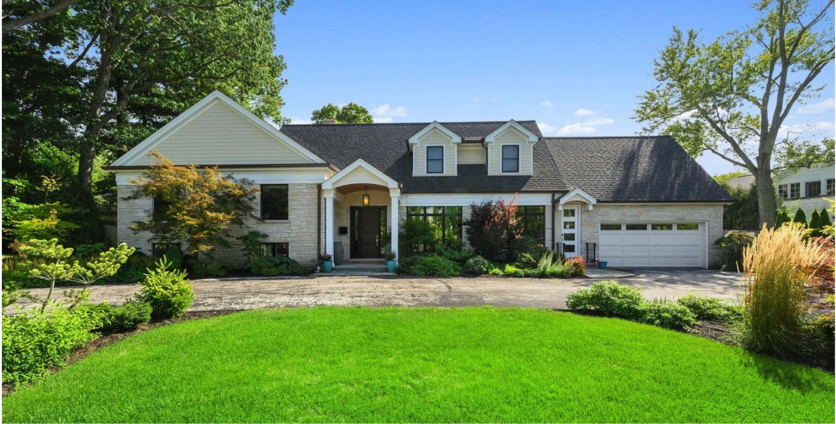
FRONT OF HOME- NORTH
