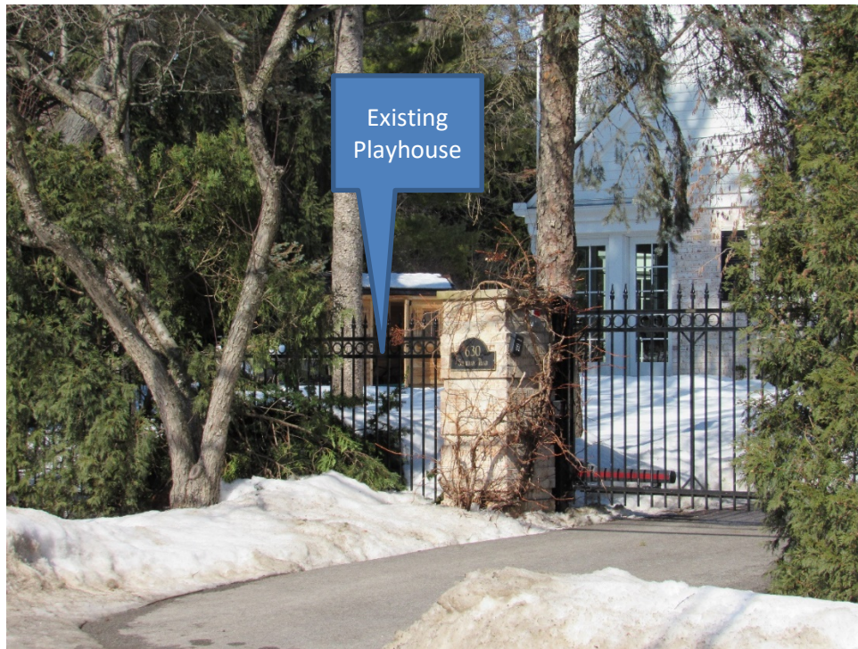
Figure 3 – Subject Property – (view from Pine Street looking northwest towards playhouse)
