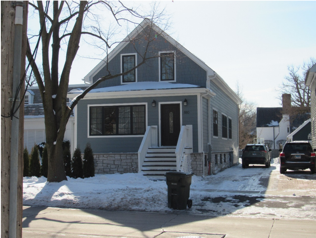
Figure 3 – Subject Property (North Building Elevation)
