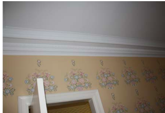
Detail of dining room crown molding
