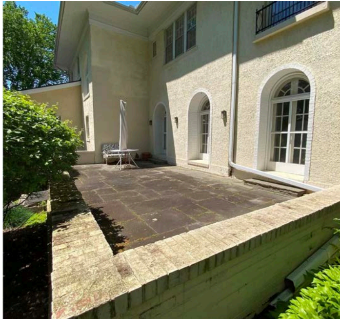
South elevation, looking west Zillow.com, accessed August 13, 2020
