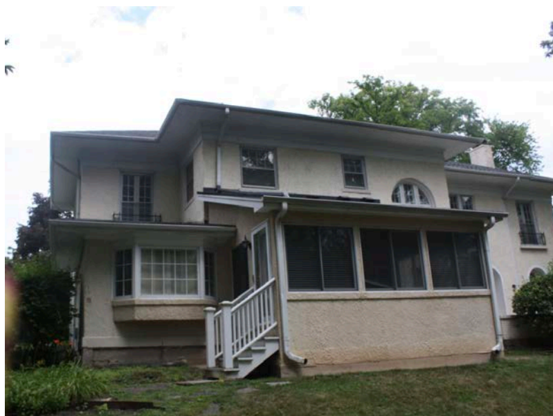
South elevation, looking north
