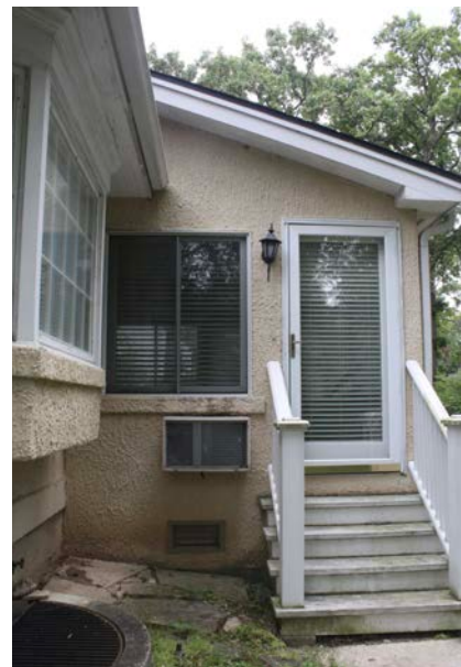
West elevation of addition, looking east
