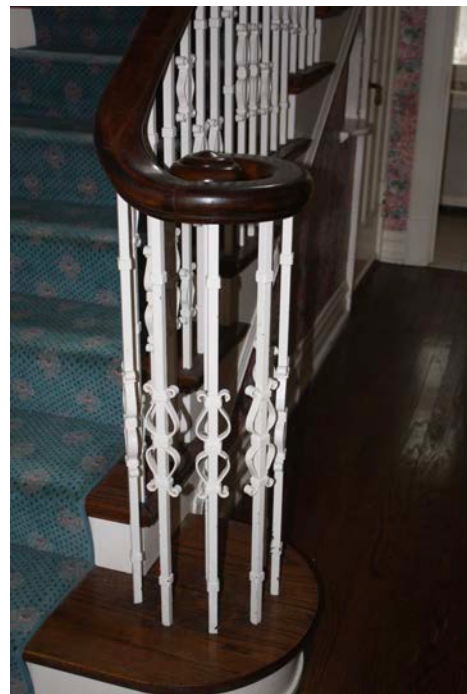
Detail, front stairs
