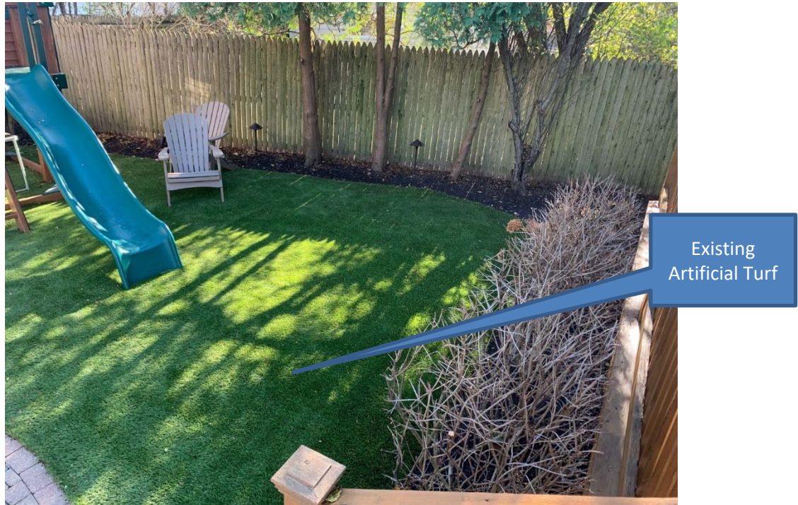
Figure 5 – Existing Artificial Turf in Rear Yard
