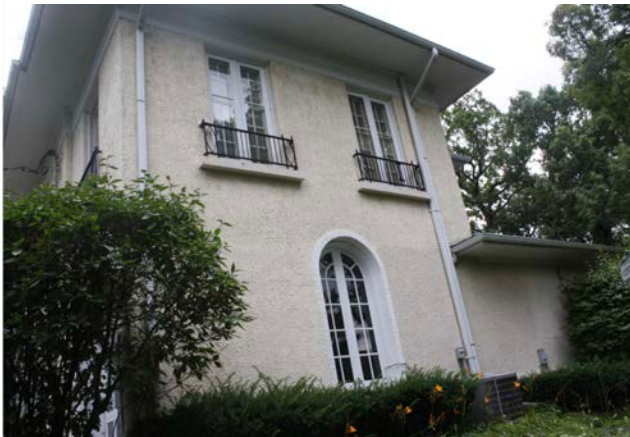
West elevation, looking east
