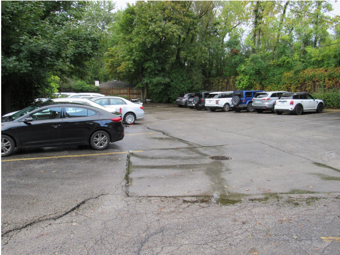
Figure 2 – Subject Property – Southern Portion of Parking Lot
