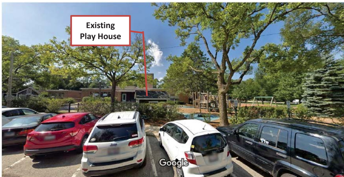
Figure 1 – Subject Property (looking west from Glendale Avenue)
