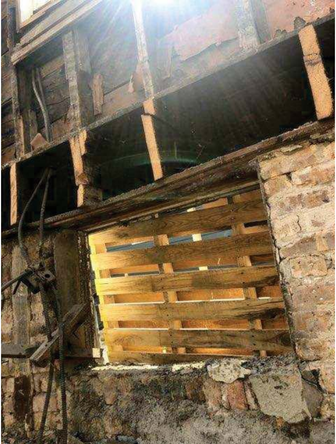
EXISTING WEST SIDE EXTERIOR WALL
