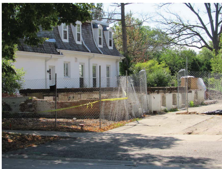
Figure 2 – Subject Property – Existing Condition
