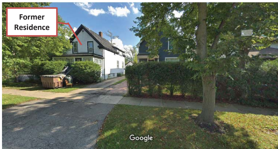
Figure 1 – Subject Property Prior to Demolition
