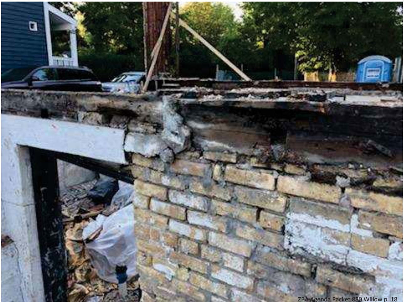
EXISTING SOUTH SIDE BRICK WALL
