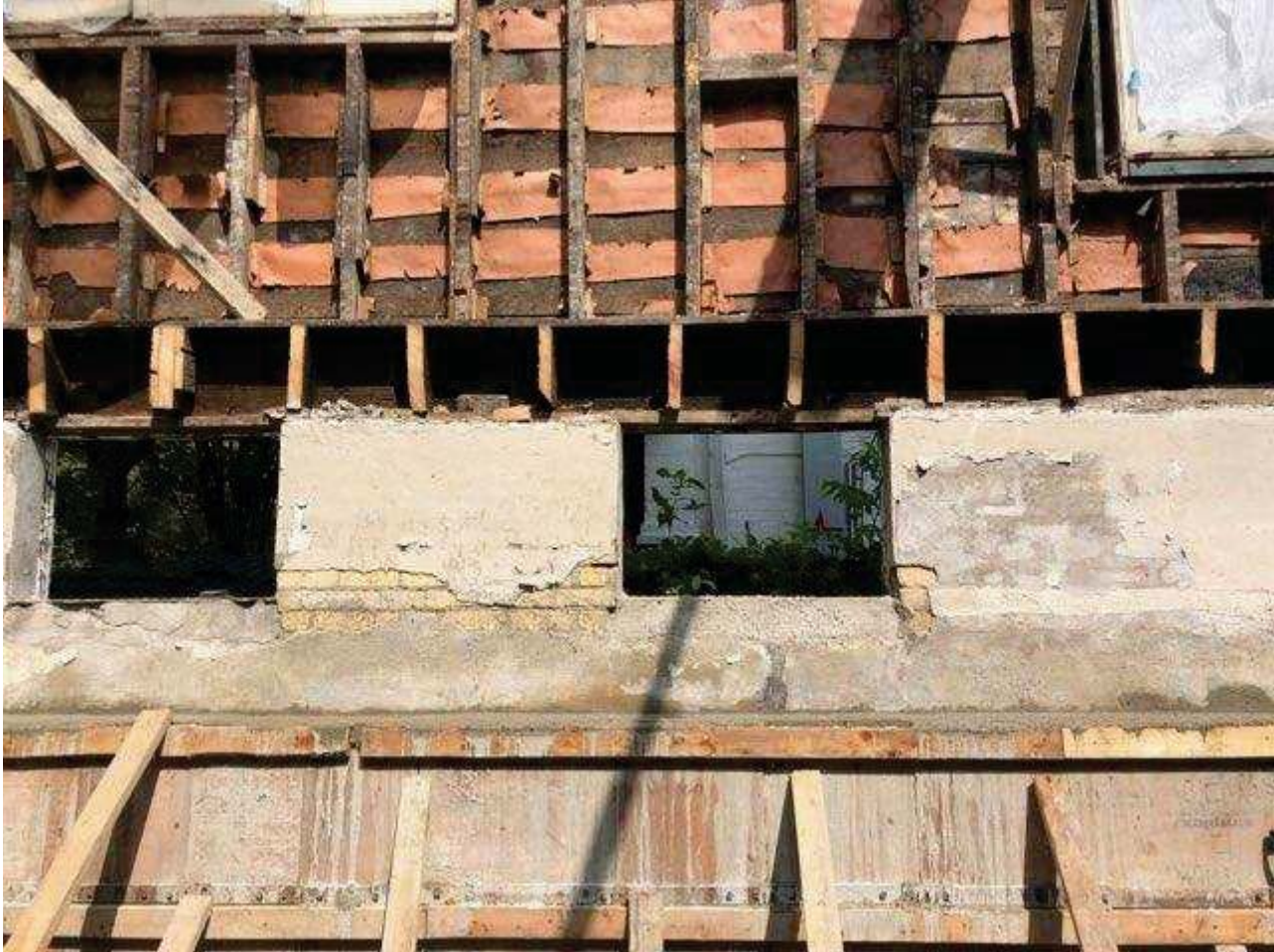
New concrete around interior perimeter for existing foundation reinforcement.
