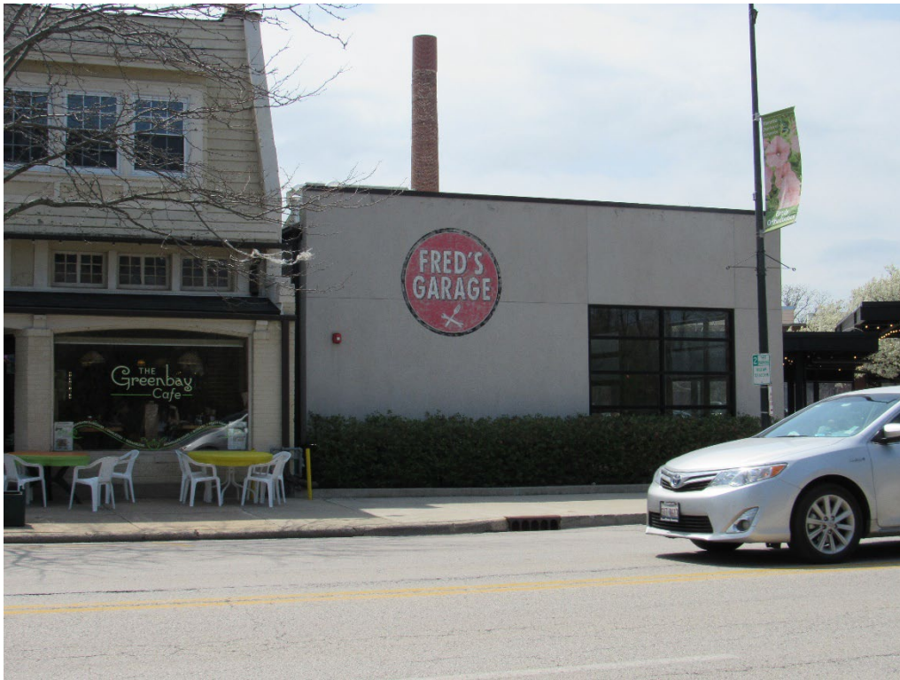
574 Green Bay Road (restaurant to north)
