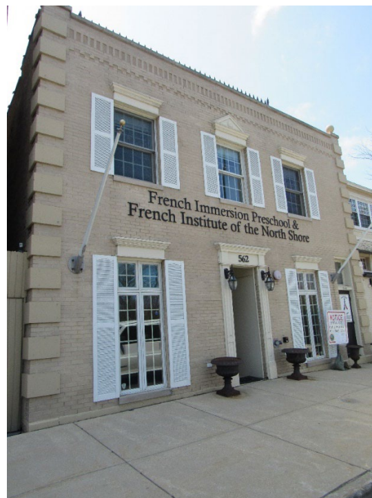
Figure 2 – Subject Property – Existing Front Building Elevation
