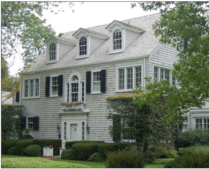
Wood shingles are traditionally used as primary materials for exterior walls and are one of the preferred materials for new construction.
