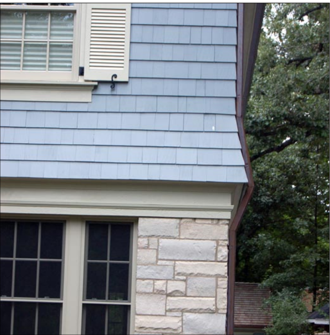
A molding is used to separate the two primary facade materials.
