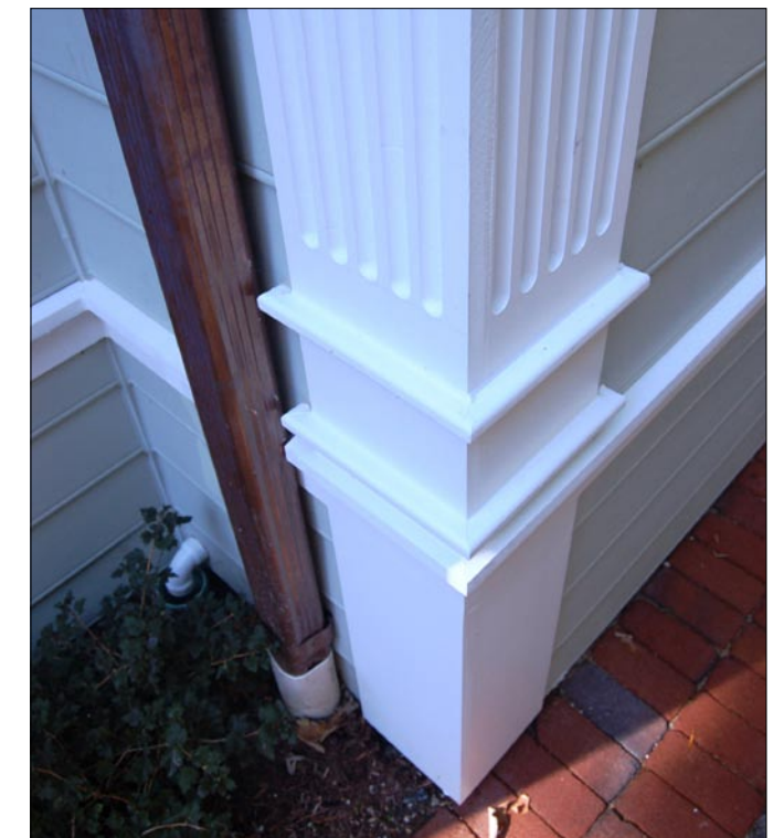
Fluted corner boards are proportional to horizontal siding and exhibit a high level of detail and fine craftsmanship.
