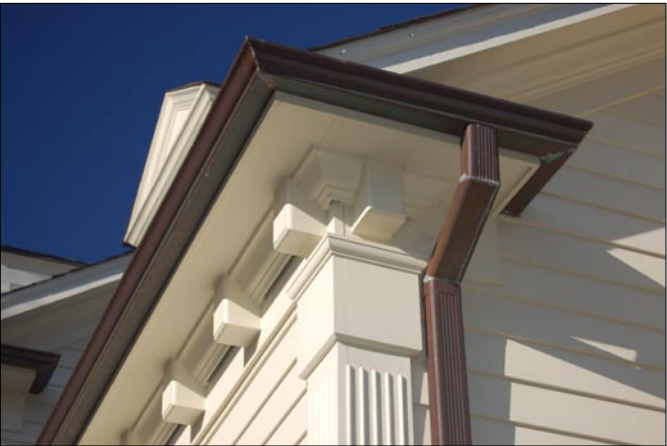
Attention to detail is evident in this eave overhang. Eaves return around the gable end, and the underside includes a built-up molding with dentil bracket details.
