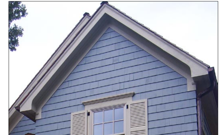
Fascia board beneath gable “supports” roof visually, and is proportional with rake board.
