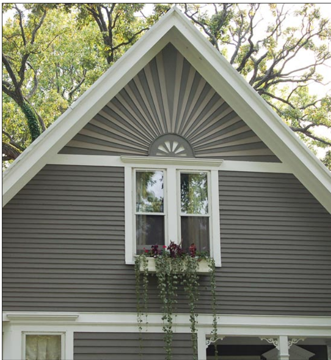
Patterned trim creates visual interest on this gable-end facade and is consistent with the style.
