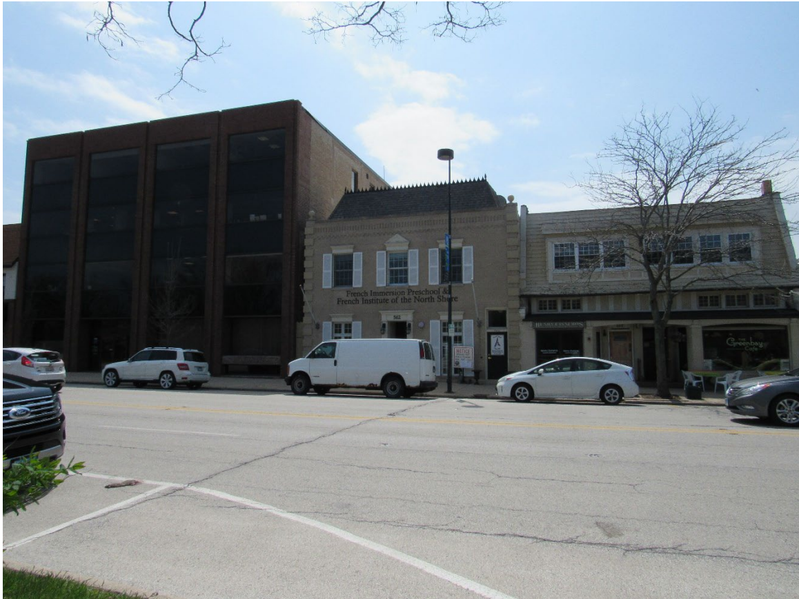
Figure 3 – Subject Property with Neighboring Properties
