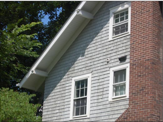
Generous eaves are appropriate to the building style, and are integrated into the overall design through use of “expressed beams” which serve to support the roof both structurally and visually.
