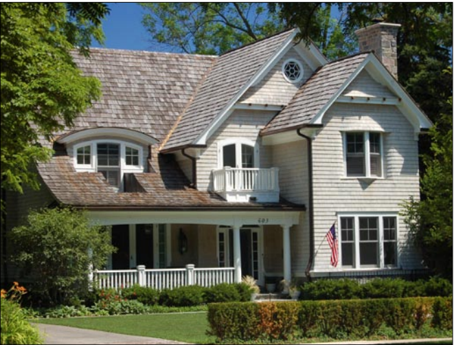
Cedar shingles and siding, wood windows and high quality exterior trim carpentry is sympathetic toward other frame homes in the neighborhood, helping it blend in gracefully. The long slope of the roof line establishes an intimate scale and terminates at an inviting, well detailed front porch, creating a welcoming appearance from the street.
