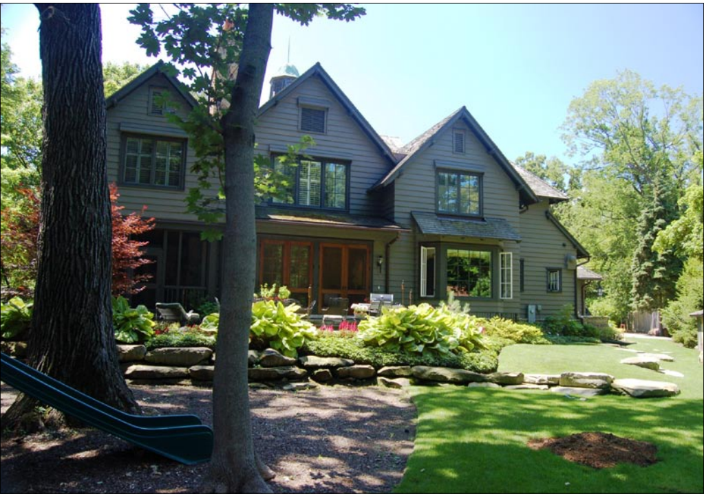
Minimize disruption to existing grade to prevent damage to mature trees. A severe grade change on this site was managed in a natural fashion utilizing natural stone outcropping to retain the slope and avoid a more severe retaining wall.
