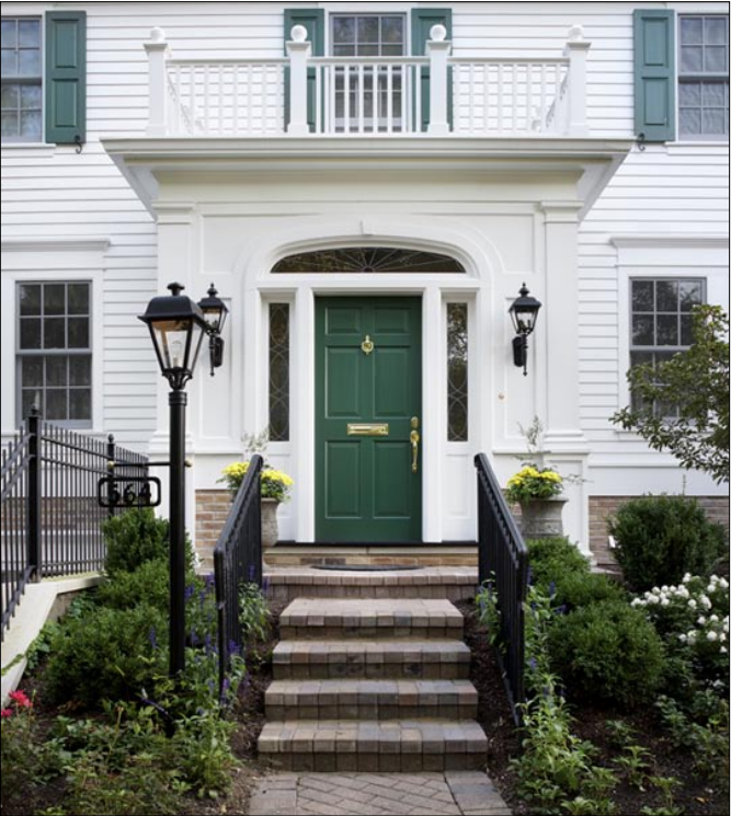
This entry conveys a sense of human scale though the use of transom windows, lighting features and stairs.
