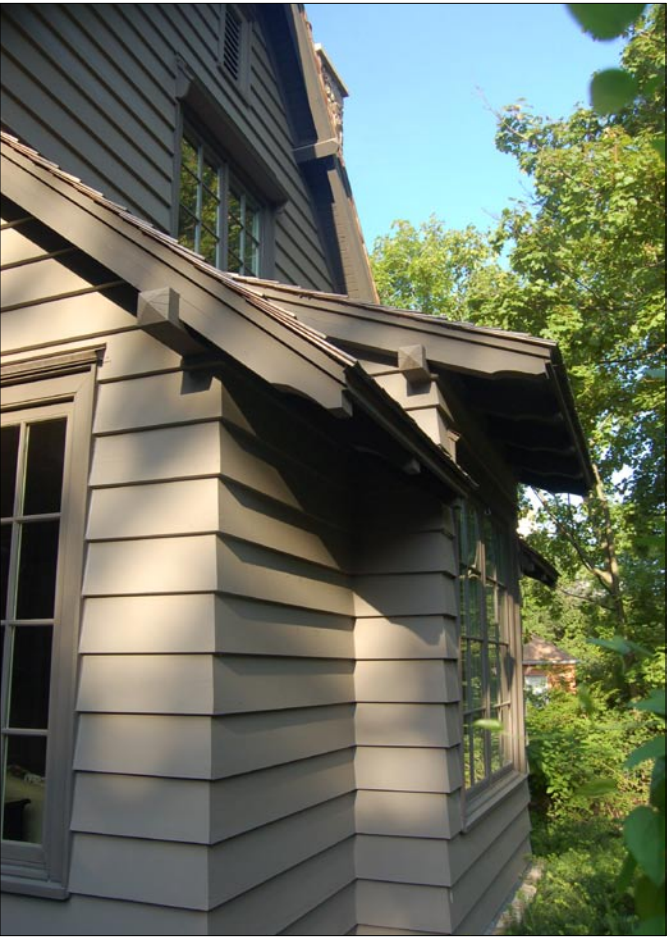
Traditional clapboard siding and muted earth tones integrate this new home seamlessly with the neighborhood and surrounding landscape. Elements such as expressed beams and exposed rafter tails express a sense of craftsmanship and attention to detail.
