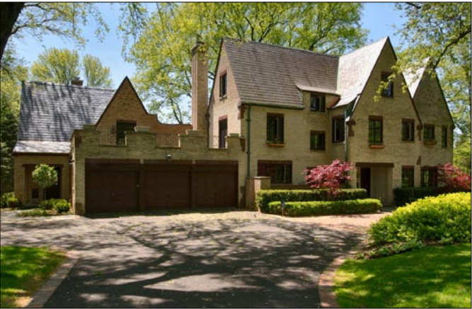
A steeply pitched gable roof is appropriate in this setting, on a larger house setback a considerable distance from the street and its neighbors. Variations in building mass translate into an attractive, sculpted roof form.
