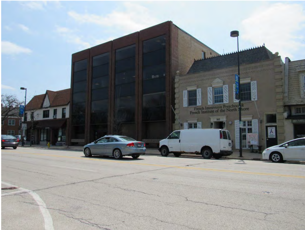
Subject Property with Neighboring Properties to South
