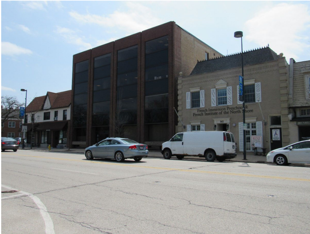
Subject Property with Neighboring Properties to South
