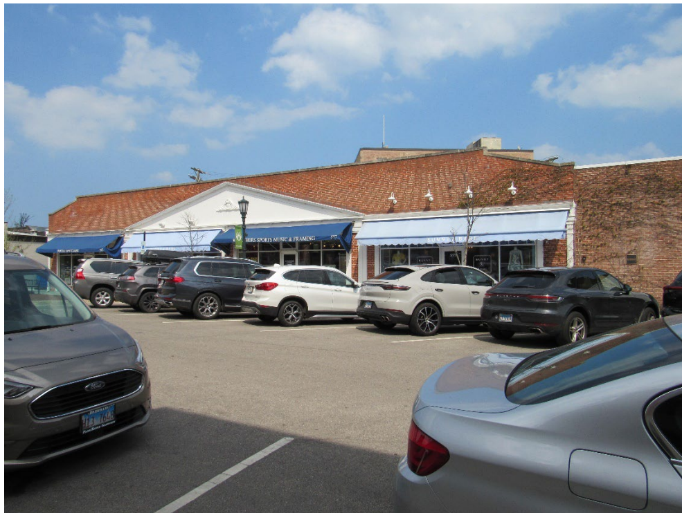
555-571 Chestnut Street (commercial building to west)
