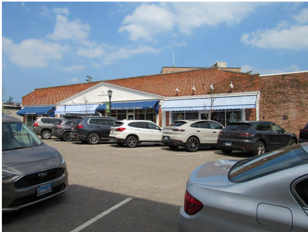
555-571 Chestnut Street (commercial building to west)
