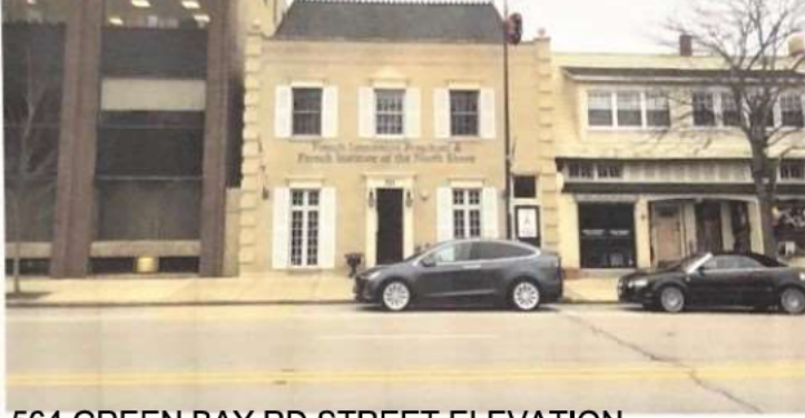
564 GREEN BAY RD STREET ELEVATION
