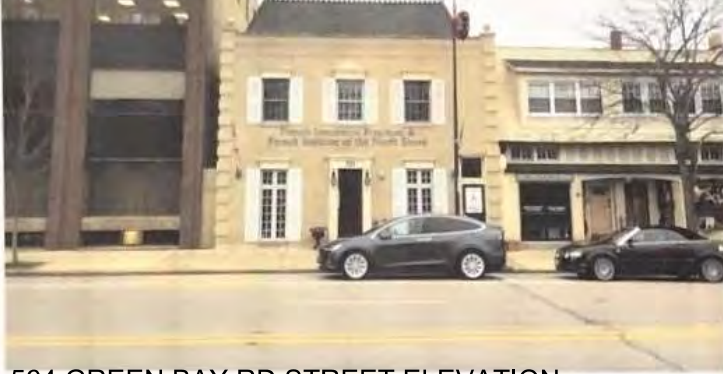
564 GREEN BAY RD STREET ELEVATION
