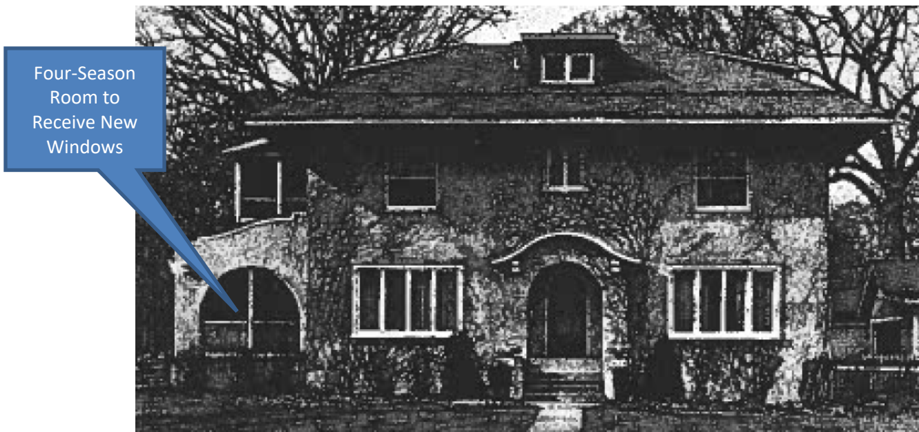
Figure 2 – Subject Property – Original South Building Elevation prior to installation of existing sliding doors and windows
