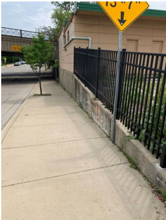
North Side of 93 Green Bay Road Building (Note: retaining wall)
