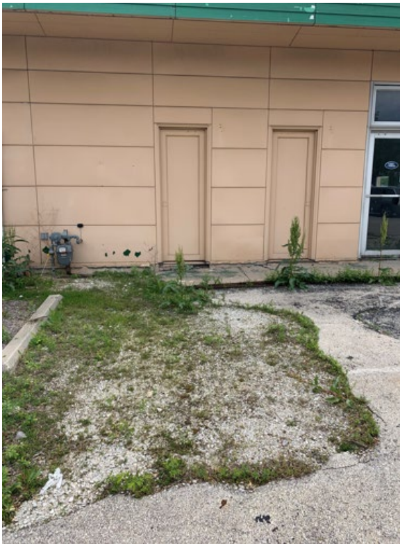
West Side (north end) of 93 Green Bay Road Building
