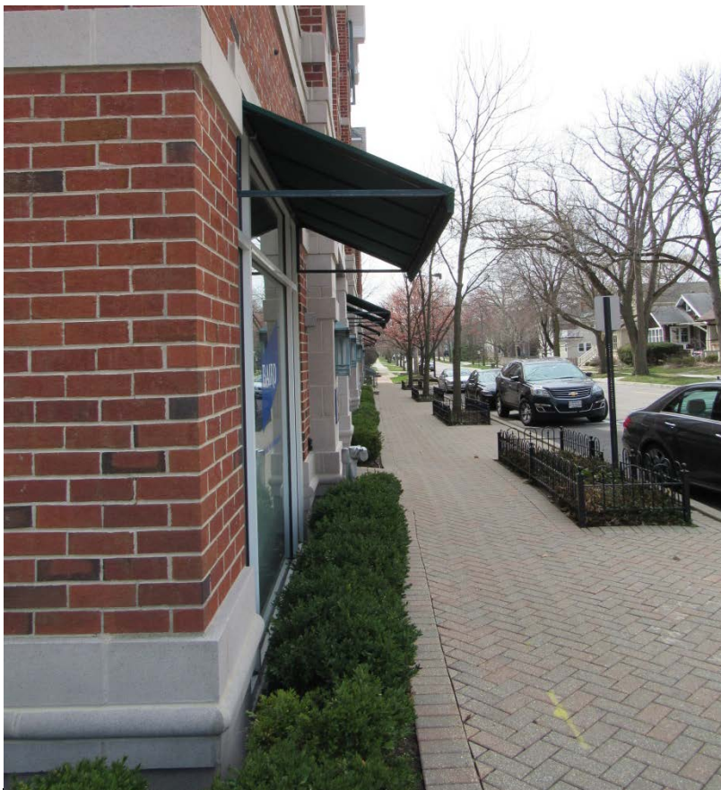
Figure 5 –Awning frame up close
