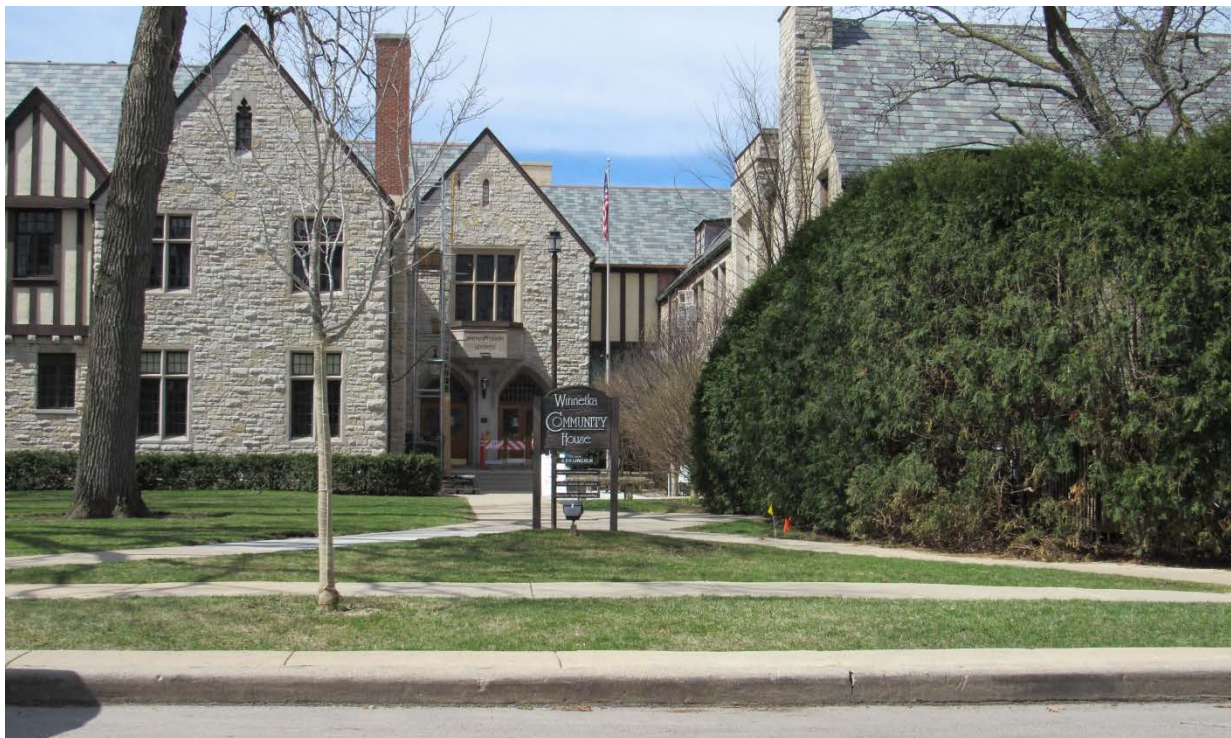
Figure 4 - Directory sign along eastern street frontage of Subject Property
