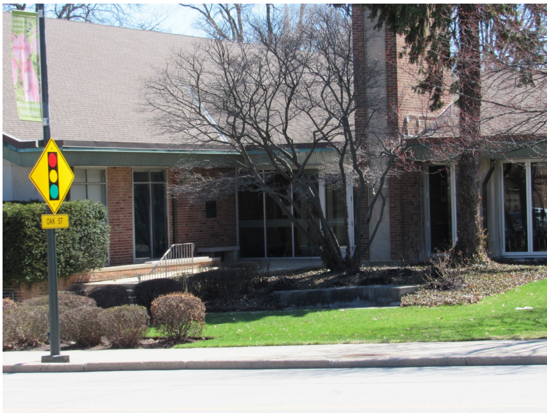
Figure 3 – Existing North Entrance
