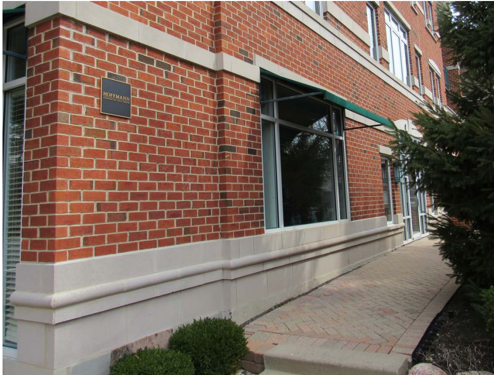
Figure 4 – Awning on south face of building.
