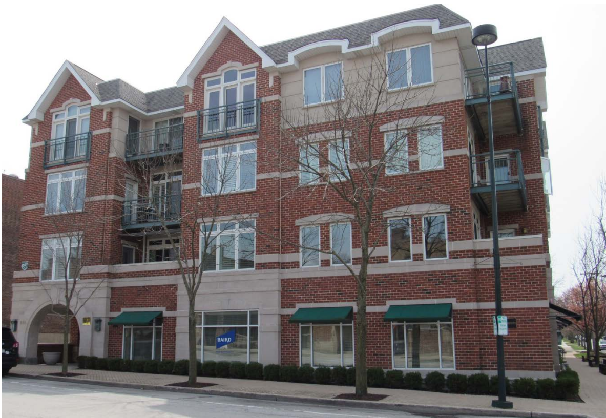
Figure 1 – Subject Property – North Elevation
