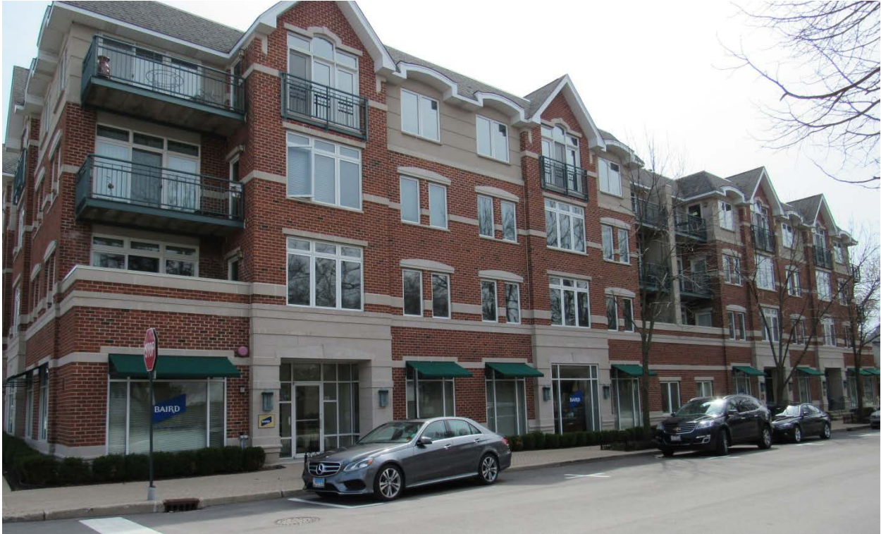
Figure 2 – Subject Property – West Elevation
