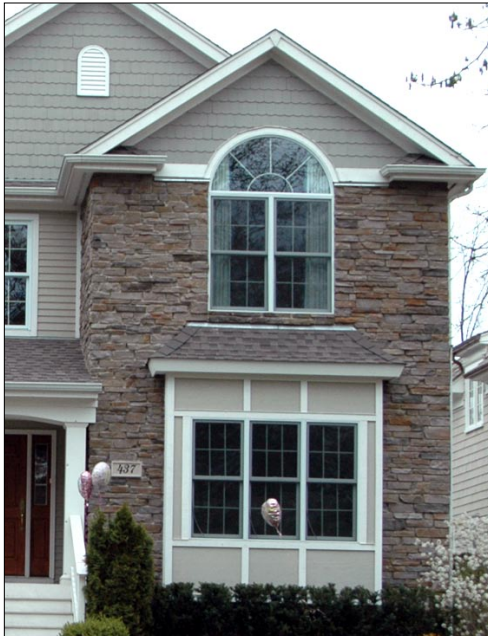
Four materials are used on this facade: wood siding, shingles, stone and stucco with wood trim. This creates a busy facade, increasing the apparent scale of the building.
