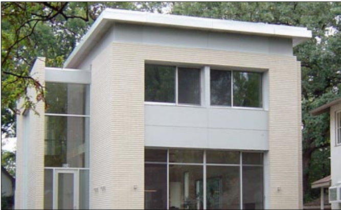
Contemporary Flat Roof
