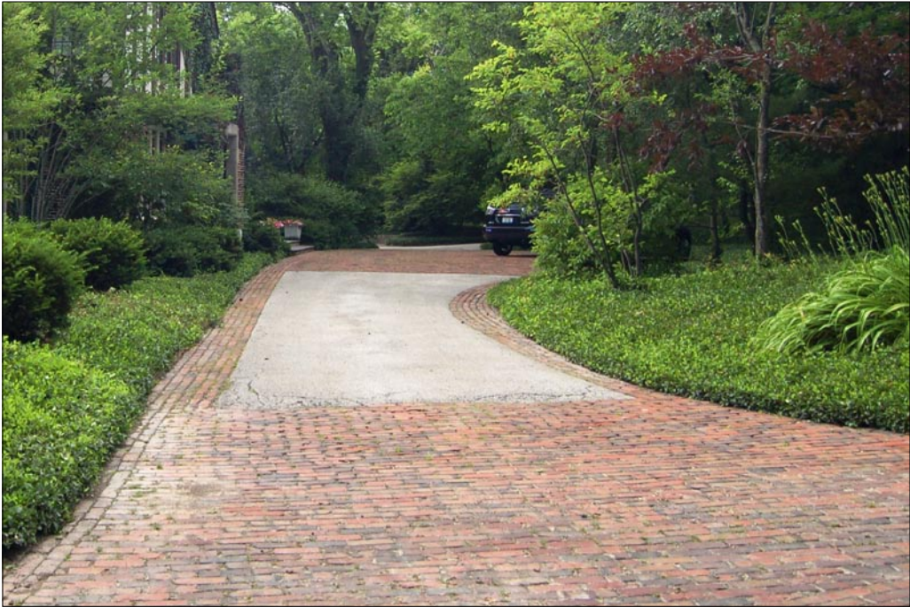
This driveway uses stone pavers which are visually appealing and help to reduce the extent of surface areas. Landscape features also help to screen the drive from view and integrate it into the site.
