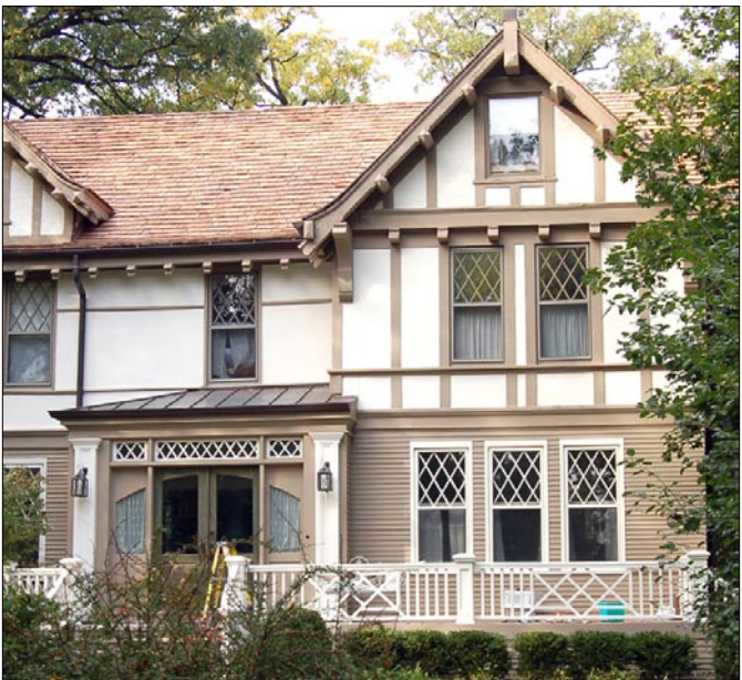
Rafter tails and purlins in the eaves and the half-timber siding help to establish a sense of proportion and scale across a facade.
