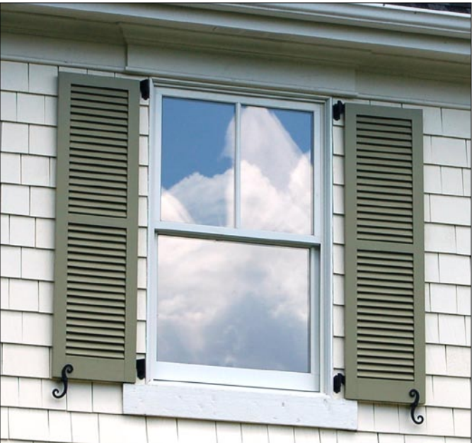
Shutters are proportional to window opening; operable hinges and hardware provide additional dimension of detail and authenticity.
