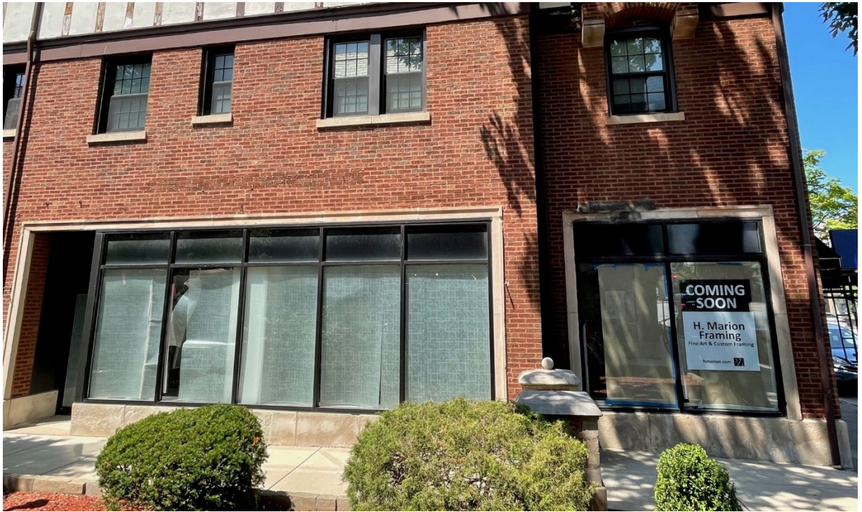
Figure 4 – Subject Property – Store frontage of south building façade along inner courtyard
