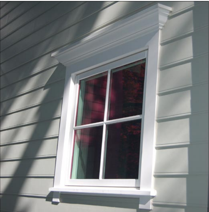
In lieu of shutters, window is detailed with wider flat casing and head molding. Joinery at sill and side casings demonstrates fine craftsmanship and attention to detail.
