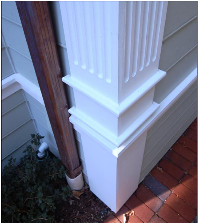
Fluted corner boards are proportional to horizontal siding and exhibit a high level of detail and fine craftsmanship.
