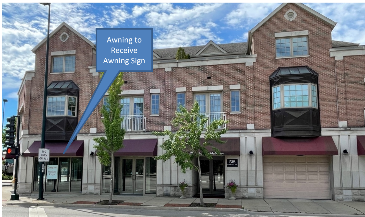
Figure 3 – Subject Property – North Elevation along Winnetka Avenue
