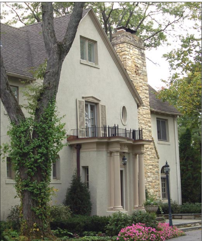
Chimney is integrated into the overall building design.
