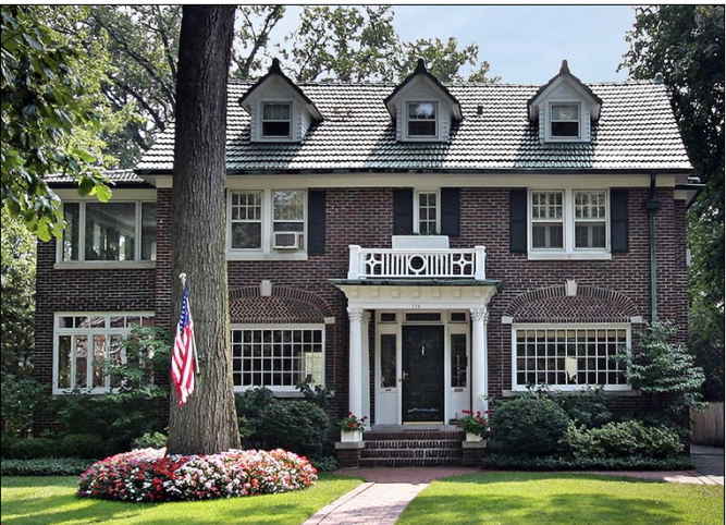
Dormers are proportional to the roof form, and appropriate to the Colonial style of the building.
