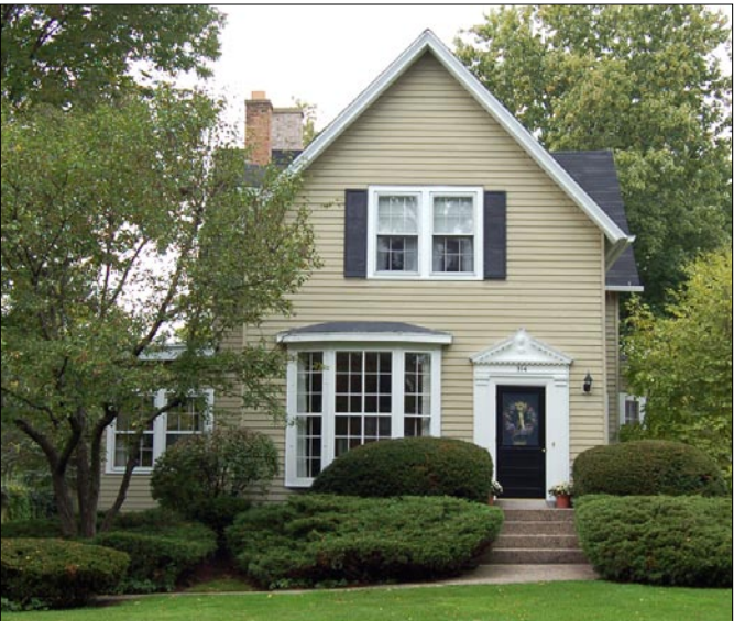
Placing a portion of the second story in the roof form limits the overall height of a home.
