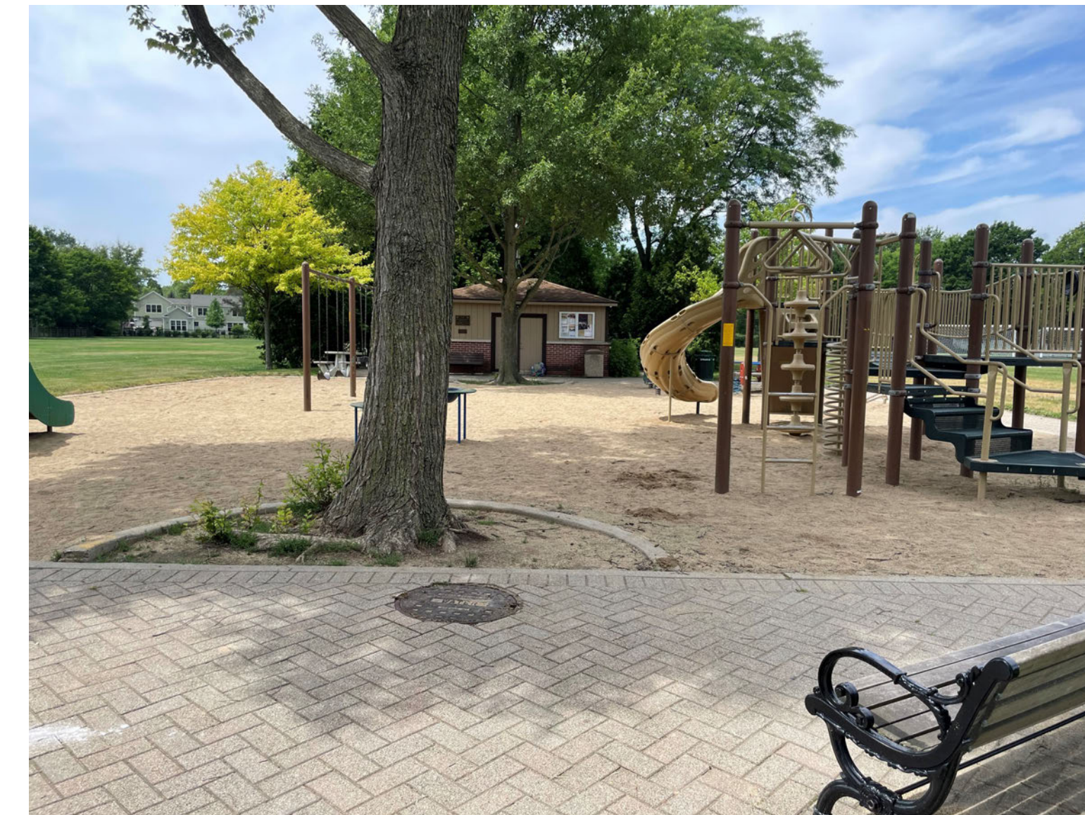
EXISTING PLAYGROUND LOOKING WEST
