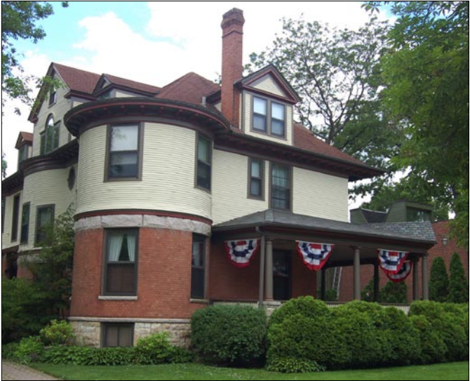
Tower is appropriate to the Queen Anne style of the home. The primary wall materials continue onto the tower, blending it into the overall composition.
