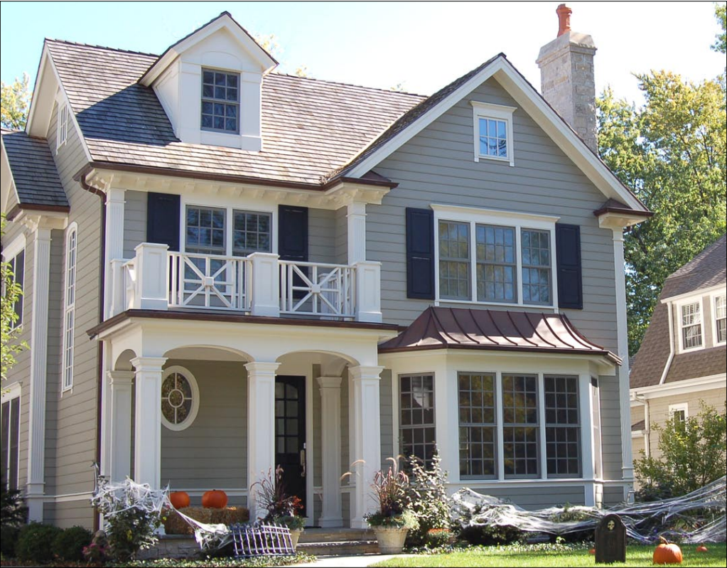
Varied roof forms, substantial detailing and massing variations convey a sense of scale characteristic of many Winnetka neighborhoods.
