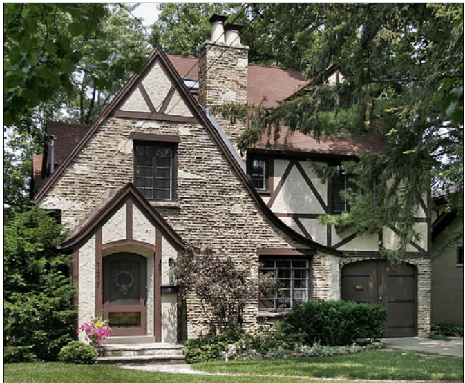
Architectural details, materials and articulated massing combine to create visual interest and convey a sense of human scale.
