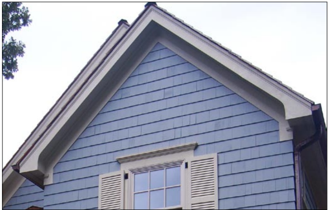
Fascia board beneath gable “supports” roof visually, and is proportional with rake board.
