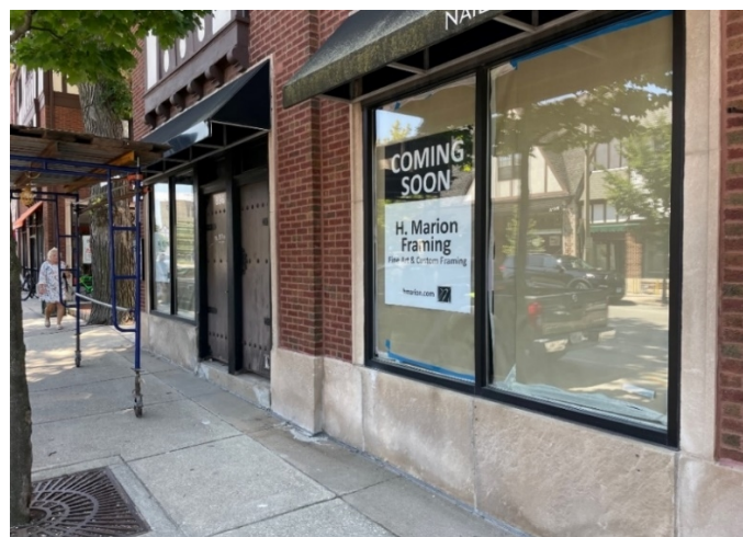
Figure 3 – Subject Property – Store frontage of east building façade along Green Bay Road
