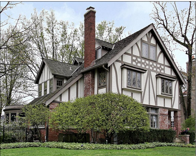
A change in materials from a brick base to stucco above, combined with the application of half-timber details, conveys a sense of human scale.
