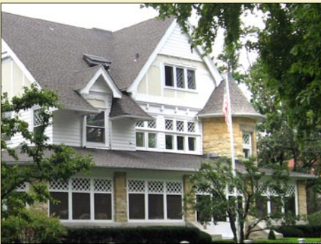
Tower is proportional and does not rise above the height of the main wall plate.
