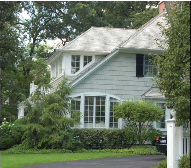
This home maintains a full second story along the side (left), but is inset from both the front and side wall of the first floor, and is visually “laid atop” the main roof line. As a result, the second floor appears lower and smaller, contributing to a reduced side wall height, and a sense of scale and detail.
