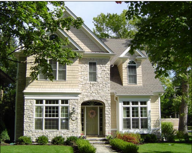
This home’s entry, materials use and detailing convey a sense of human scale.
