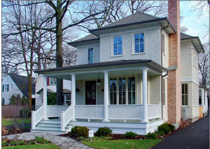
This home combines horizontal and vertical massing articulations to reduce its perceived scale. Vertically the home steps down to a one story porch, and horizontally the side wall is stepped in away from the side lot line.
