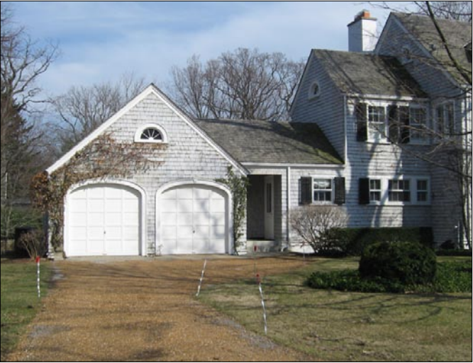
A gravel driveway permits percolation of water into the soil and reduces storm water runoff.
