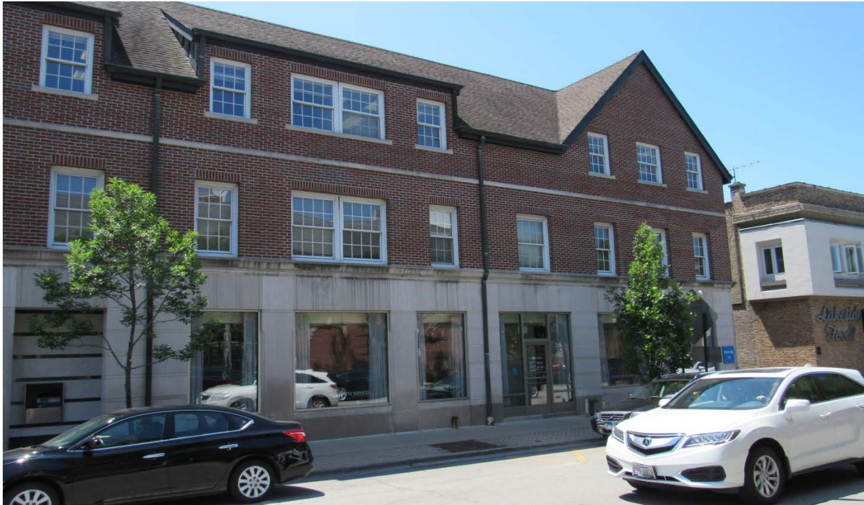
Figure 5 – Subject Property – North elevation, further west along Elm Street
