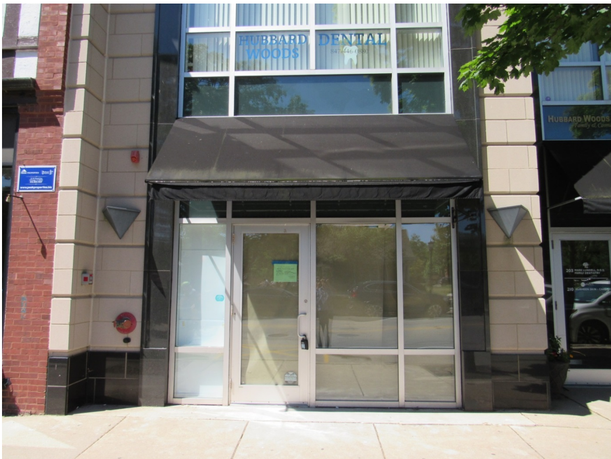
Figure 1 – Subject Property – Storefront along Green Bay Road
