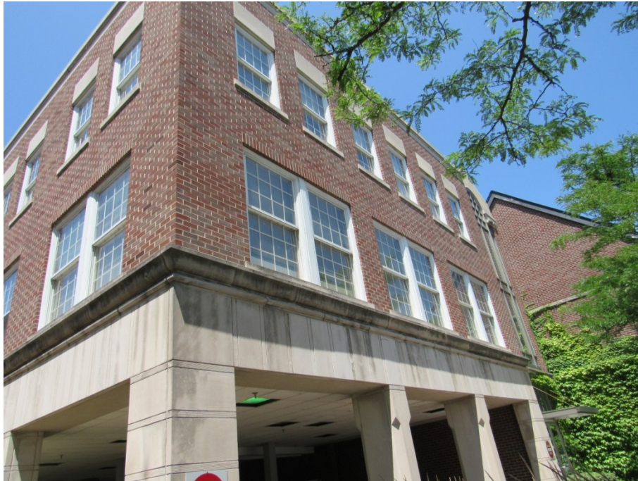
Figure 1 – Subject Property – Corner of south and east elevations
