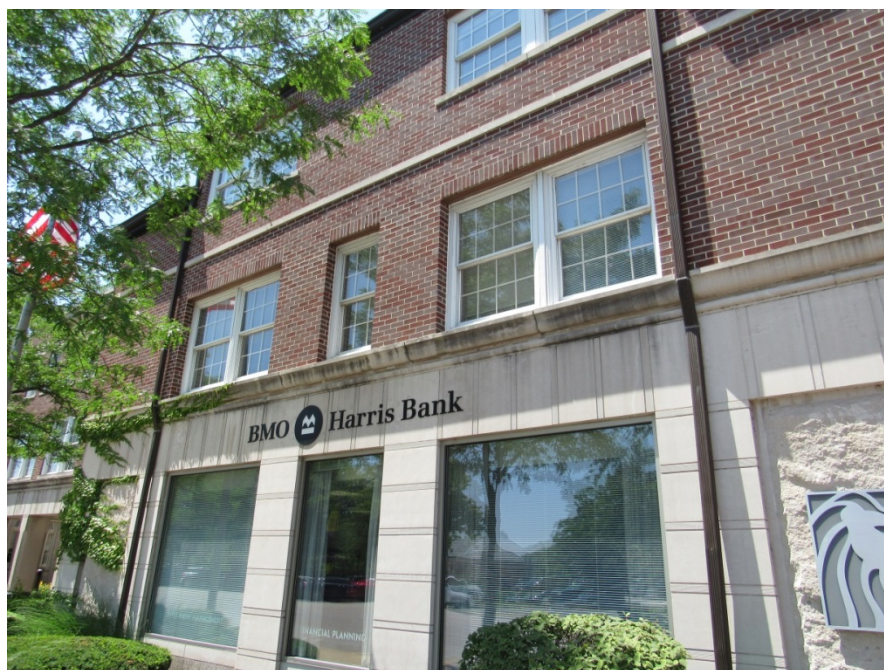
Figure 2 – Subject Property – East elevation
