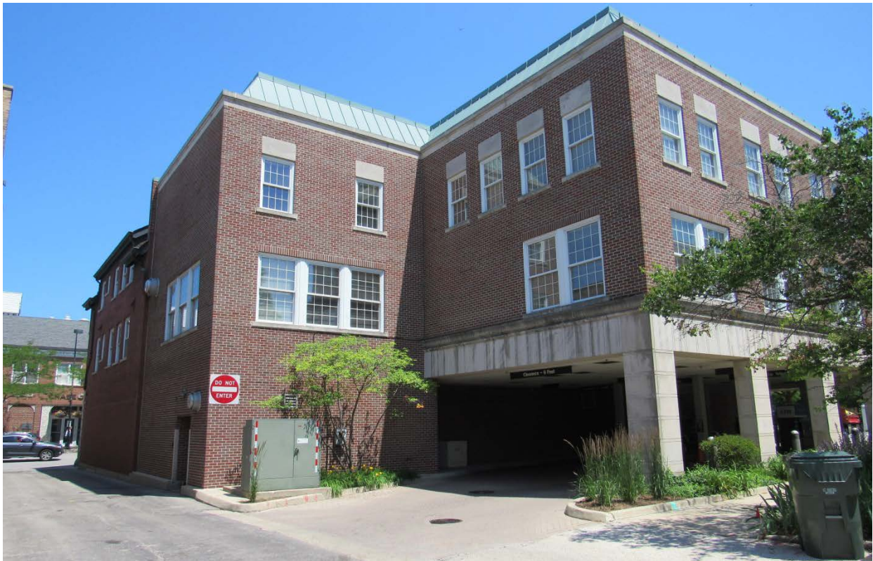
Figure 6 – Subject Property – Corner of west and south elevations
