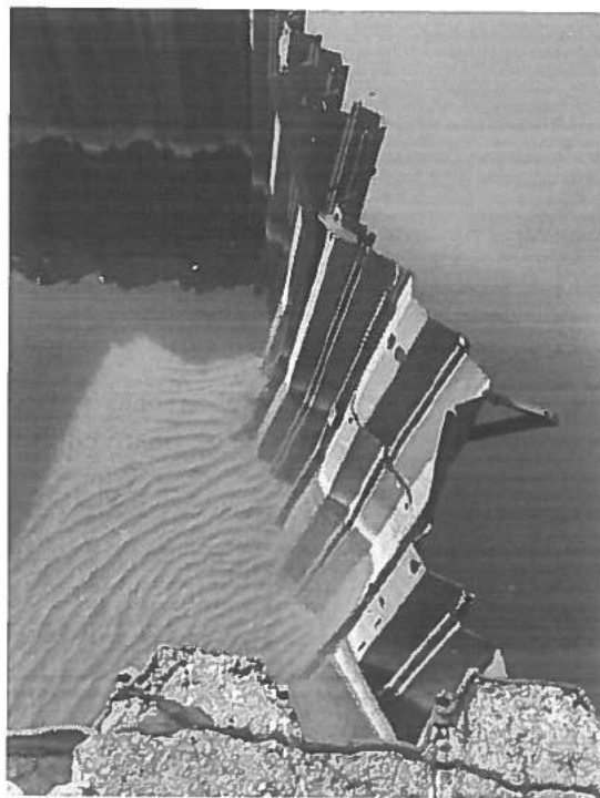
Photo – Area Between Pier And Sheet Piling
