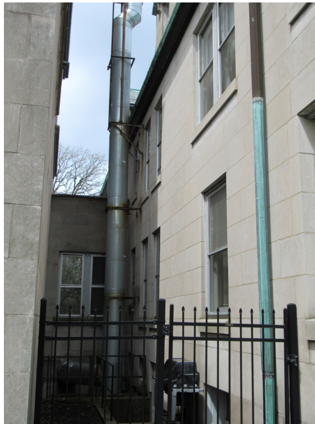
Figure 5 – South façade, near building connection to church
