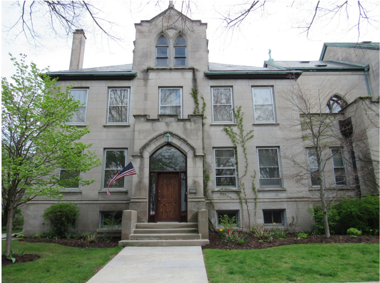
Figure 1 – West façade along Burr Avenue
