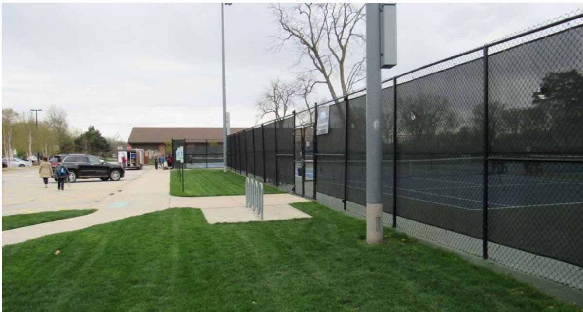
Figure 2 – Tennis courts with existing windscreens (southern part of the campus)
