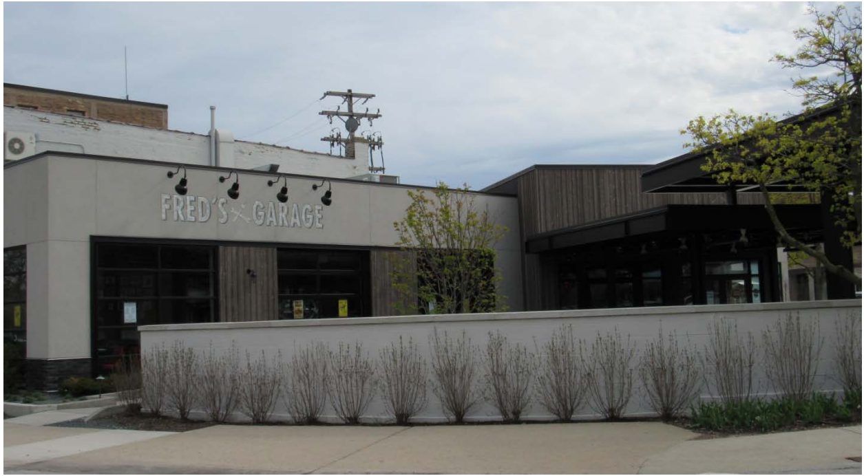
Figure 3 – Northeast façade, site of proposed wall sign change
