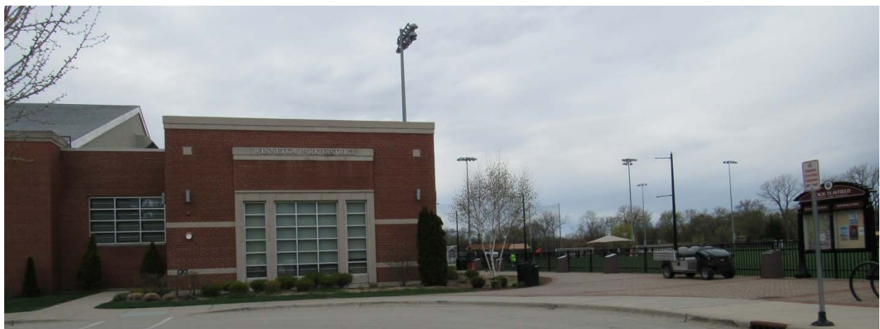
Figure 5 – Northeast corner of Park District building near sports fields, from parking lot along Hibbard Road
