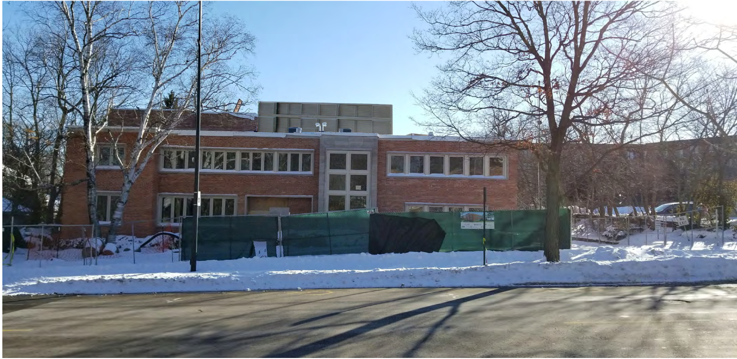
VIEW OF FRONT ELEVATION, FROM ELM ST
