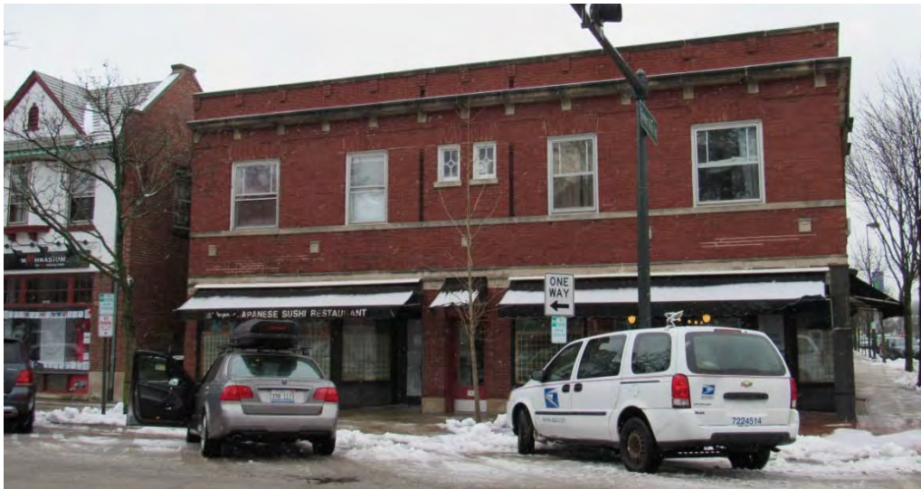
Figure 1 – North façade along Gage Street
