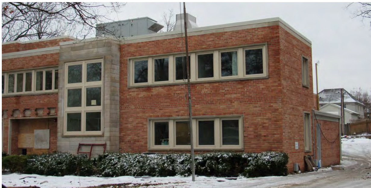
Figure 1 – Northwest view of building.
