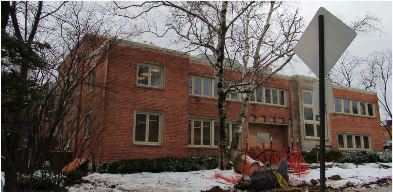
Figure 2 – Northeast view of building.
