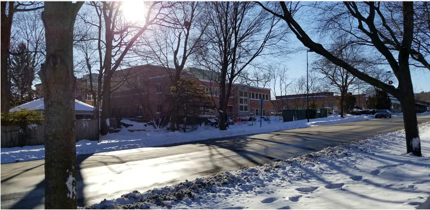
VIEW OF FRONT ELEVATION, FROM ELM ST
