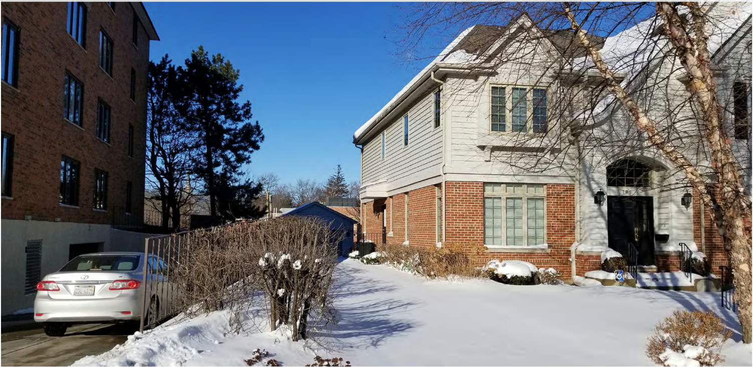
VIEW OF SOUTH ELEVATION, FROM OAK ST
