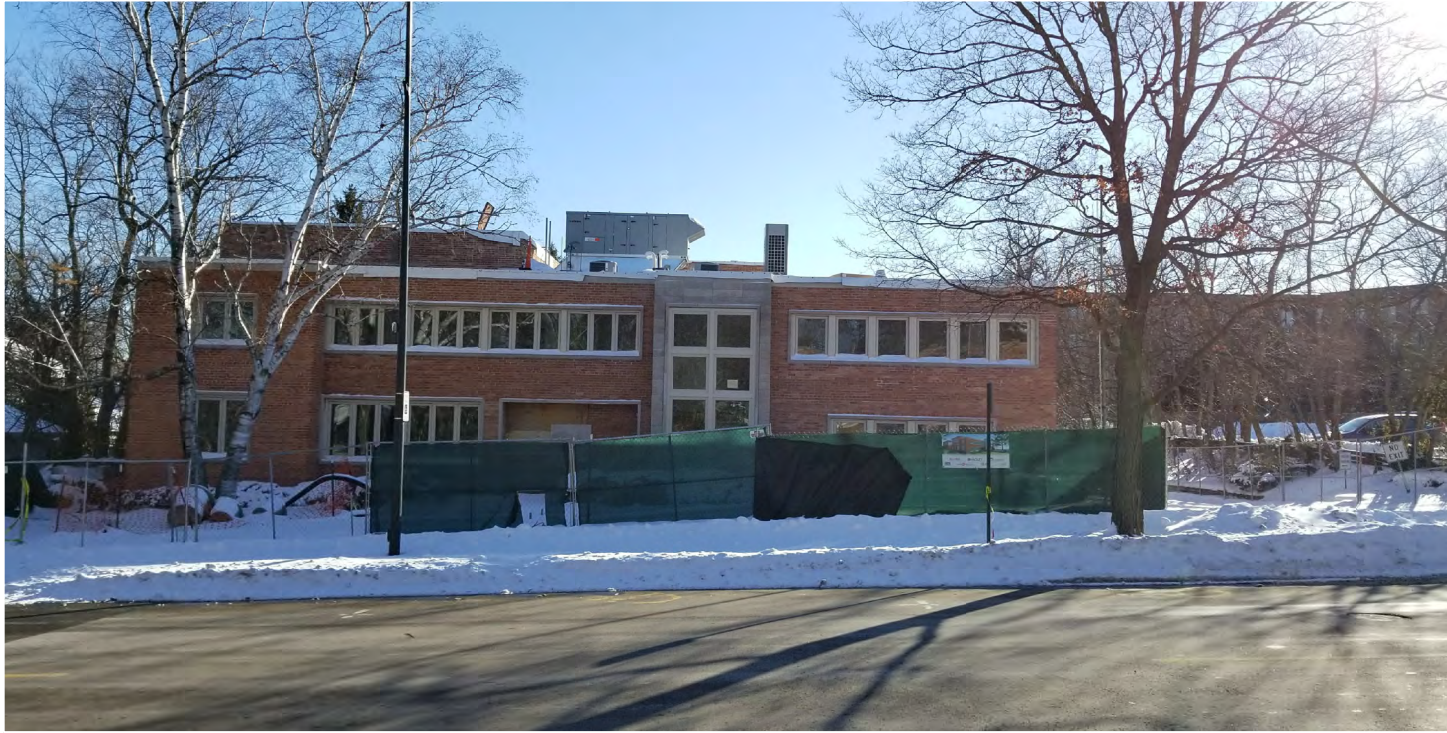
VIEW OF FRONT ELEVATION, FROM ELM ST
