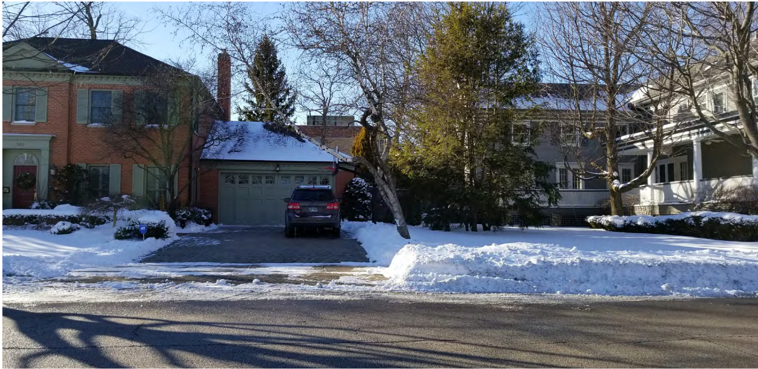
VIEW OF EAST ELEVATION, FROM MAPLE ST
