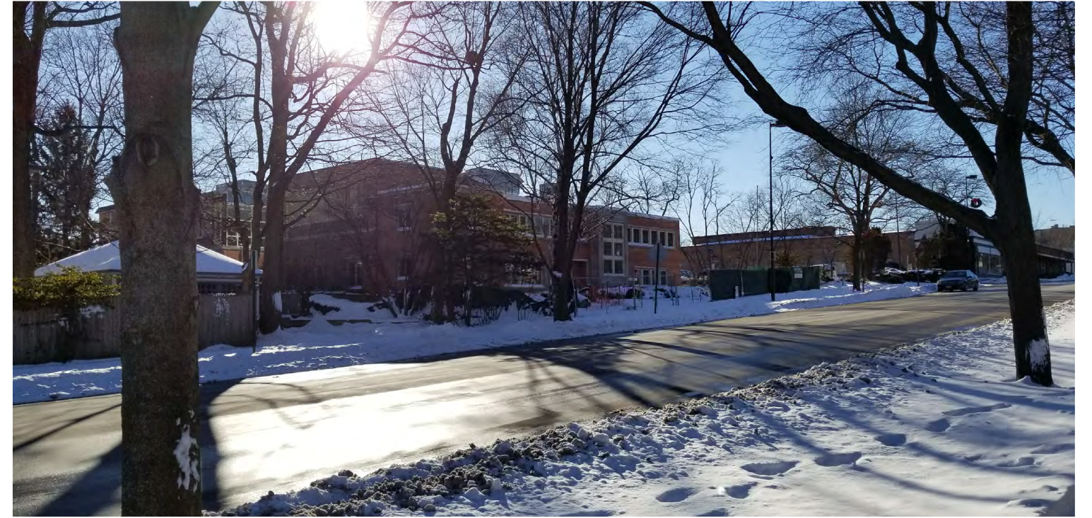
VIEW OF FRONT ELEVATION, FROM ELM ST
