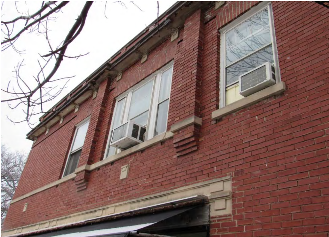
Figure 4 – West façade, second story windows
