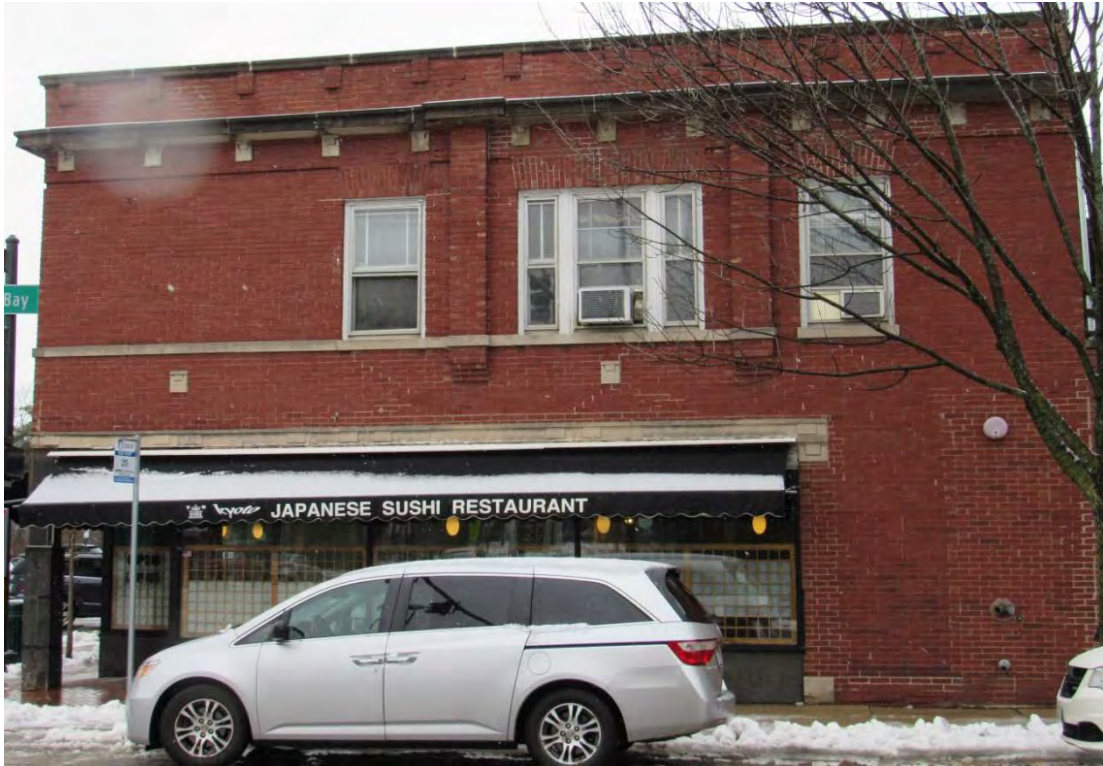
Figure 3 – West façade, along Green Bay Road
