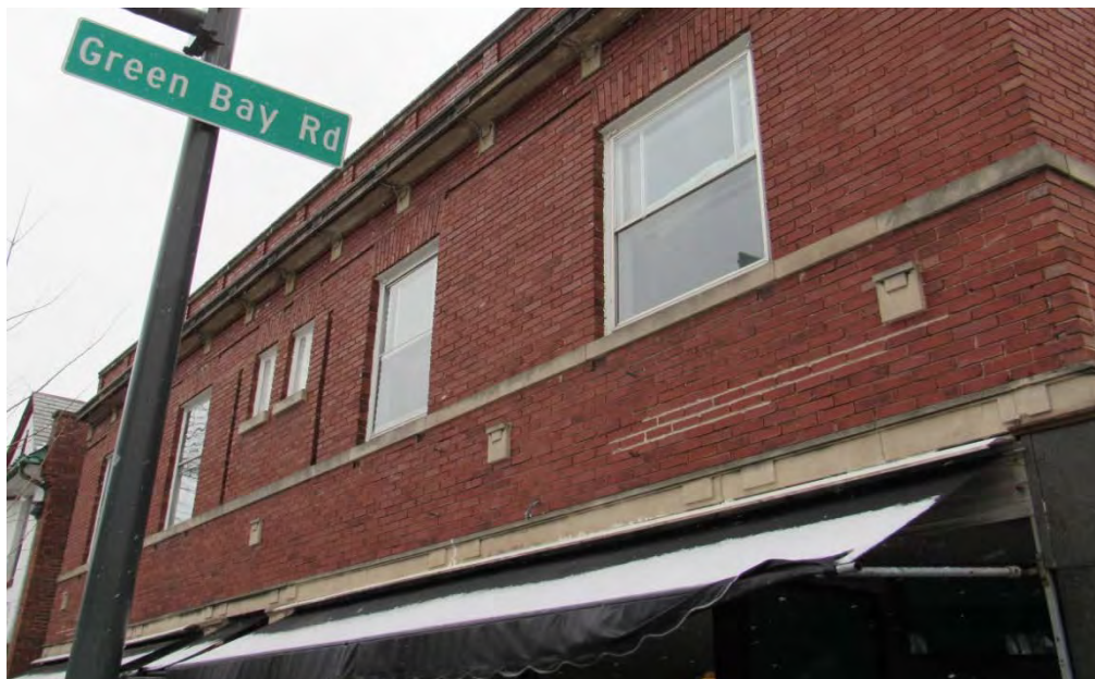
Figure 2 – North façade, second story windows
