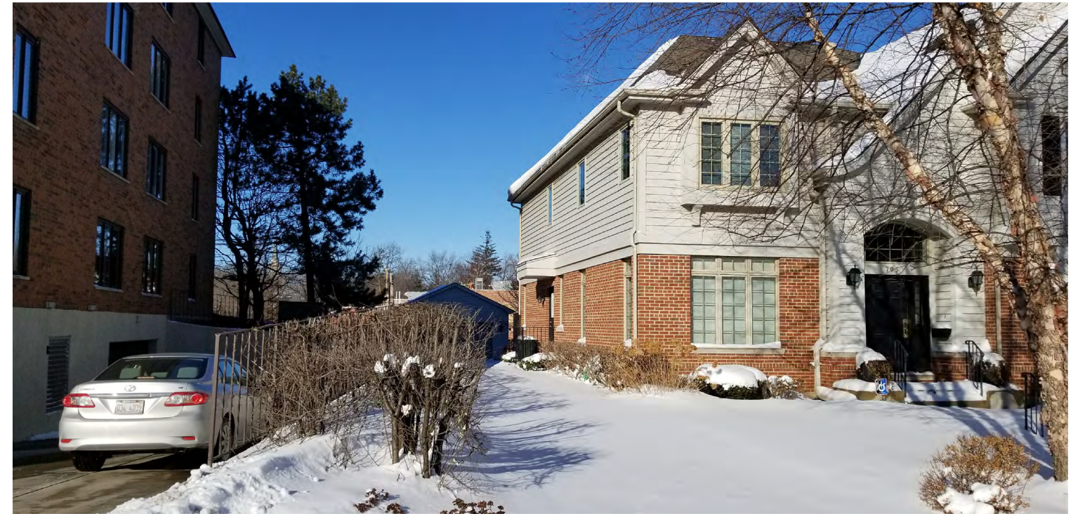
VIEW OF SOUTH ELEVATION, FROM OAK ST
