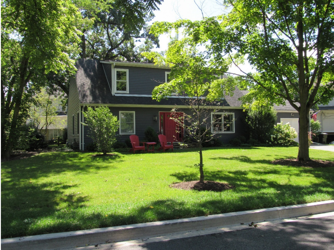
Figure 3 – Subject Property (Easterly Front Elevation – Gage Street)
