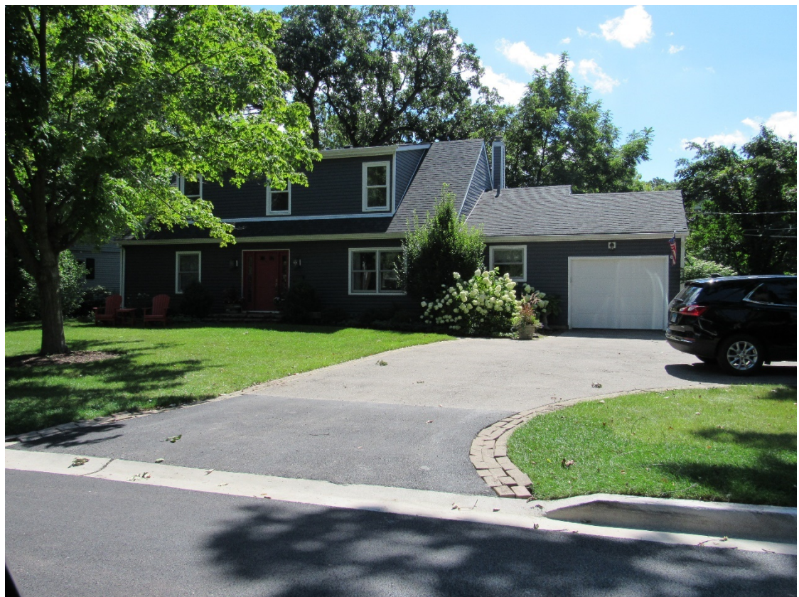
Figure 4 – Subject Property (Westerly Front Elevation – Gage Street)
