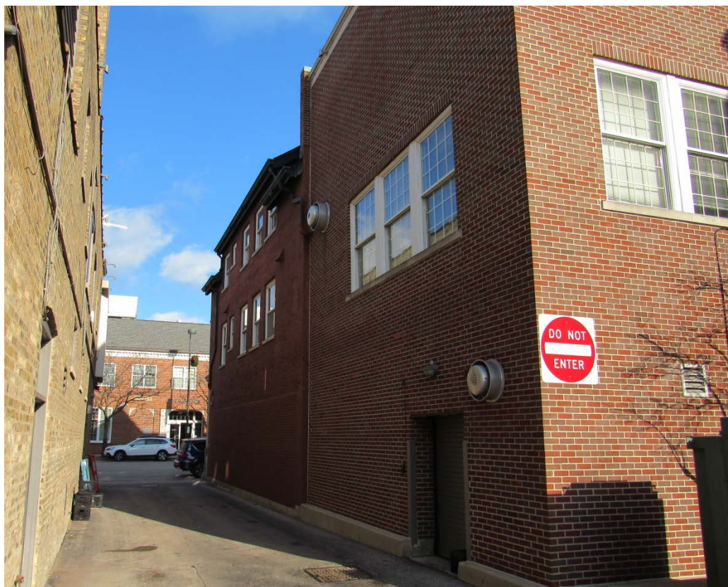
Figure 4 – Subject Property – West elevation, along alley
