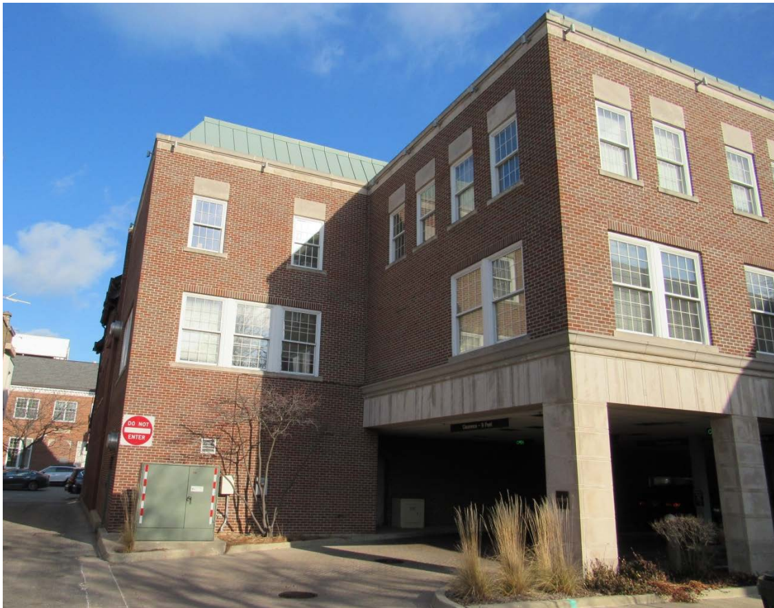
Figure 5 – Subject Property – Corner of west and south elevations
