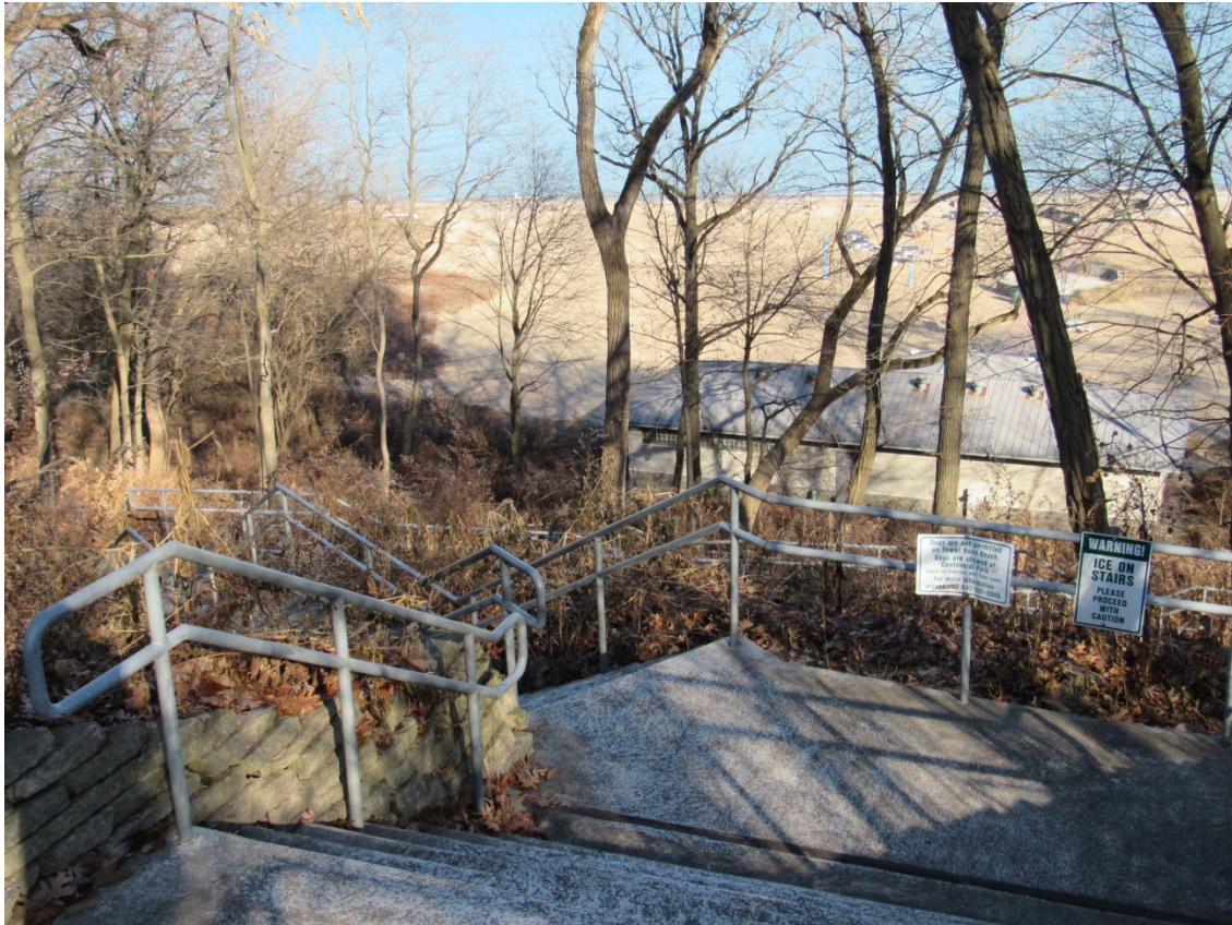
Figure 3 – Existing stairs to beach
