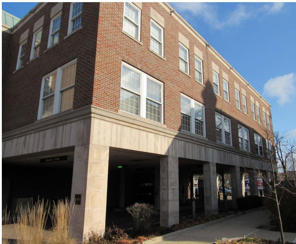
Figure 6 – Subject Property – South elevation facing Village Hall
