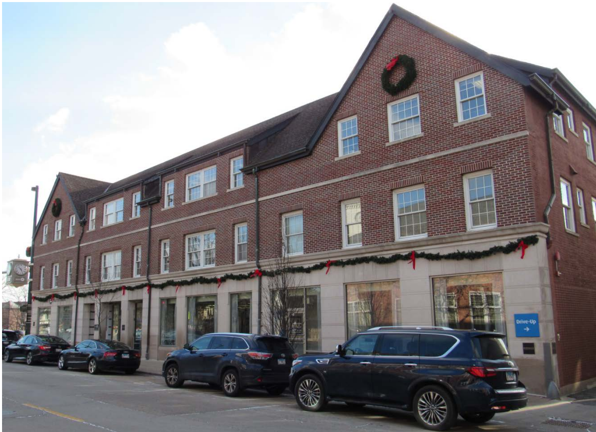
Figure 3 – Subject Property – North elevation, along Elm Street
