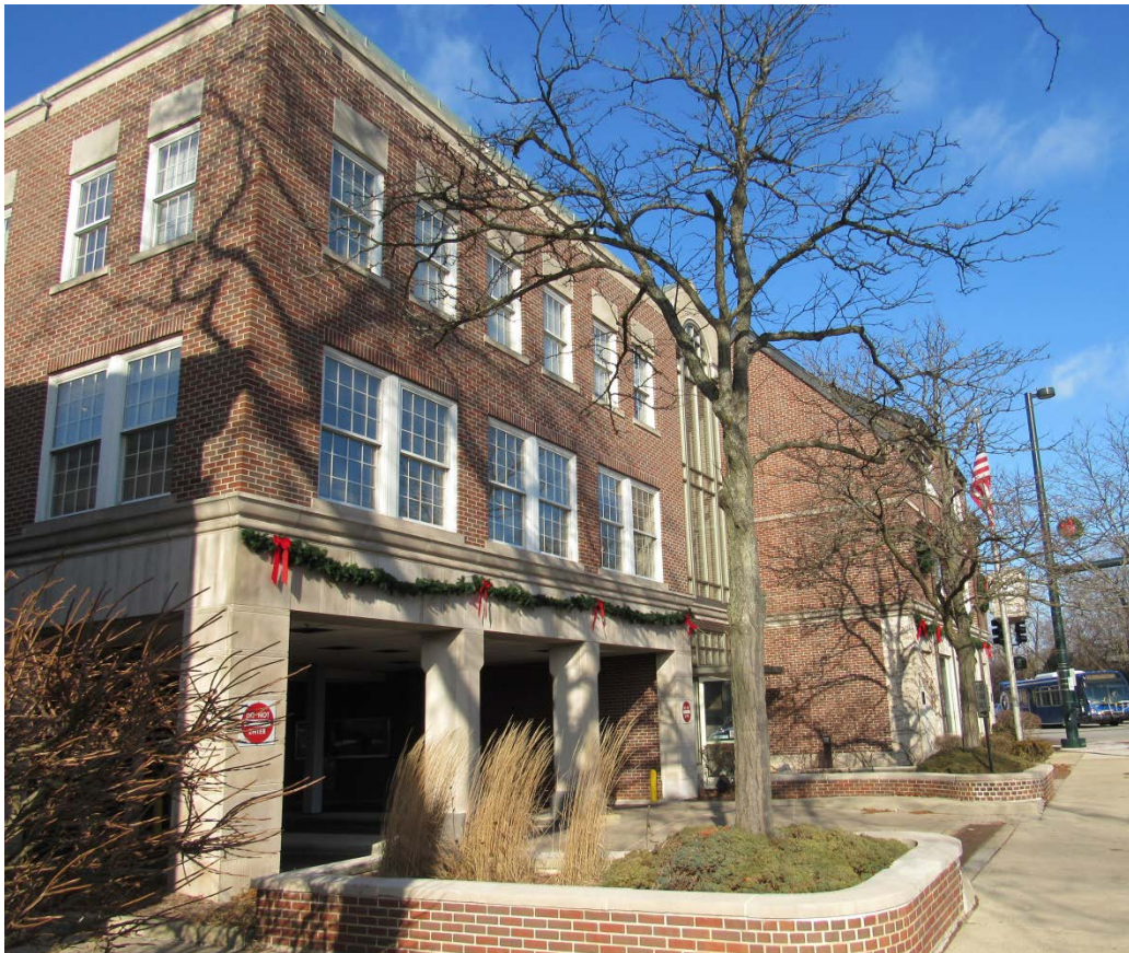
Figure 1 – Subject Property – Corner of south and east elevations
