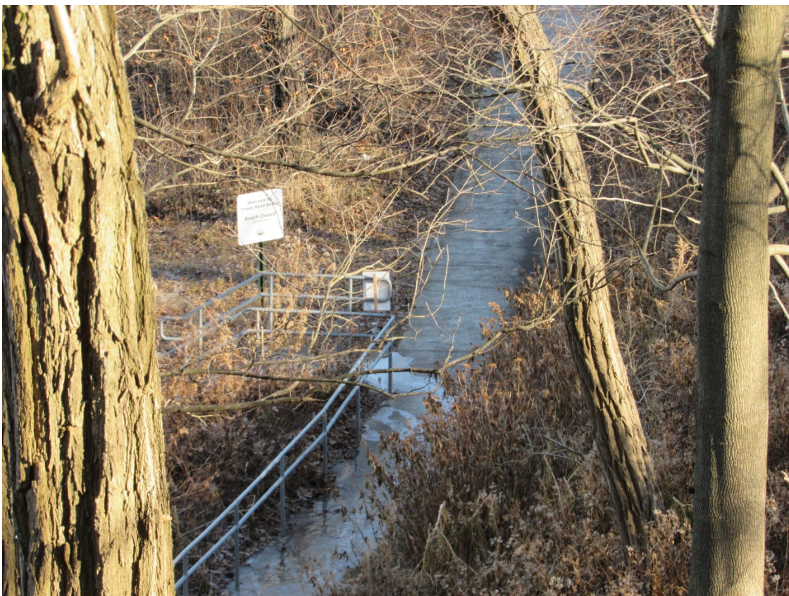
Figure 4 – General location of seepage at base of bluff where dry creek and boardwalk are proposed
