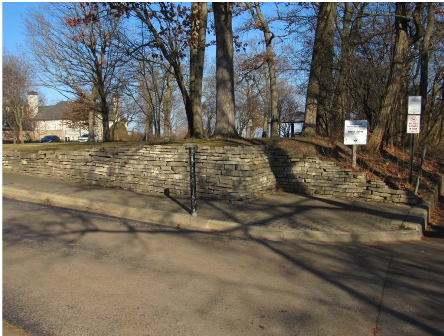
Figure 2 – Entrance to Subject Property
