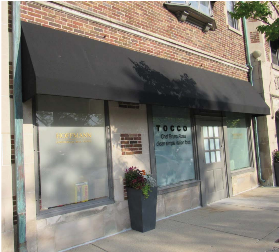
Figure 3 – Subject Property – Window and awning along western frontage of Chestnut Street
