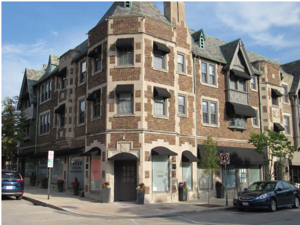
Figure 4 – Subject Property – Southeast corner of Chestnut Court and Chestnut Street
