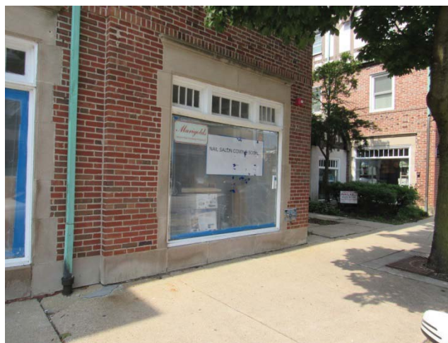
Figure 1 – Subject Property – Main window along street frontage on Green Bay Road
