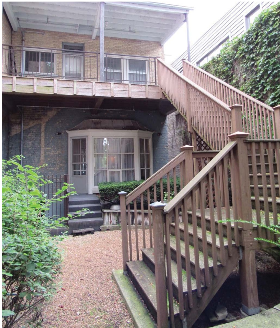
Figure 3 – Subject Property – Rear deck, stairway, and window trim as visible from Chestnut Court.
