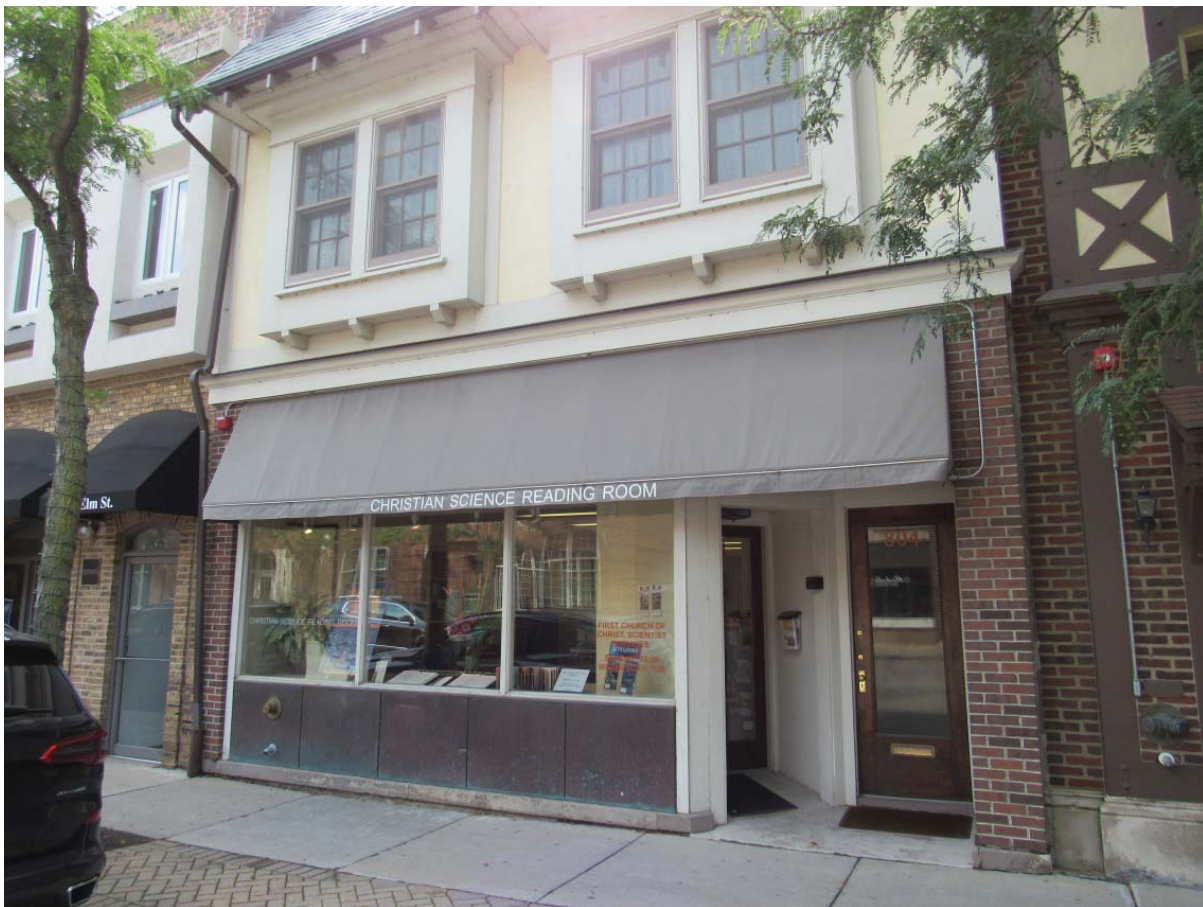
Figure 1 – Subject Property – Street façade along Elm Street
