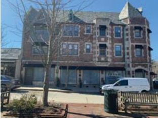
OVERALL EXISTING FACADE
