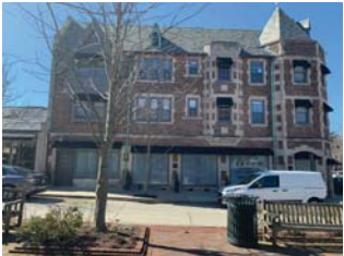
OVERALL FACADE: NEW WINDOW
