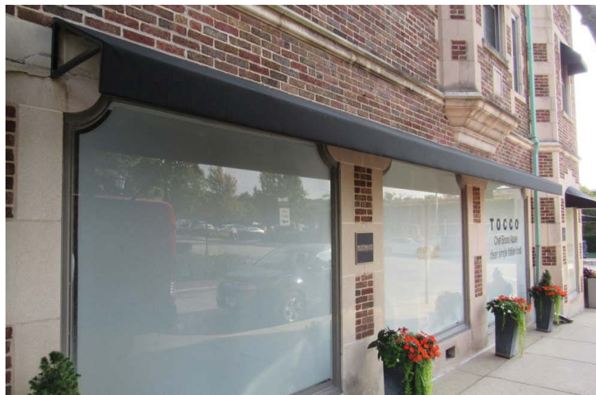
Figure 2 – Subject Property – Other awning and window along north street frontage of Chestnut Court
