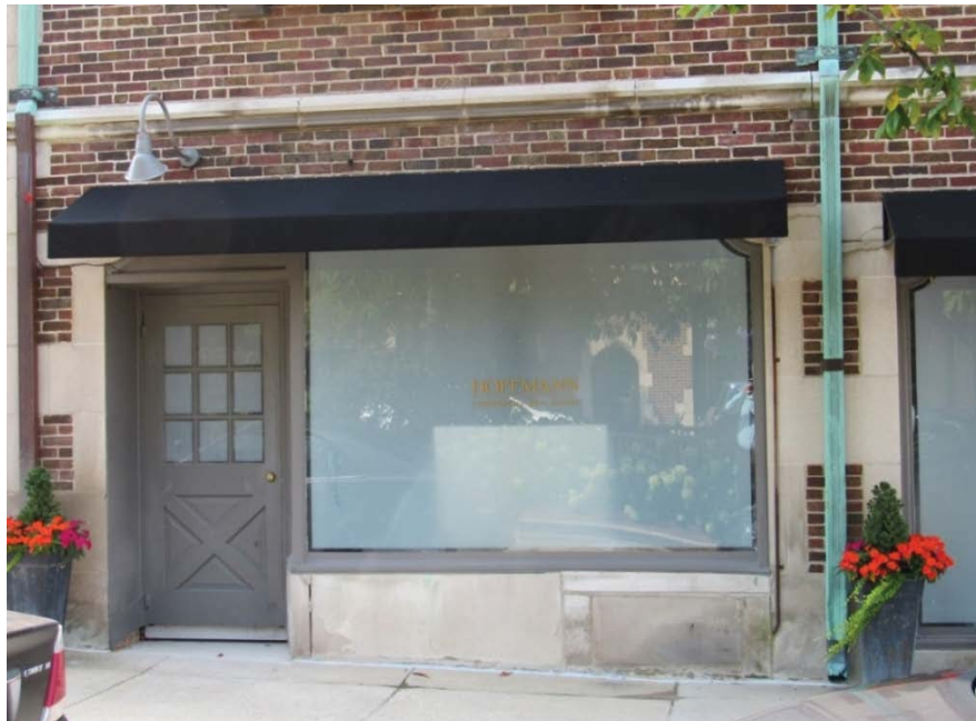
Figure 1 – Subject Property – North and easternmost window and awning along Chestnut Court
