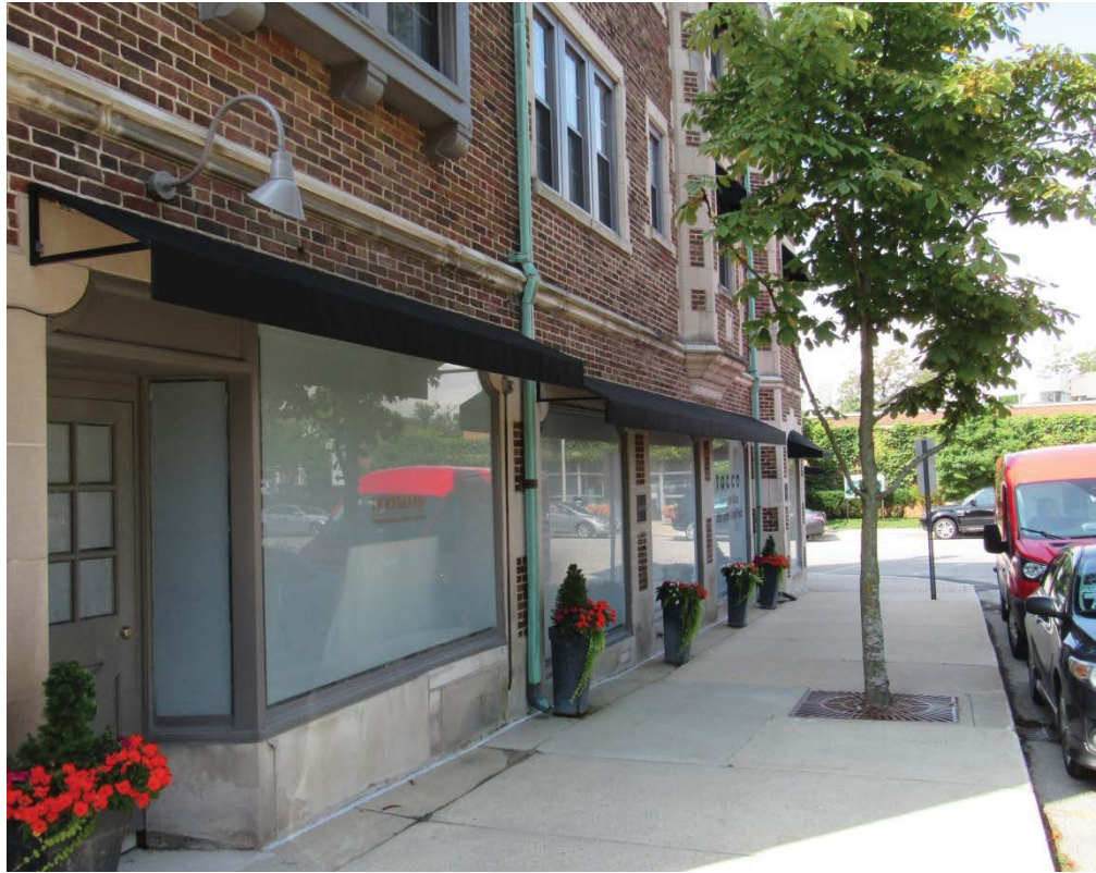
Figure 2 – Subject Property - windows along north street frontage facing west
