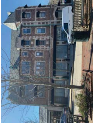
OVERALL FACADE: NEW WINDOW
