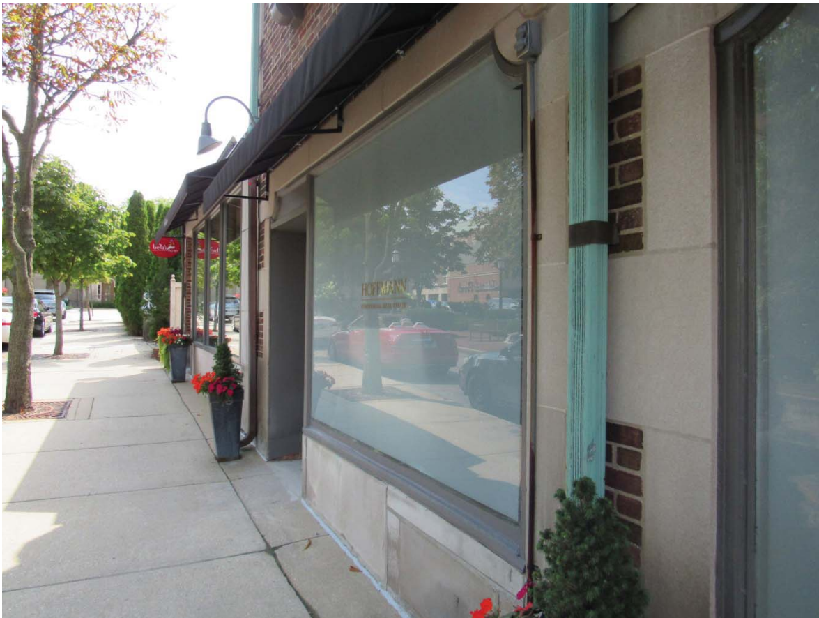
Figure 3 – Subject Property - window to be replaced facing east
