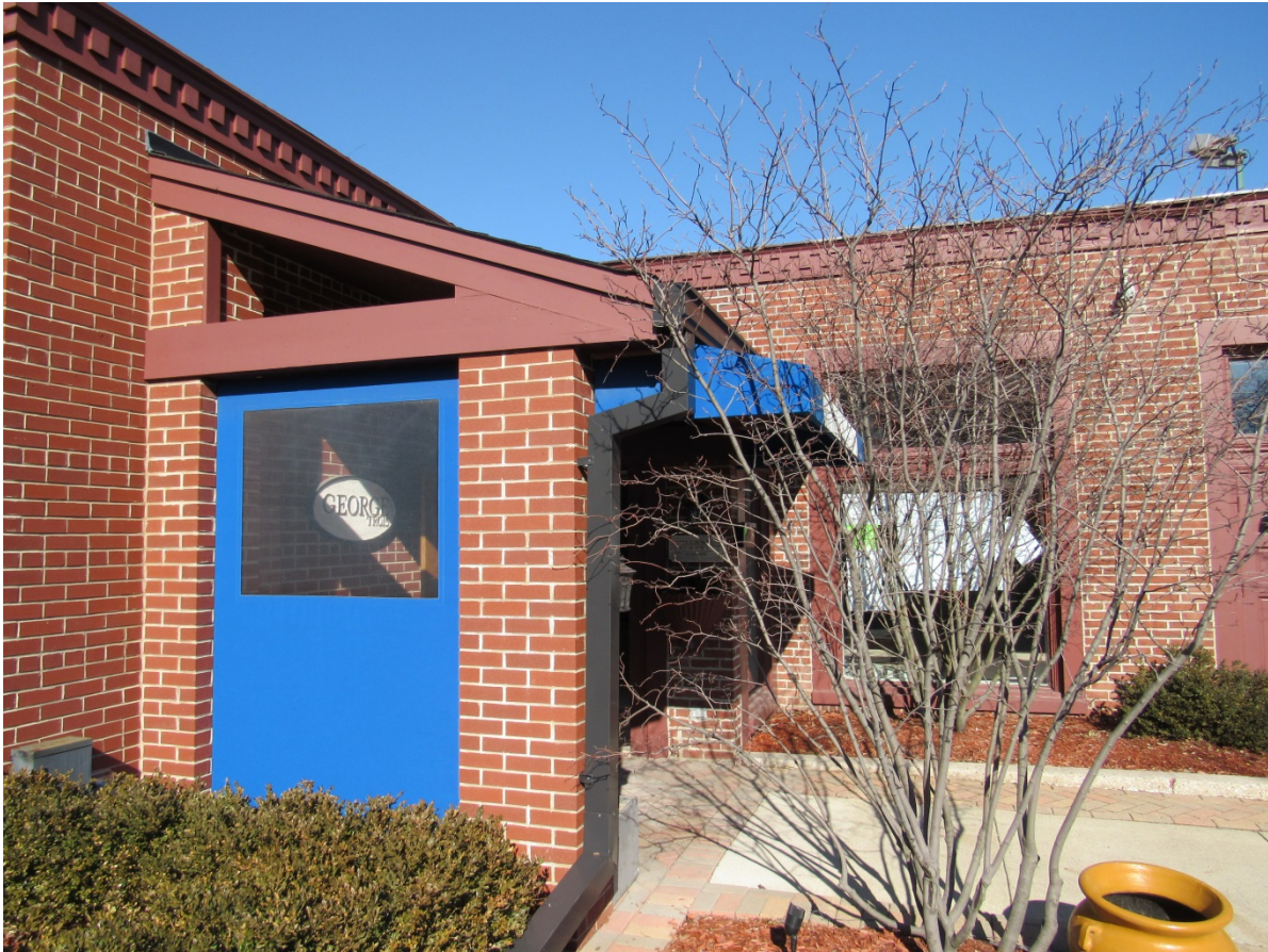
Figure 1 – Existing main entrance with roof cover awning and canvas enclosure.
