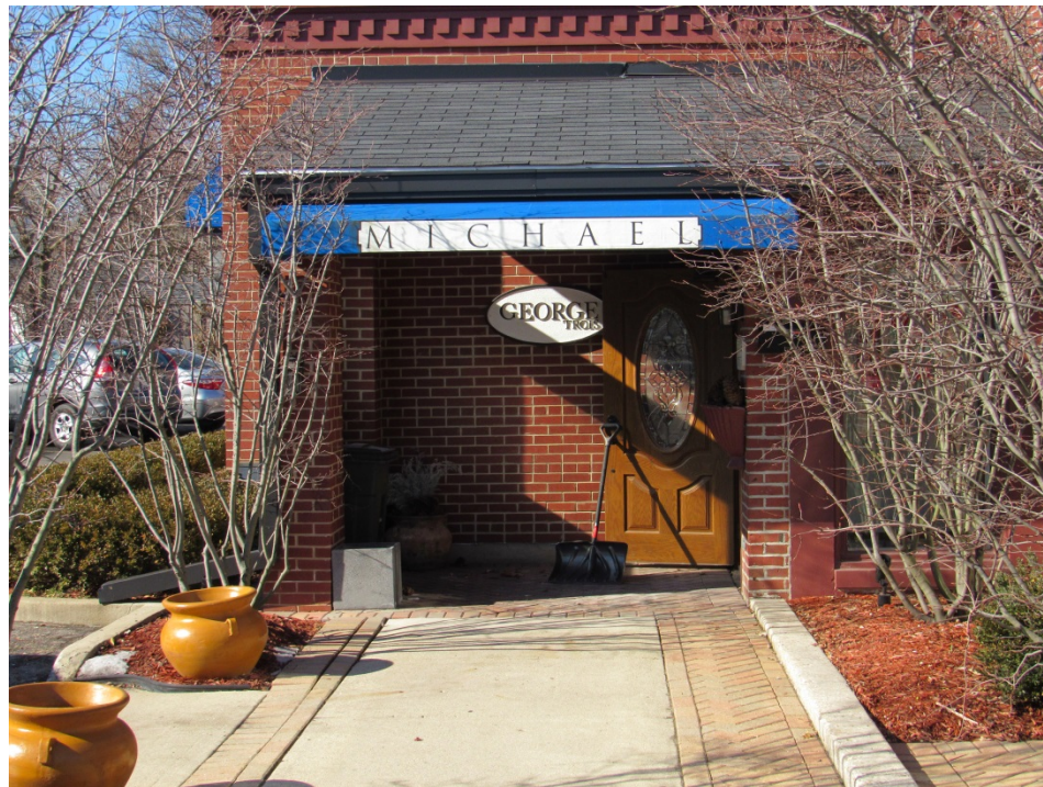
Figure 2 – Existing main entrance with roof awning and canvas enclosure.
