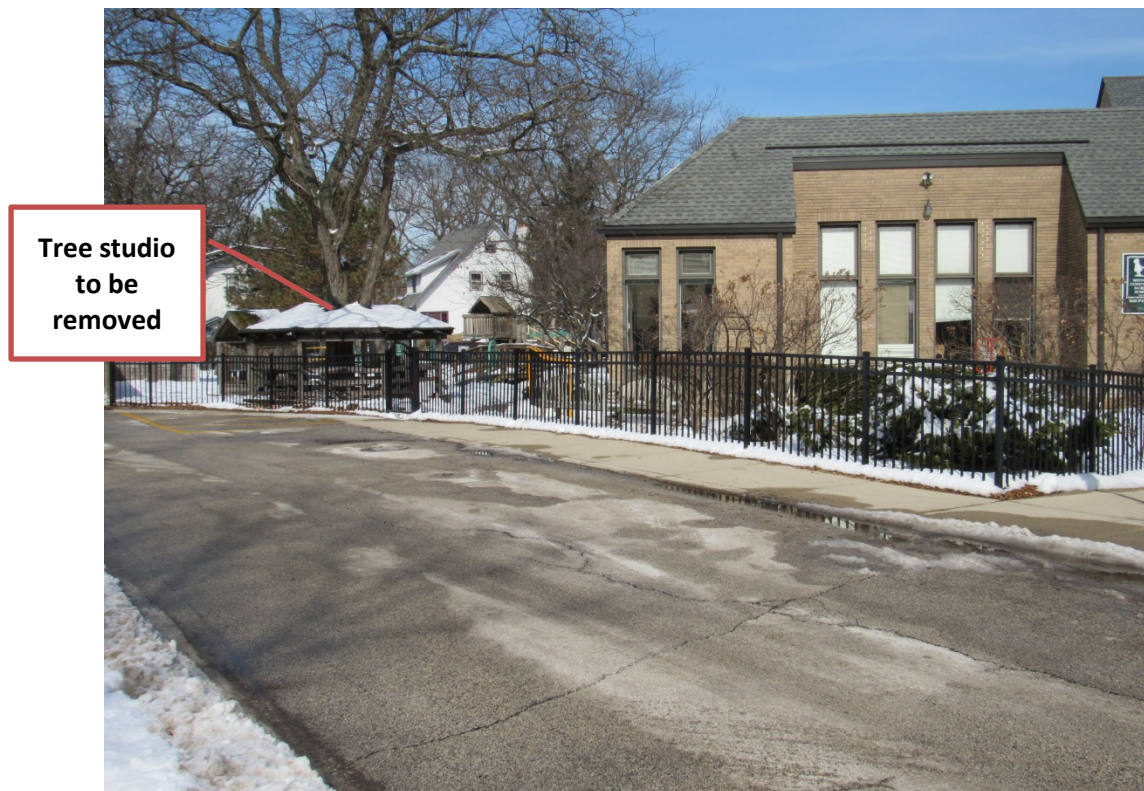
Figure 2 – Subject Property (Killian Court)
