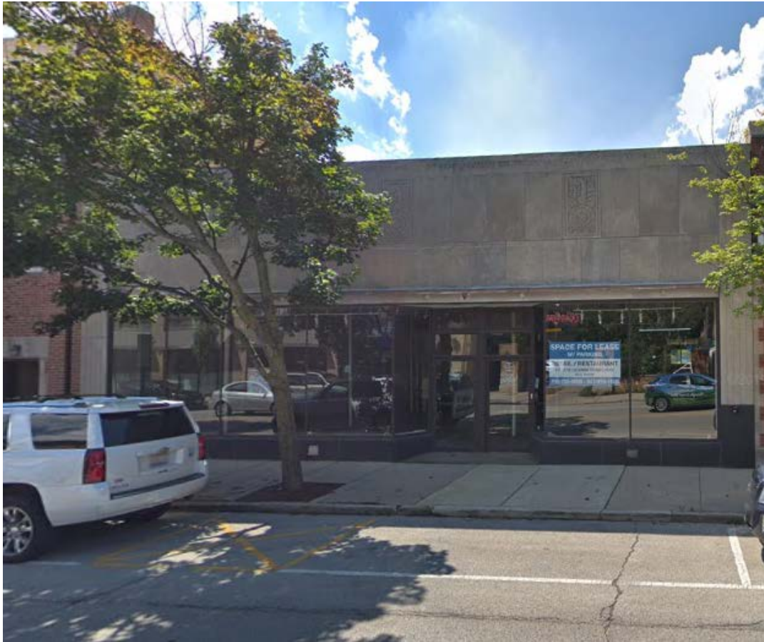
Figure 1 – East façade along Green Bay Road
