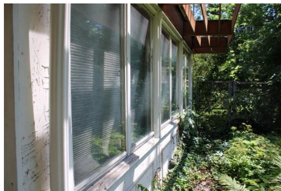
South façade of sunporch.
