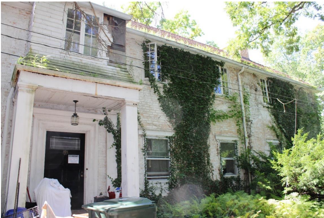
Front façade showing main entrance, looking southwest.
