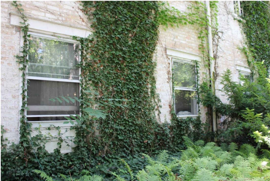
First floor windows on front façade, looking southwest.
