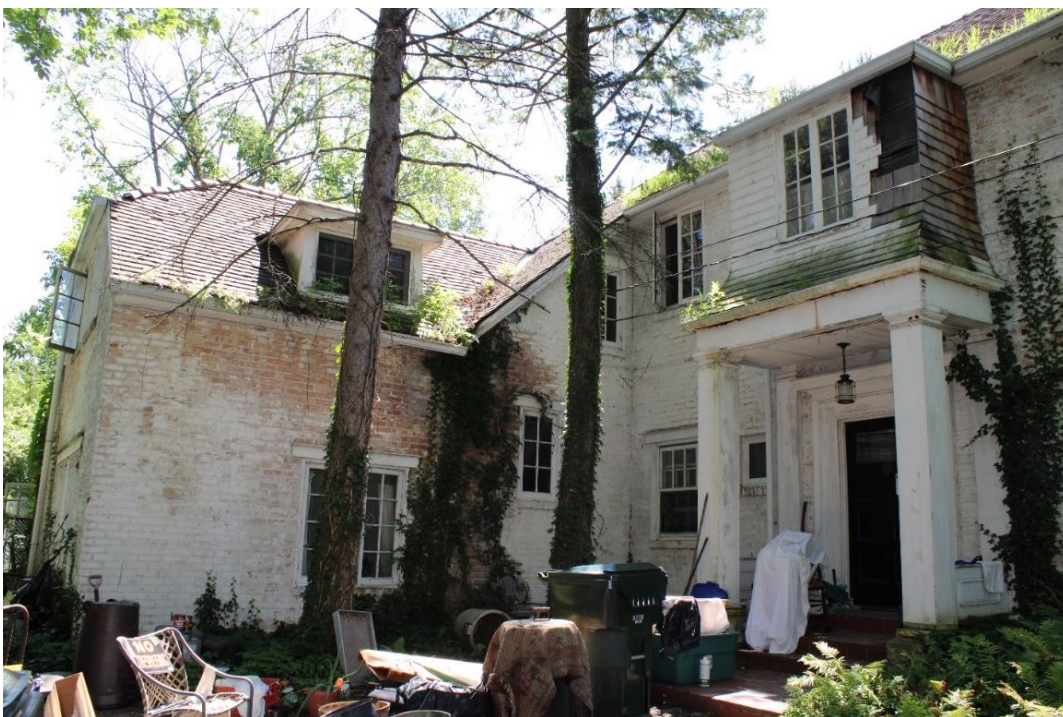
Front façade, looking southeast.
