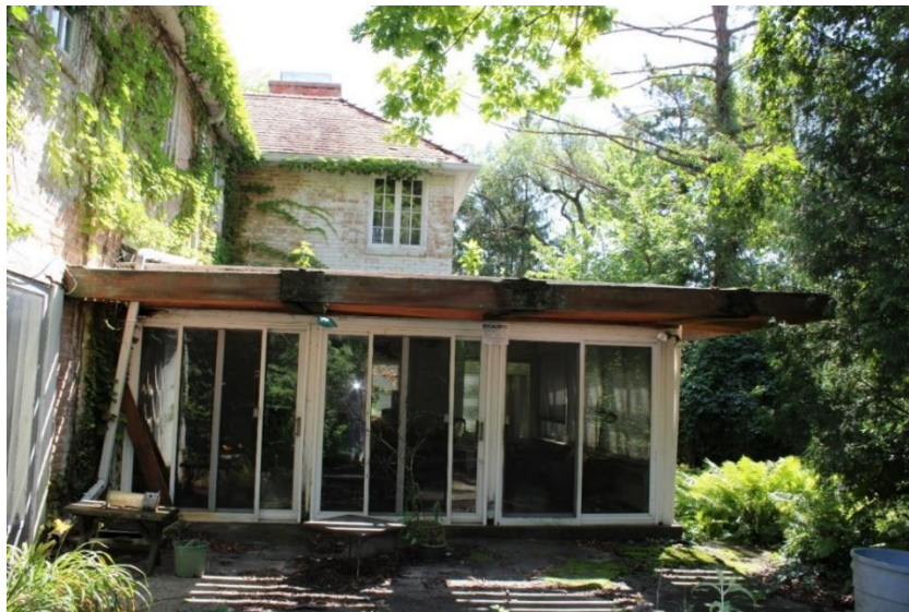
View of rear sunporch, looking east.
