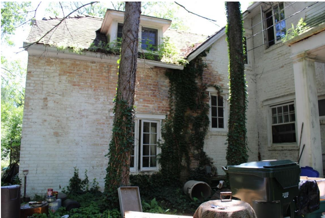
West façade of north wing.
