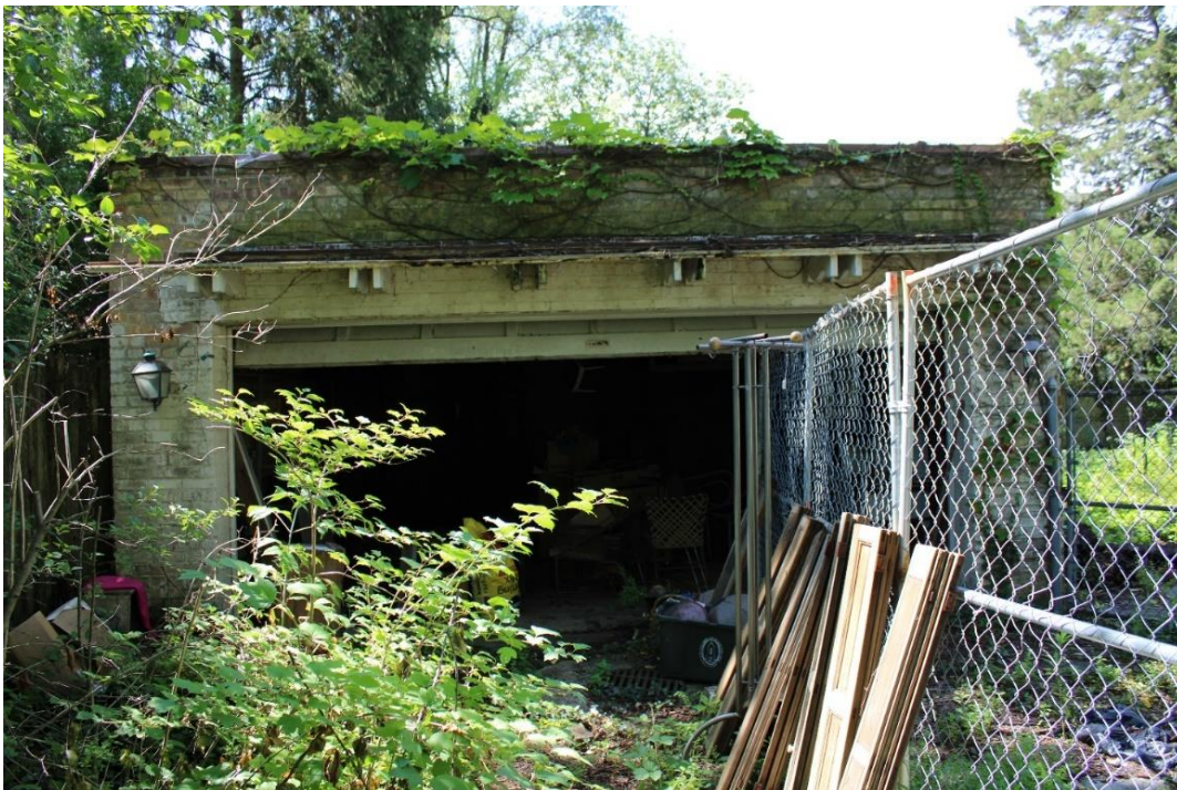
Detached brick garage, looking south.
