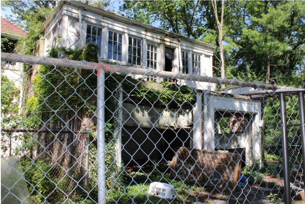
North wing, looking northwest, showing sleeping porch and attached garage.
