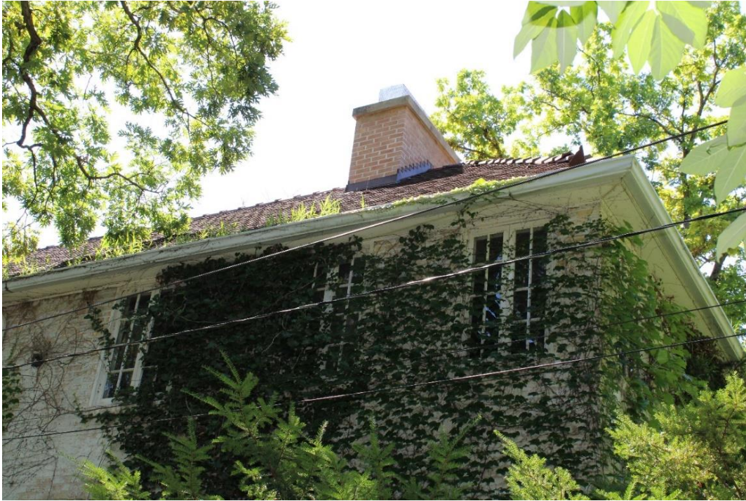
Detail of front façade's second floor.
