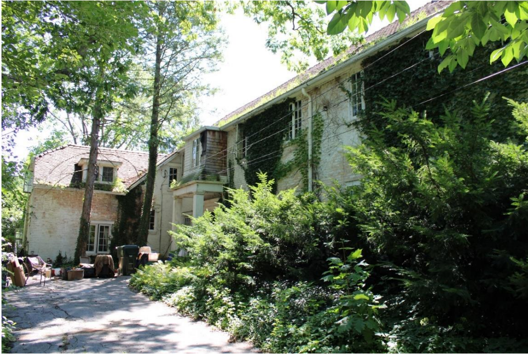
Front façade, looking east.
