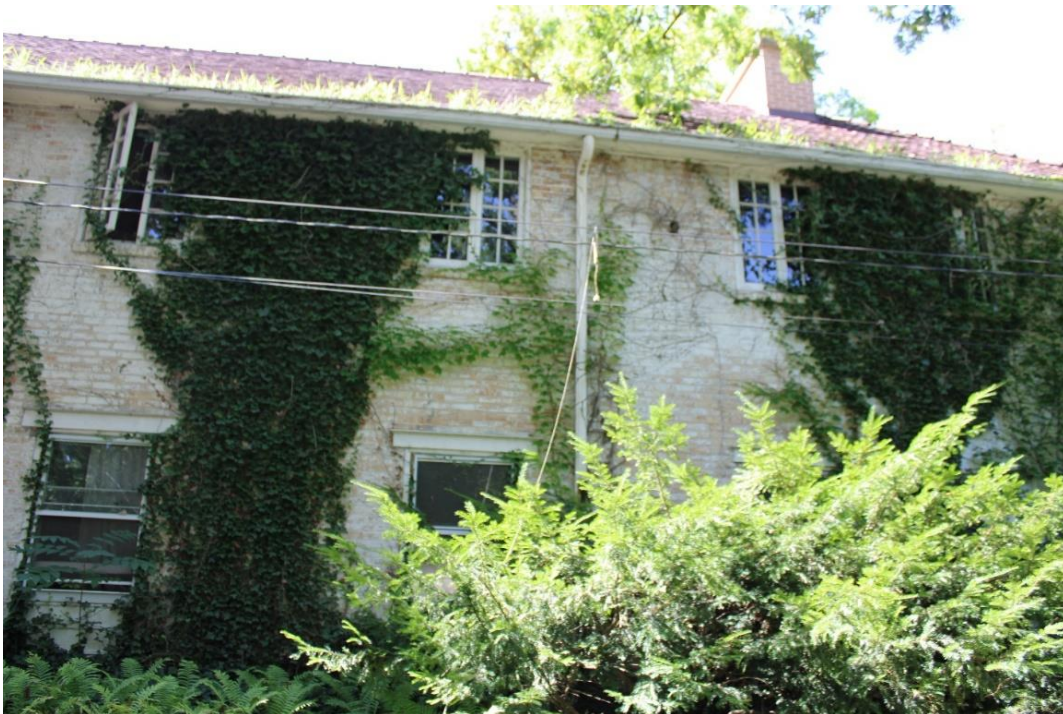
Front façade, looking south.
