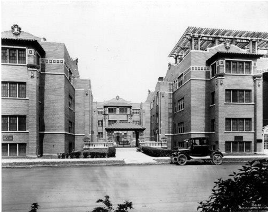
Kellshore Hotel (now apartments) at 713-756 W. Irving Park Road in Chicago.
