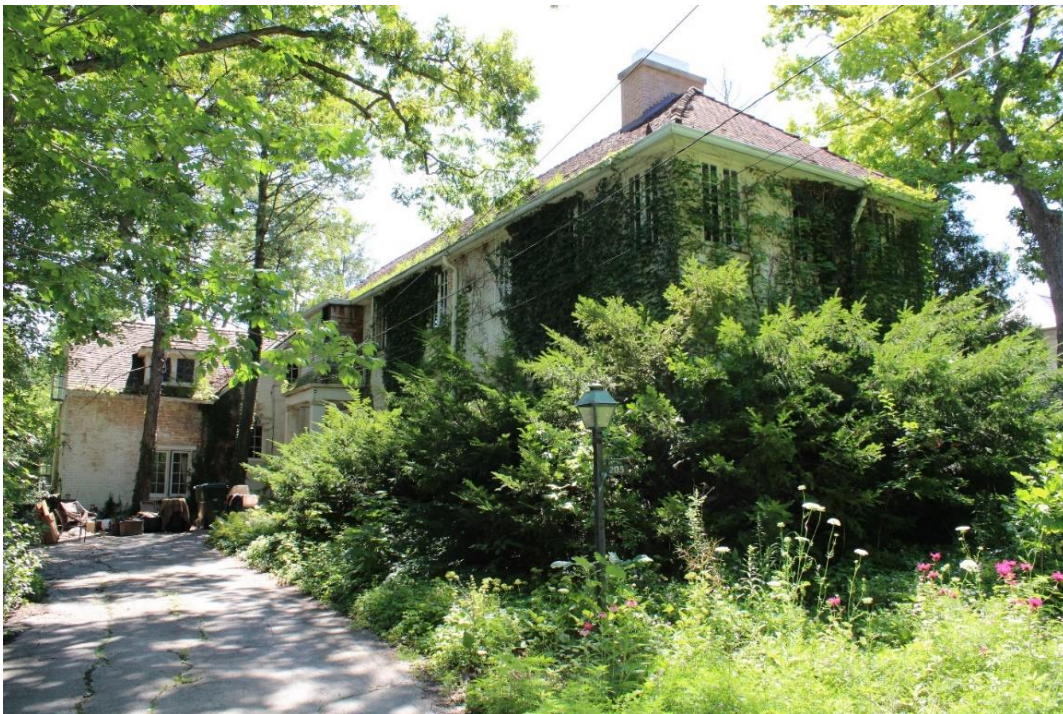
View of front of the house, looking southeast.
