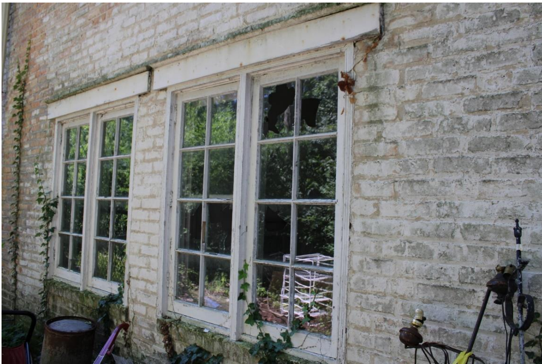
Windows on first floor of north wing, looking southeast.
