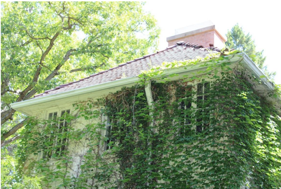
View of paired, casement windows, looking northeast.
