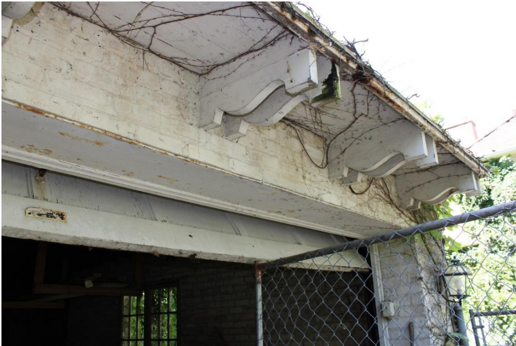
Detail of scrolled wood brackets beneath eaves of detached brick garage.
