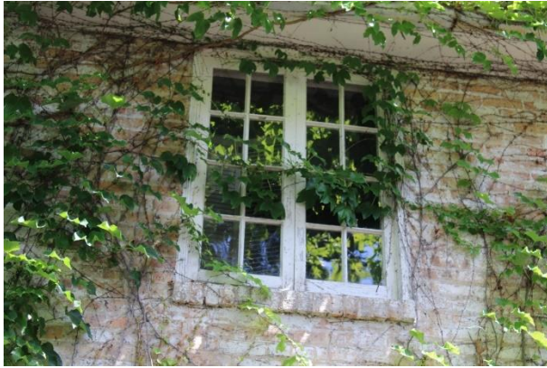
Second floor window.
