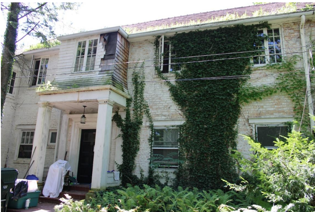
Front façade, looking southeast.
