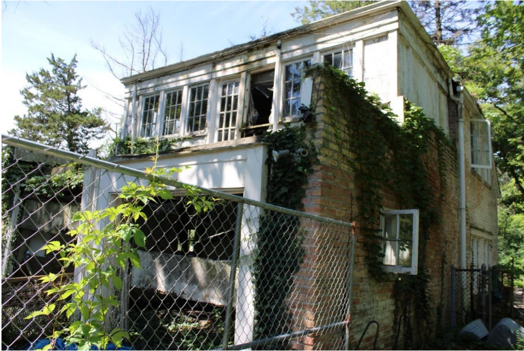
North wing, looking southwest, showing sleeping porch and attached garage.
