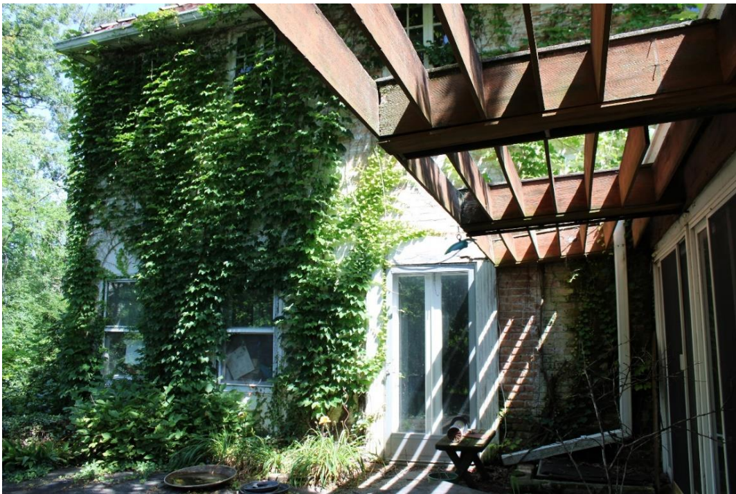
South side of the main block, view north.
