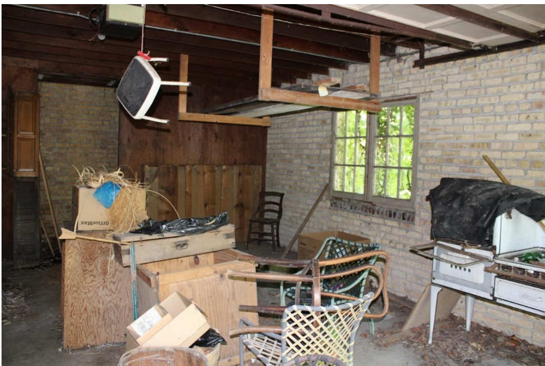
Interior of detached brick garage.
