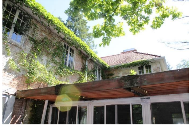
View of rear portion of house.
