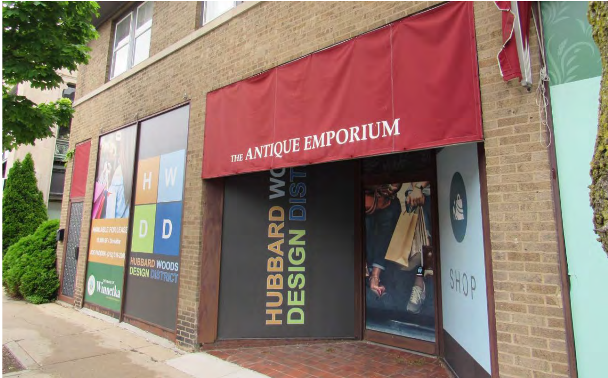
Figure 3 – Existing main entrance
