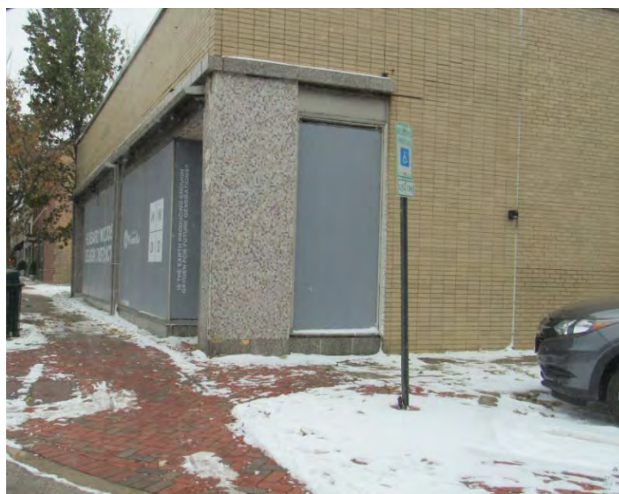
Figure 3 – Close-up of corner doorway, existing brick façade, and masonry accents (November 2019)
