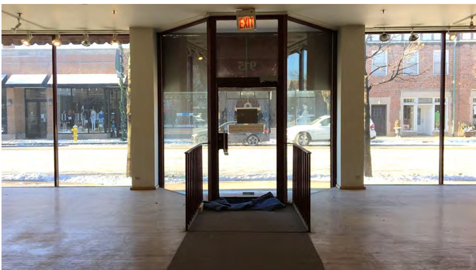
Existing Interior Storefront
