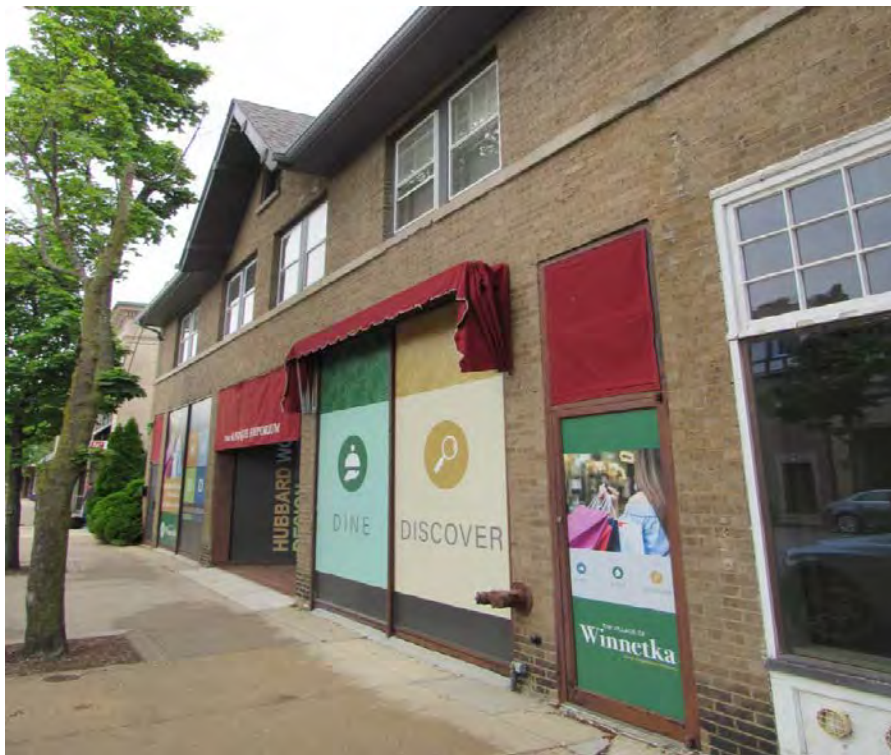
Figure 2 – Right side of frontage, facing northwest
