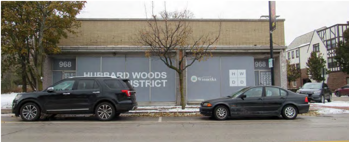
Figure 1 – Street frontage along Green Bay Road, facing west (November - 2019)
