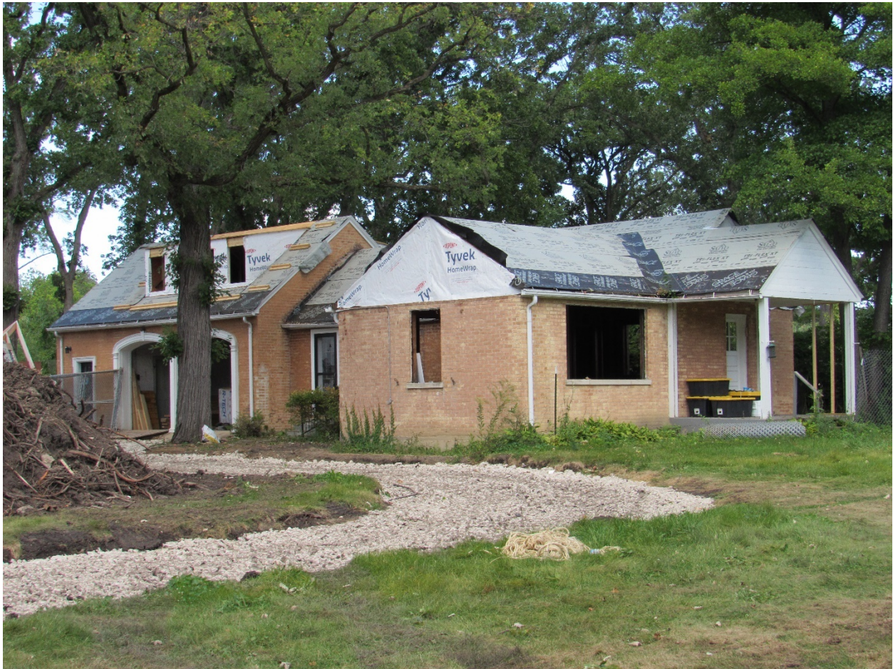
Figure 4 – Coach House on Subject Property (South and East Elevations)
