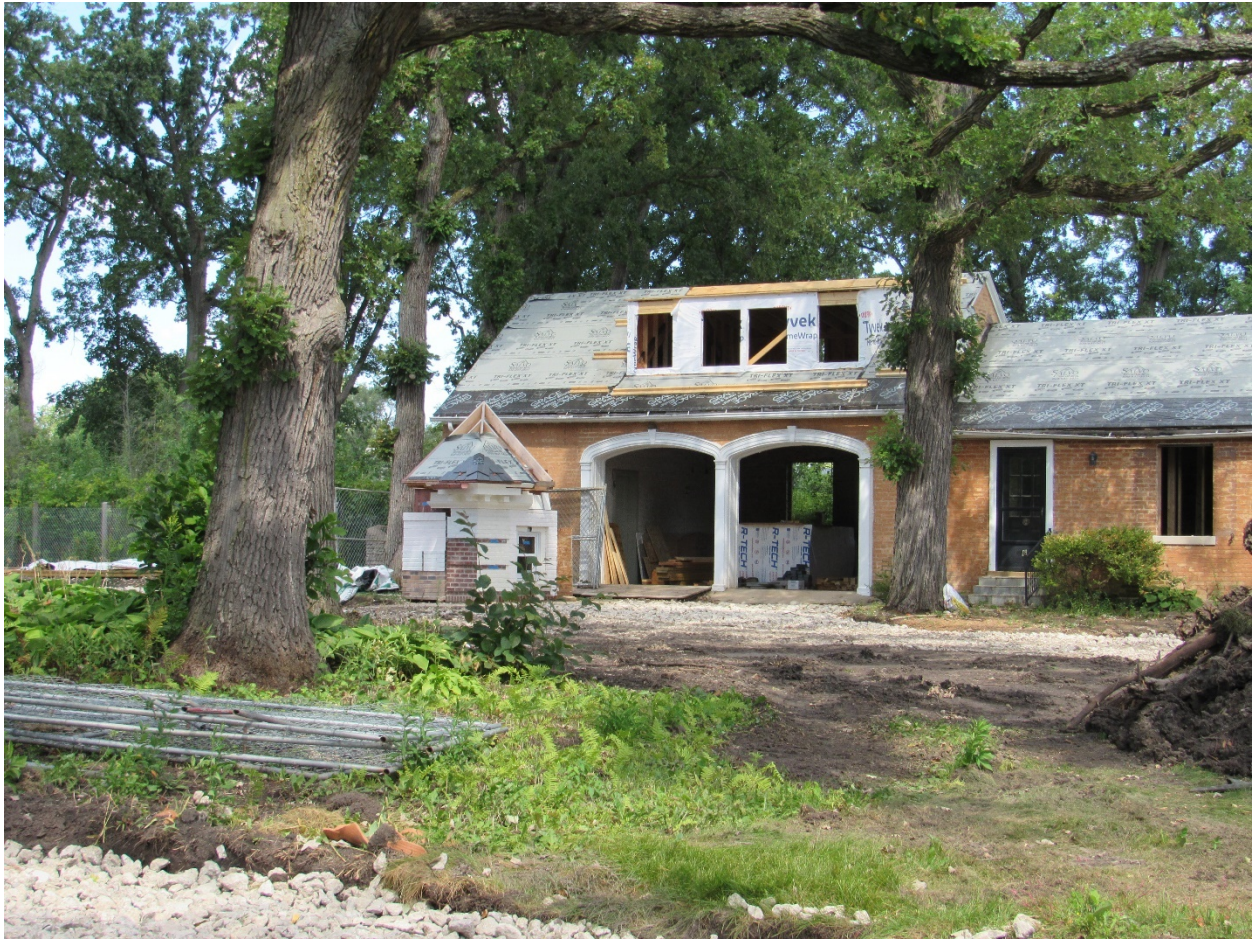
Figure 5 – Coach House on Subject Property (Partial South Elevation – Garage)
