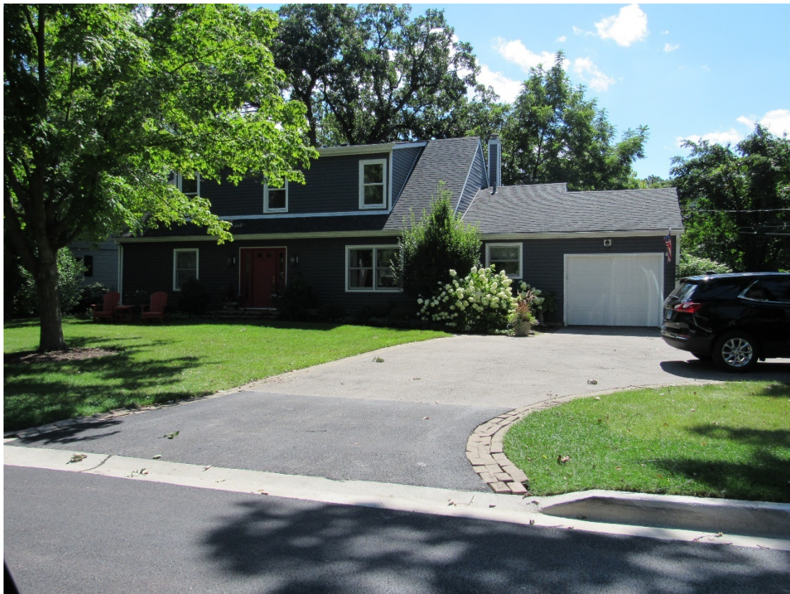
Figure 4 – Subject Property (Westerly Front Elevation – Gage Street)
