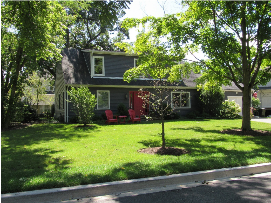
Figure 3 – Subject Property (Easterly Front Elevation – Gage Street)
