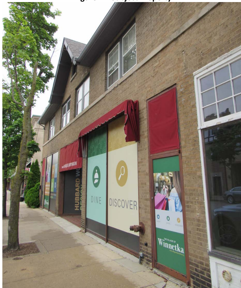
Figure 2 – Right side of frontage, facing northwest
