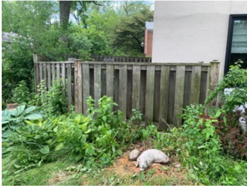
Figure 4 – Existing fence to be replaced on Subject Property
