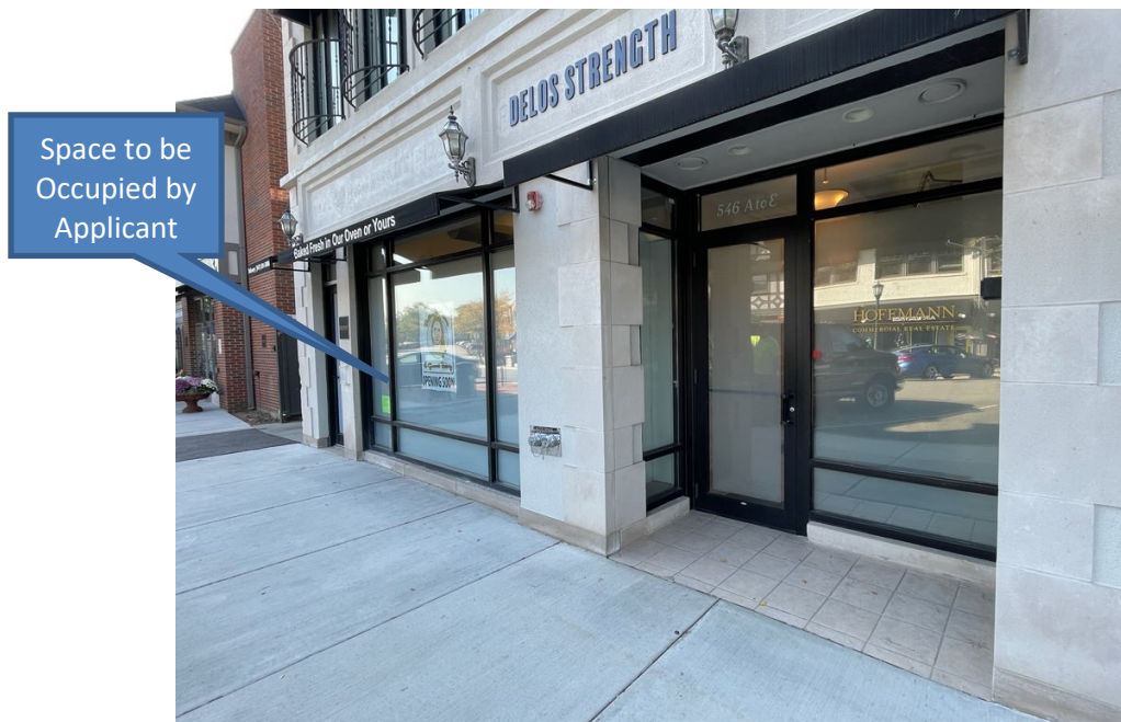
Figure 2 – Subject Property – Store Frontage and Neighboring Business
