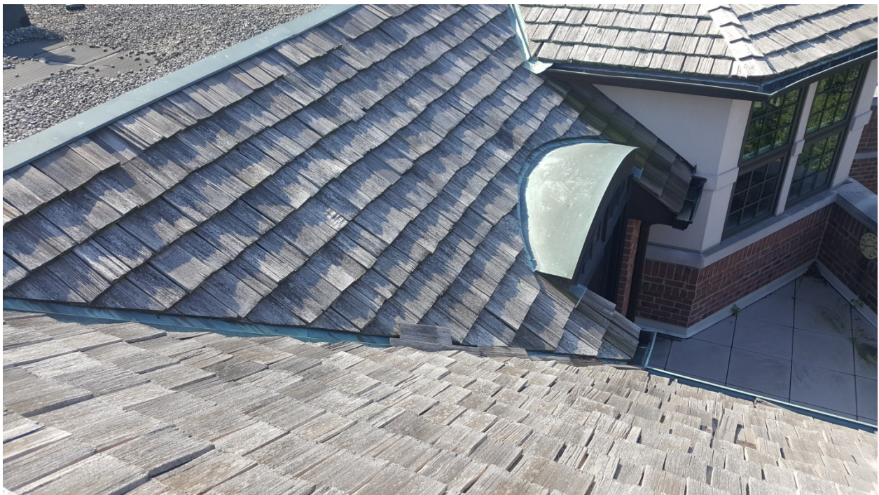
Figure 4 – Subject Property – Up close image of cedar roof shingles on roof gables.
