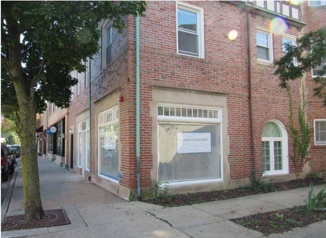
Figure 2 – Subject Property – Storefront along Green Bay Road, inner courtyard
