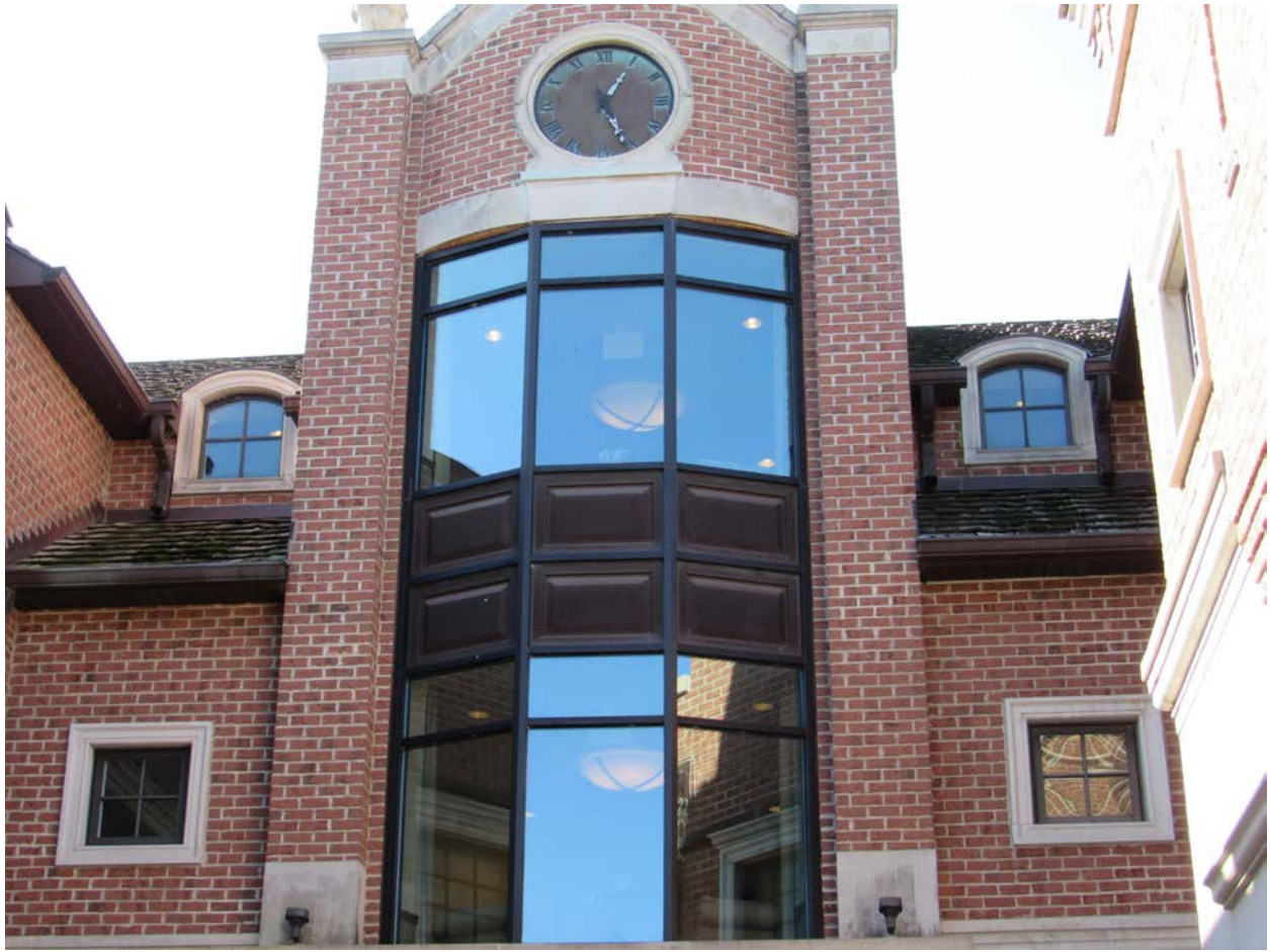
Figure 3 – Subject Property – Clock tower and visible roof segment along street frontage.
