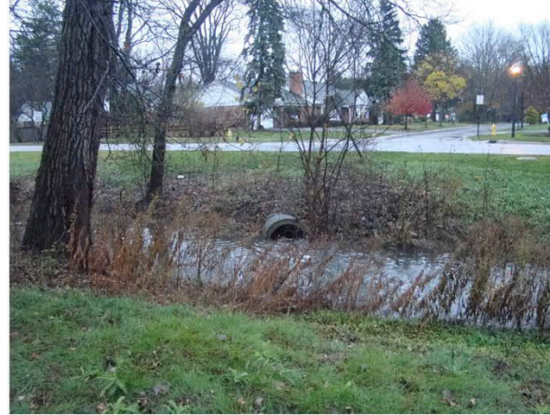
2. 36" outfall from Sunset Rd.
