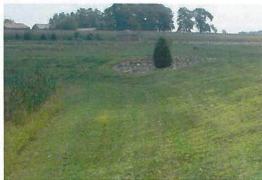
Figure 5.14: Unwanted vegetation - tree on embankment
