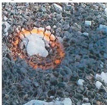
Figure 4.4: Marking a hole in gabion fabric
