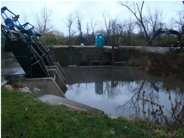
3. Winnetka Ave. PS upstream of levee
