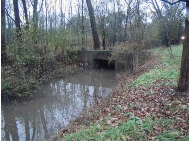
1. 8'x6' box outfall from Willow Rd.
