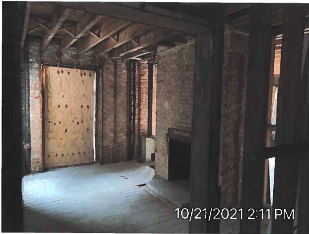
Interior finishes and mechanical systems shown removed from the interior of the home.
