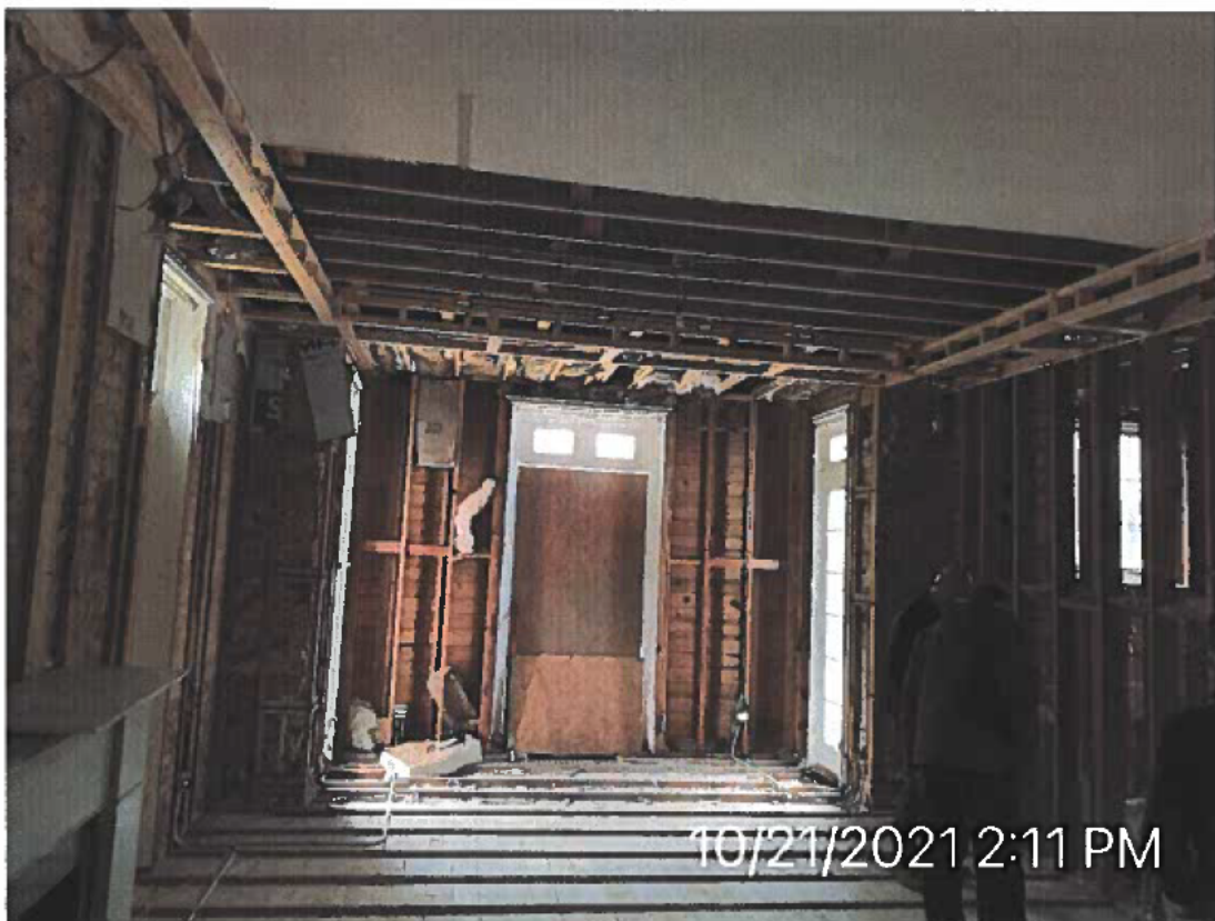
Interior finishes and mechanical systems shown removed from the interior of the home.
