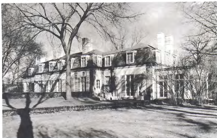
Terrace Side of Residence
