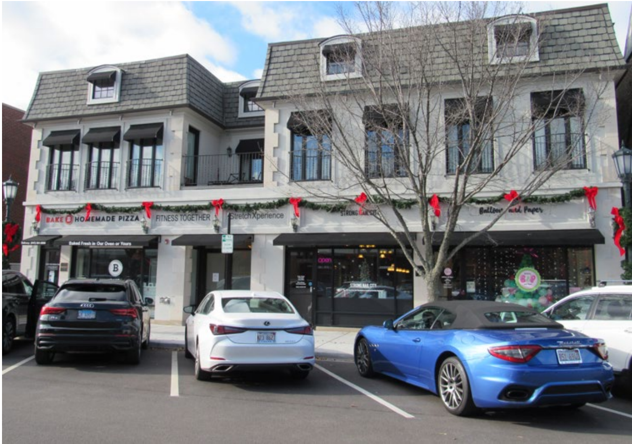
Figure 2 – Subject Property – Main building of applicant and other businesses along Lincoln Avenue
