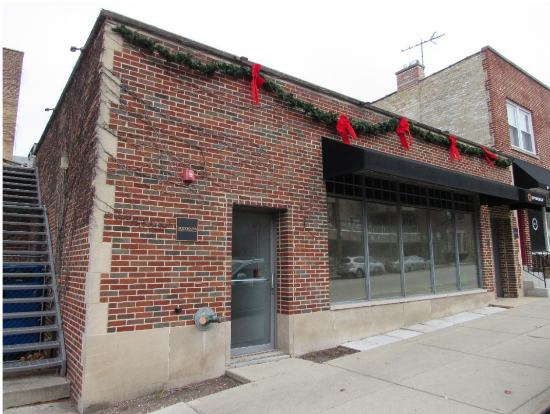
Figure 2 – Subject Property – Southwest corner of building along street façade of Oak Street
