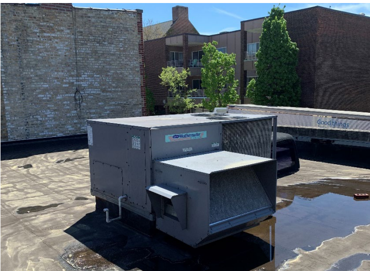
Existing Roof top Unit
