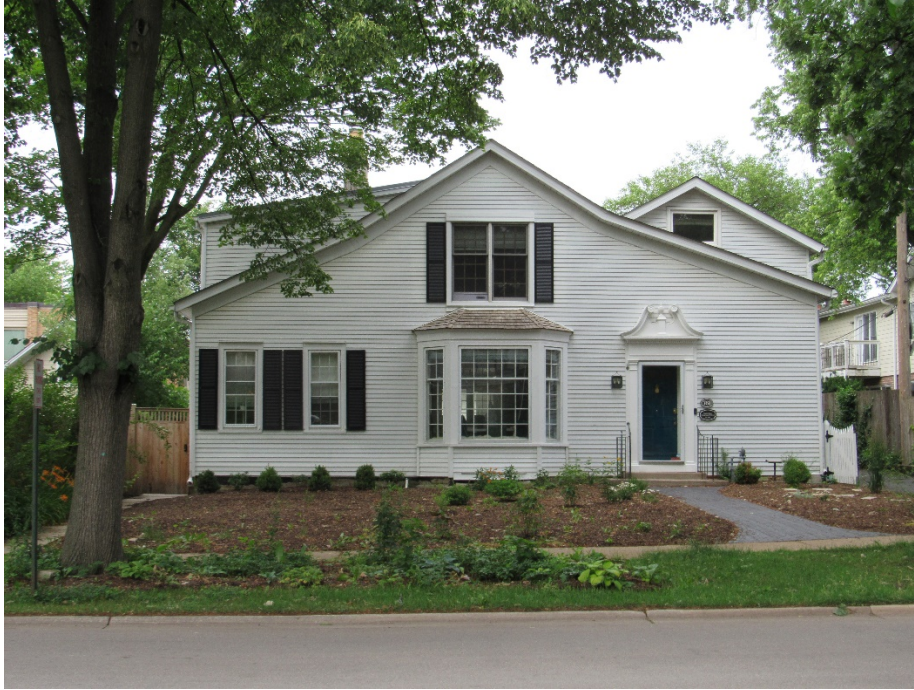
761 Cherry Street (multi-family residence to east)
