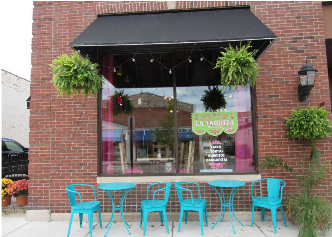
Figure 3 - Subject Property – Exterior window along frontage of Chestnut Street
