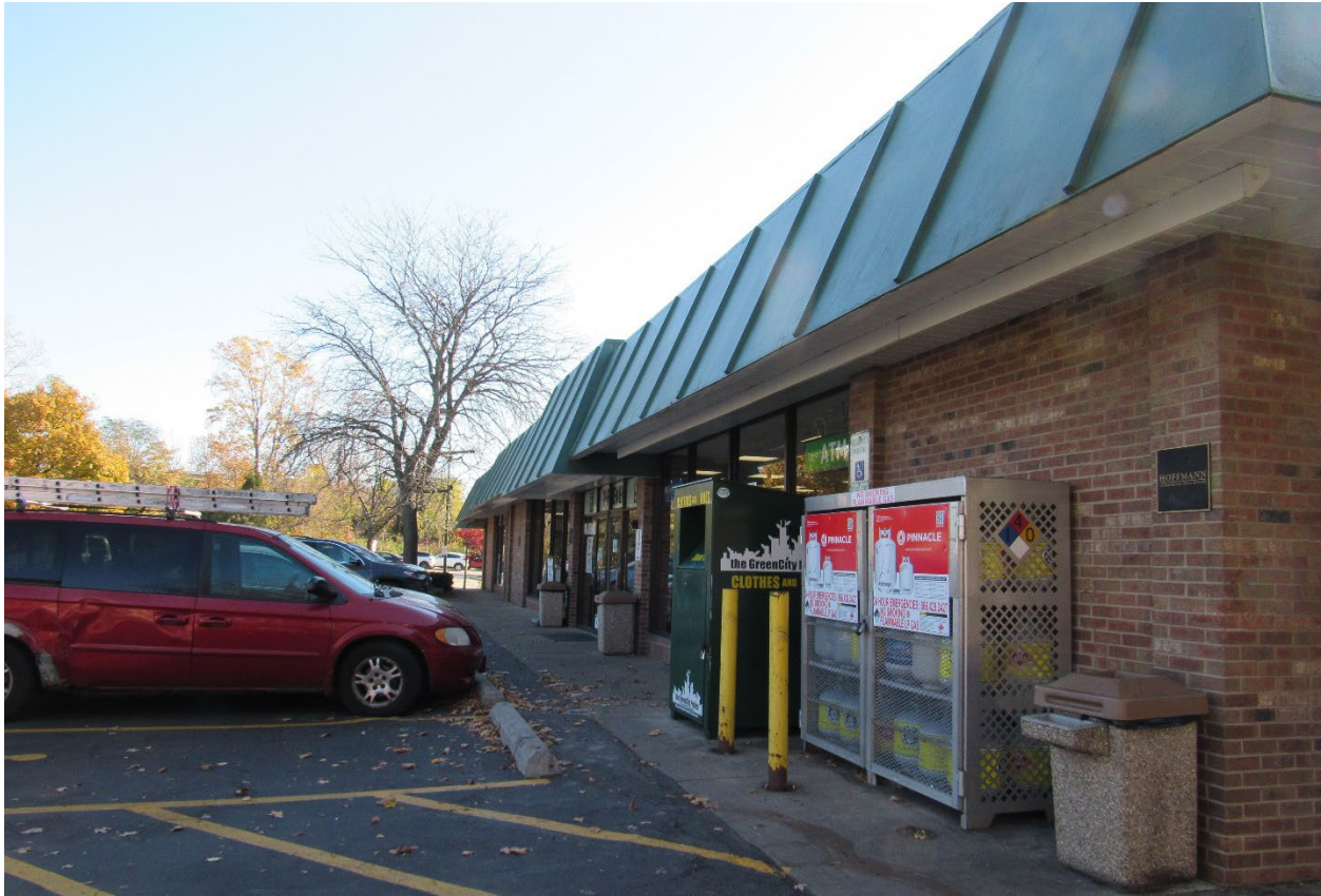
Figure 1 – Subject Property – North building façade along Green Bay Road
