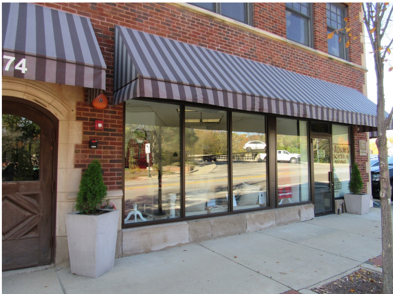
Figure 2 - Subject Property – Storefront window of business along east building façade of Green Bay Road
