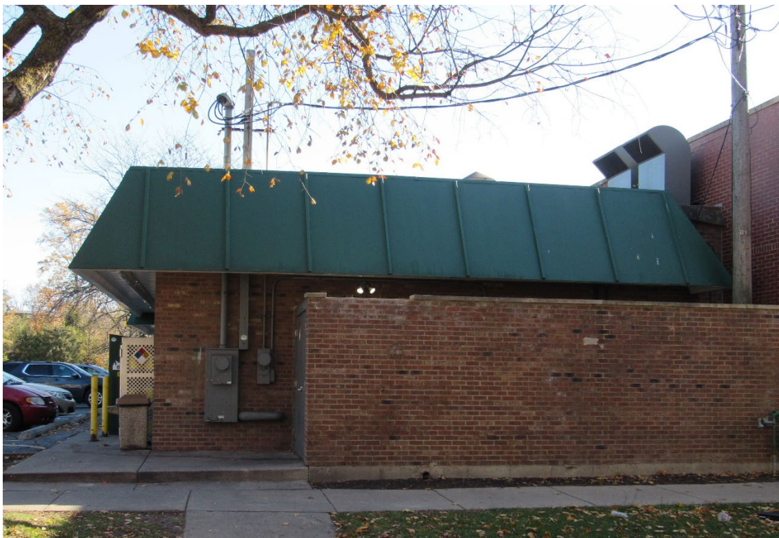
Figure 2 – Subject Property – West façade of building along Brier Street
