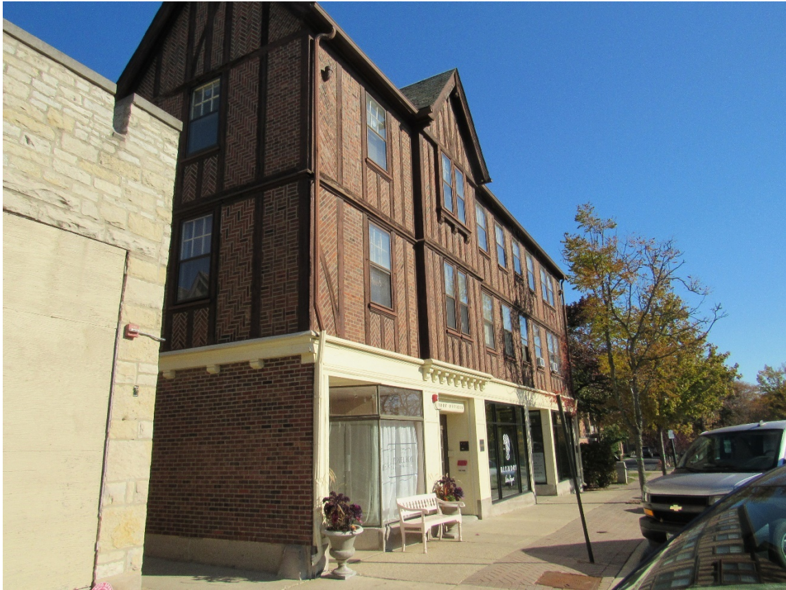
Figure 1 – Subject Property – Store frontage of building along Elm Street
