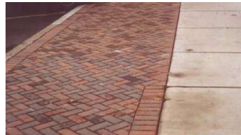
Typical concrete brick paver treatment in East/West Street Business District Figure 51d
