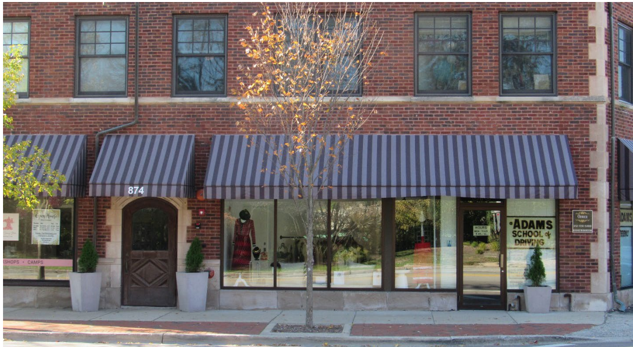
Figure 1 - Subject Property – Street frontage of the business along east building façade of Green Bay Road
