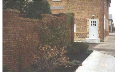
Typical masonry wall and landscape screening of service area Figure 77a
