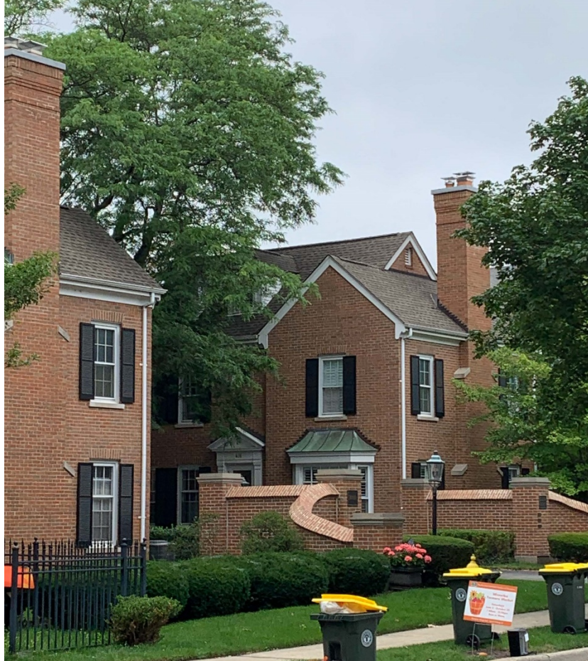
466-476 Linden Street (townhomes to northwest)
