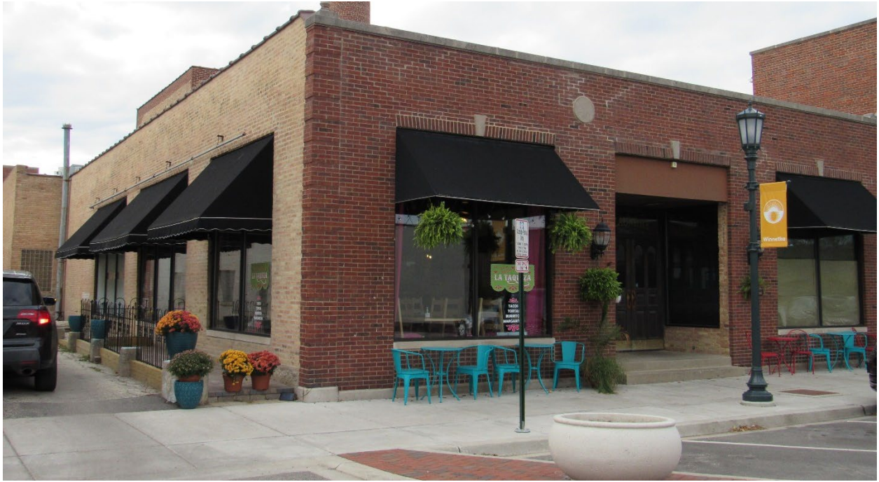
Figure 1 - Subject Property – Street frontage of the business along east building façade of Chestnut Street
