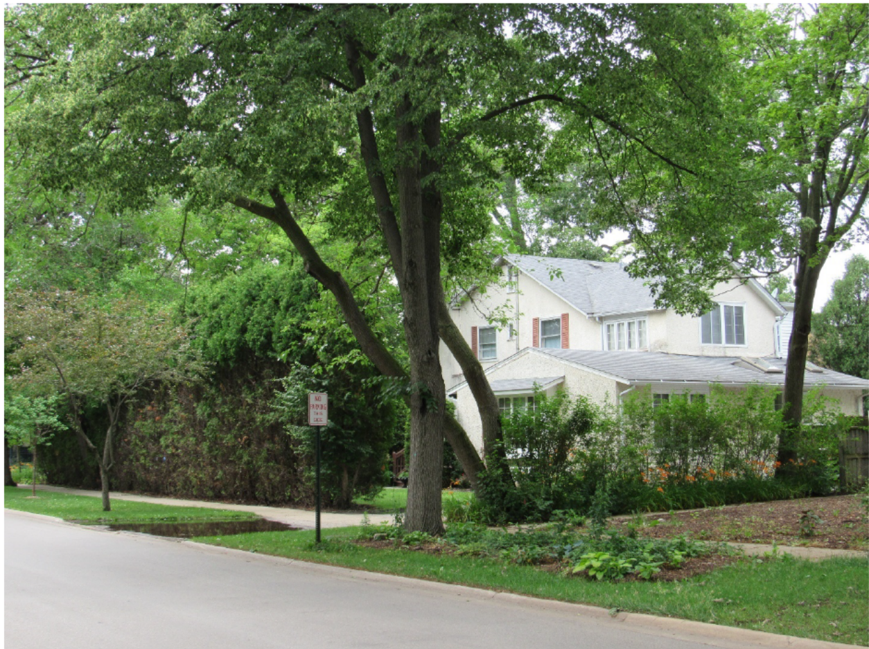
Figure 2 – Subject Property – Looking Northwest
