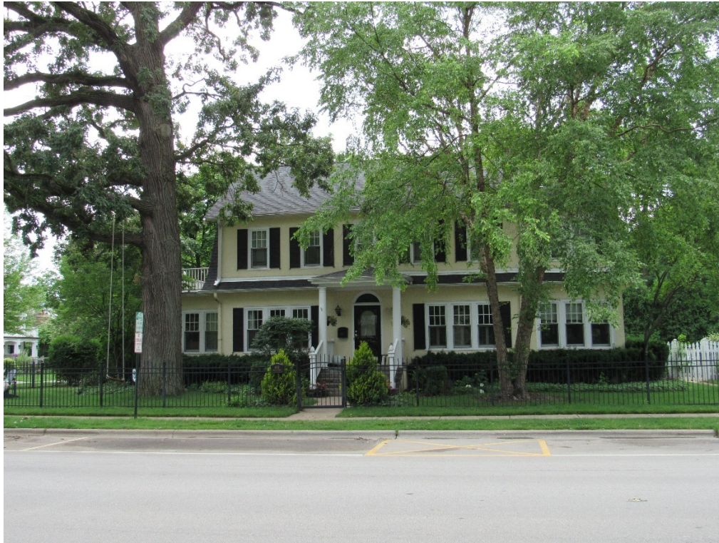
458 Linden Street (single family home to west)
