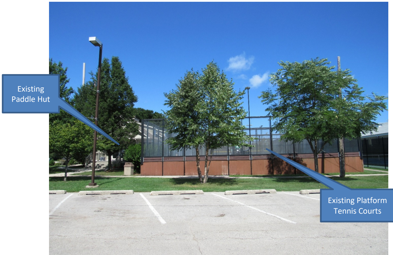
Figure 3 – South Elevation of Existing Platform Tennis Courts and Paddle Hut
