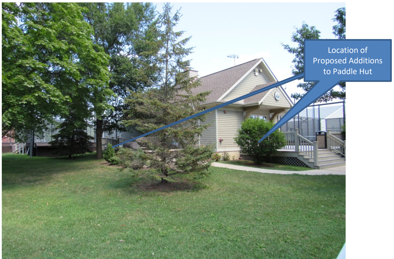
Figure 5 – Existing Paddle Hut (looking northeast)
