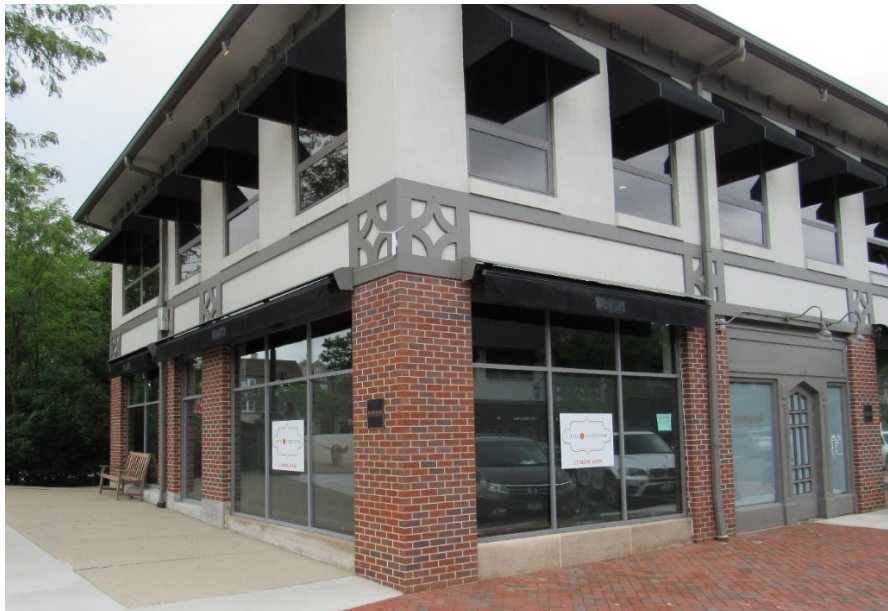
Figure 1 – Subject Property – Store frontage at corner of Elm Street and Lincoln Avenue
