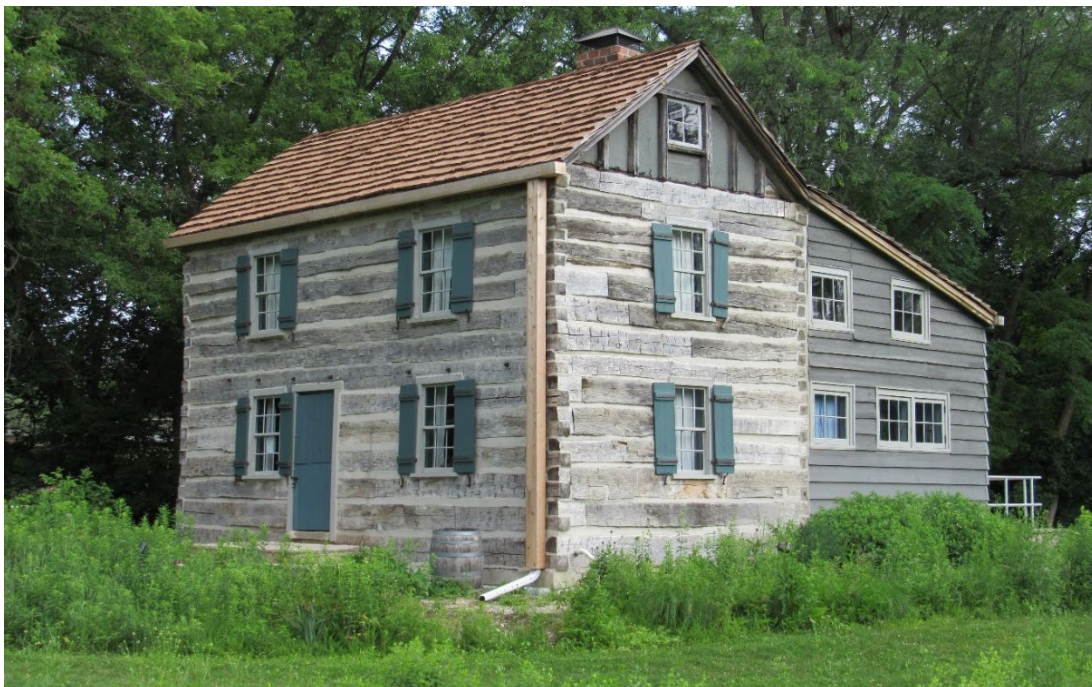
Figure 1 – Subject Property – West façade of Log House
