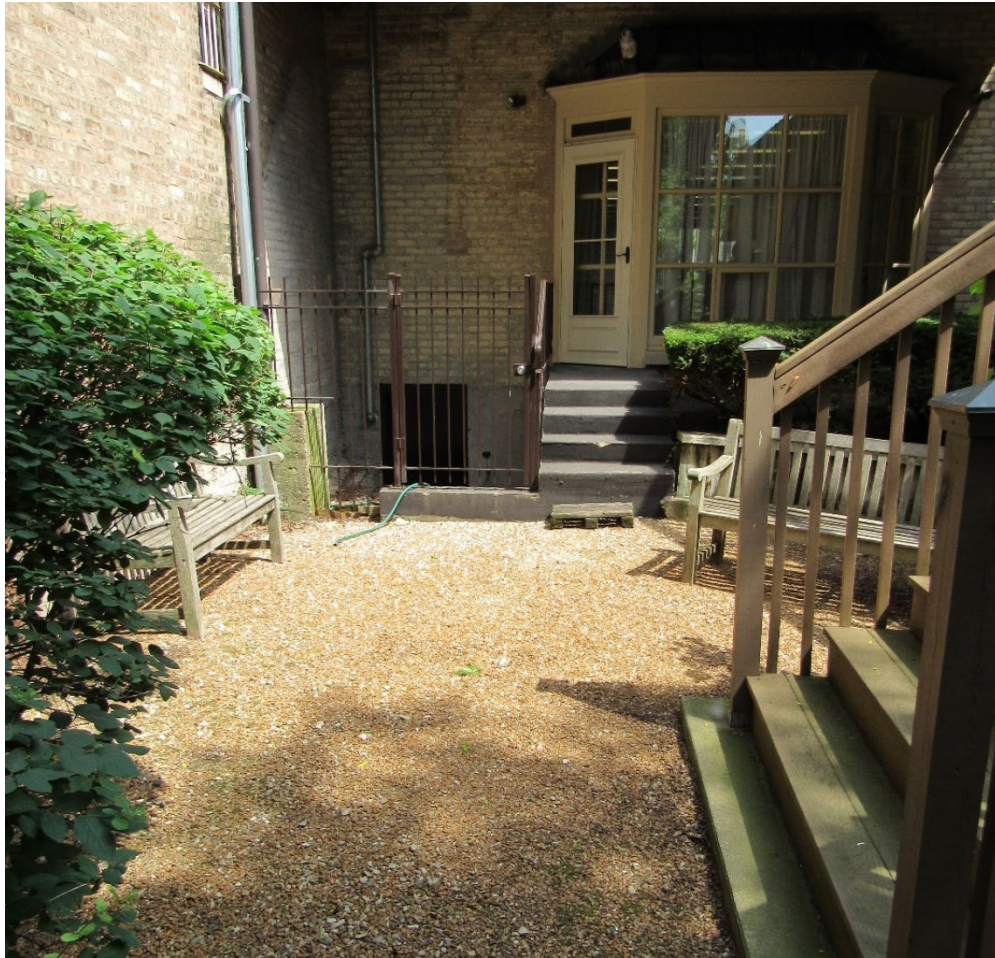
Figure 3 – Subject Property – Gravel sitting area at rear building entrance (July 2021)
