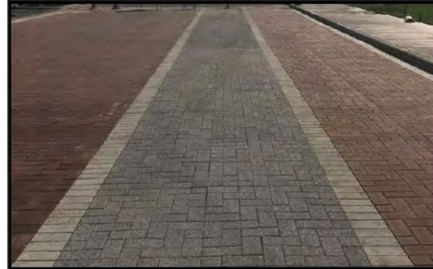
Existing Parking and Drive Pavers - Unilock Eco-Priora
