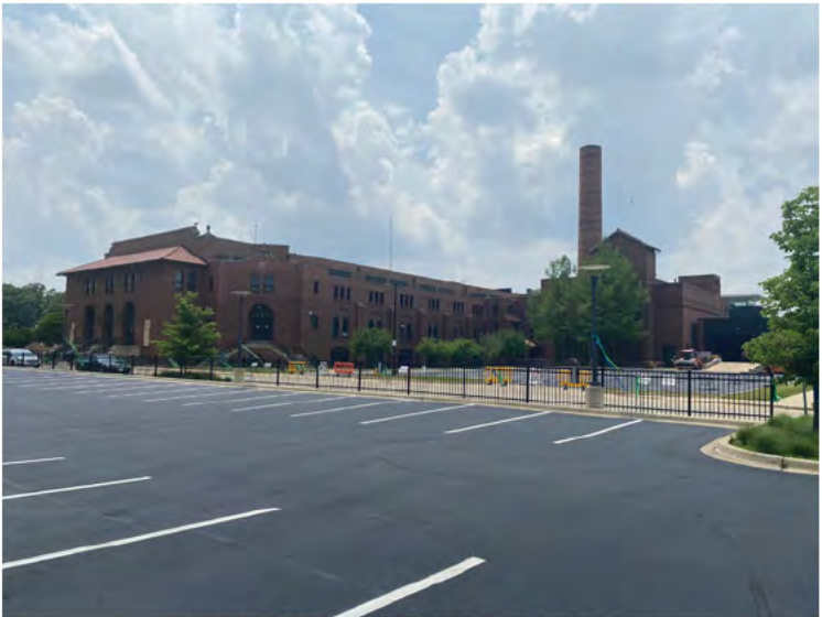
EXISTING GATES GYM - NW CORNER
