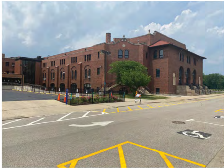
EXISTING GATES GYM - NE CORNER
