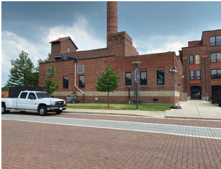
EXISTING FACADE- NORTH ELEVATION
