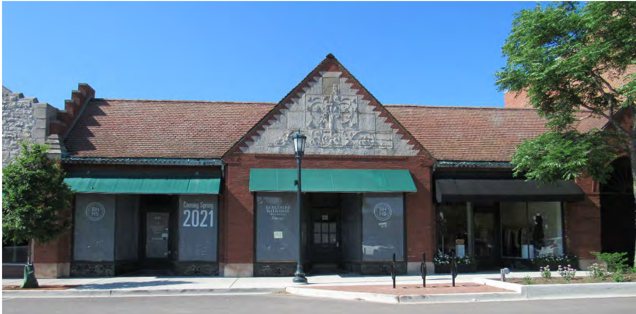
Figure 1 – Subject Property – Street frontage along Elm Street (June 2021)
