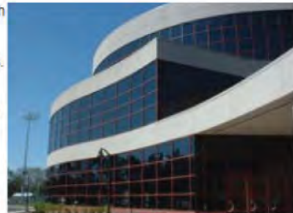
Project: Allegan High School - Entry Location: Allegan, MI Architect: TMP Associates Inc Glazing Contractor: Commercial Glass & Glazing
