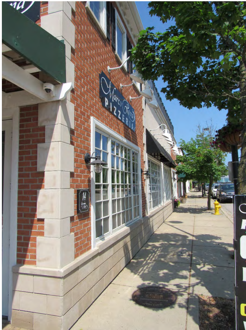
Figure 2 – Subject Property – Exterior façade along Green Bay Road (June 2021)
