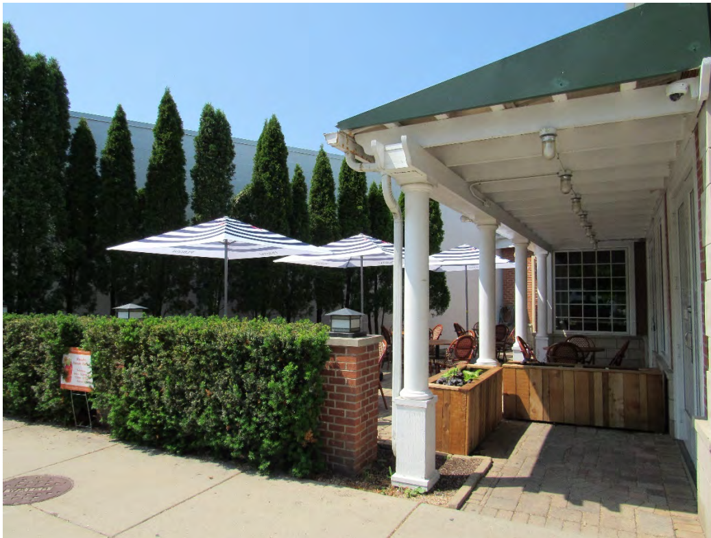
Figure 3 – Subject Property – Covered porch entrance and outdoor dining patio (June 2021)
