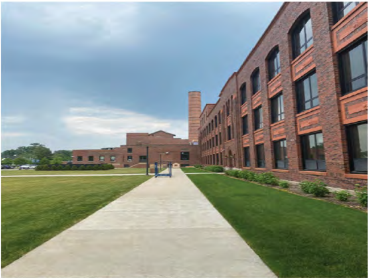
EXISTING GATES GYM - WEST ELEVATION
