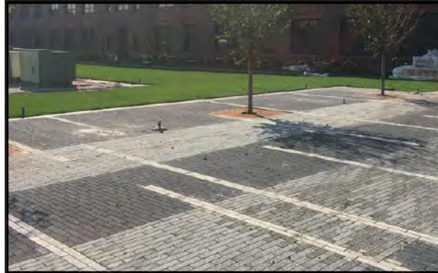
Existing Plaza Permeable Pavers - Unilock Promenade
