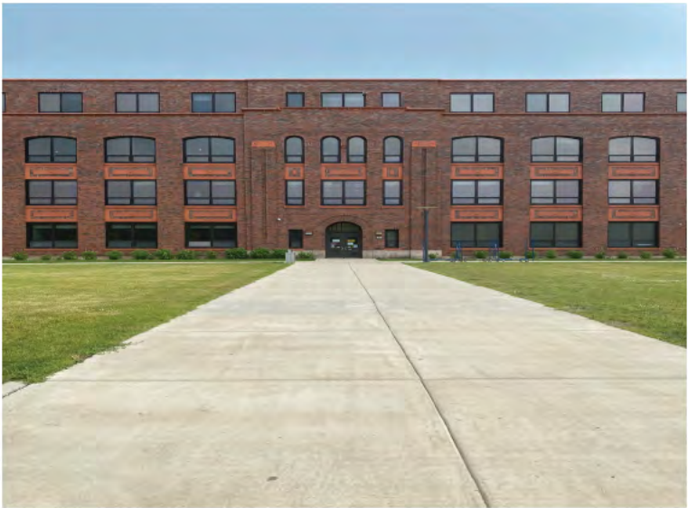
EXISTING FACADE - NORTH ELEVATION
