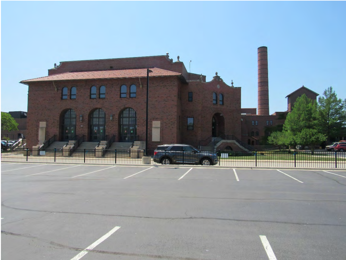
Figure 2 – Subject Property (East Elevation of Gates Gymnasium and Boiler Plant)
