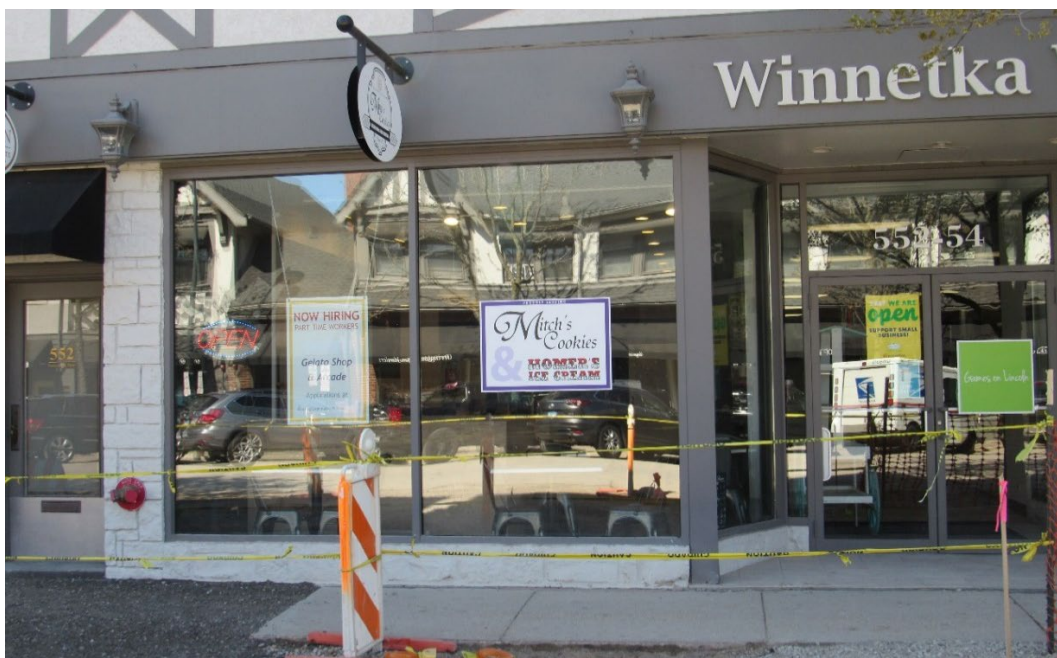
Figure 1 – Subject Property – Store frontage of Subject Property along Lincoln Avenue
