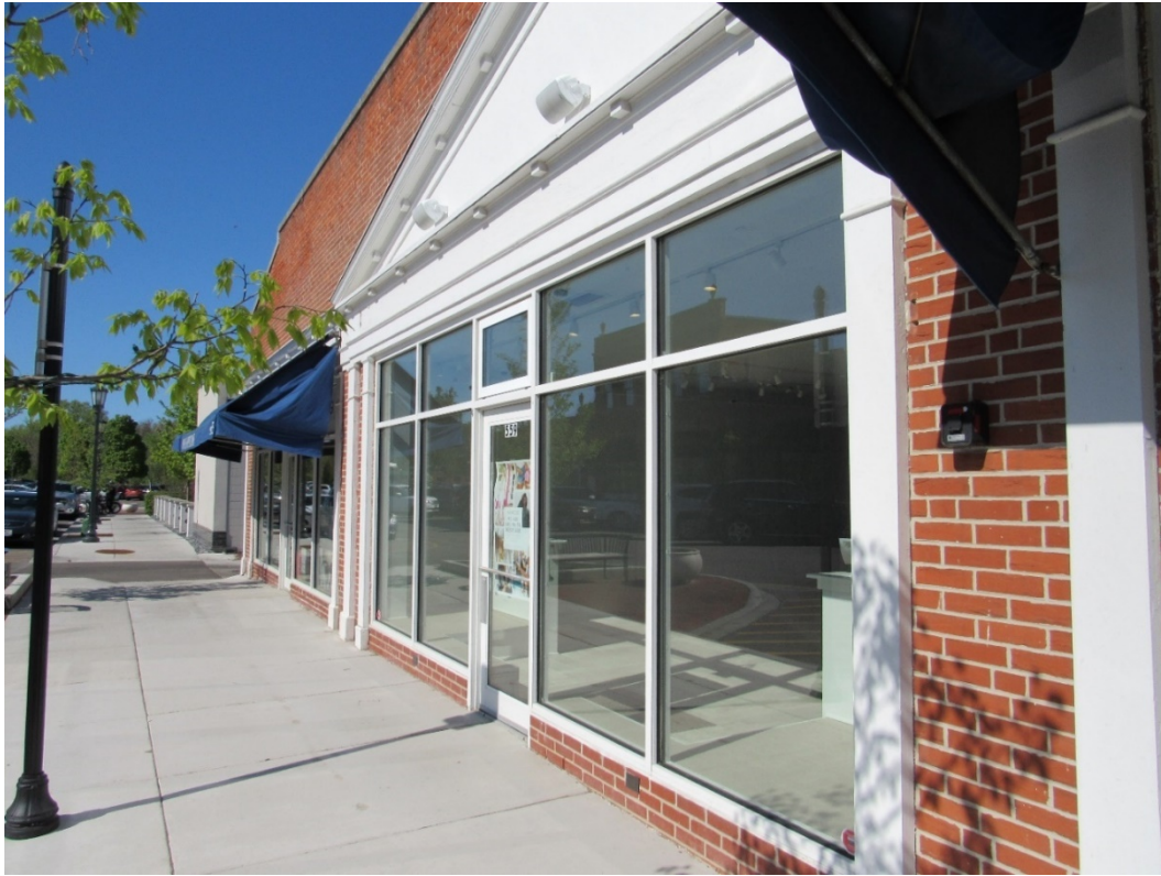
Figure 4 – Subject Property – New storefront along Chestnut Street, facing north (May 2021)
