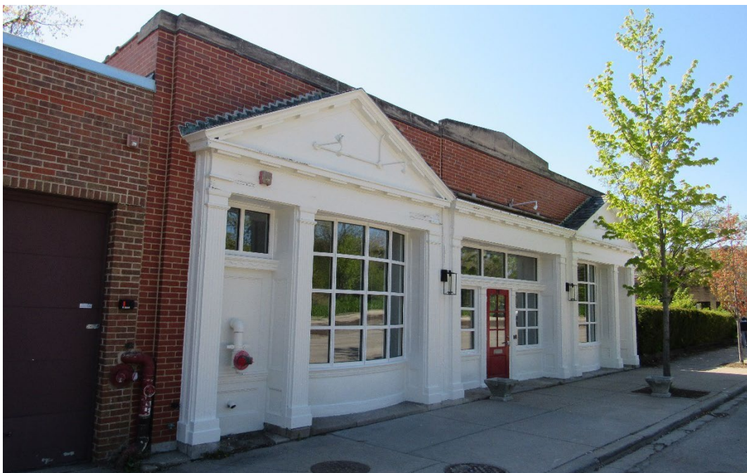
Figure 3 – Subject Property – Street frontage along Green Bay Road facing north (May 2021)
