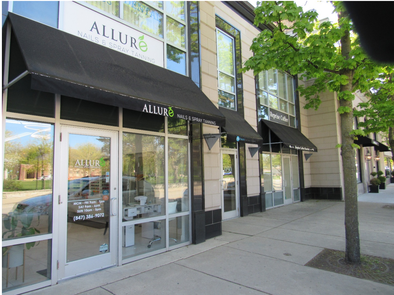
Figure 2 – Subject Property – Existing Awnings to be Replaced (May 2021)
