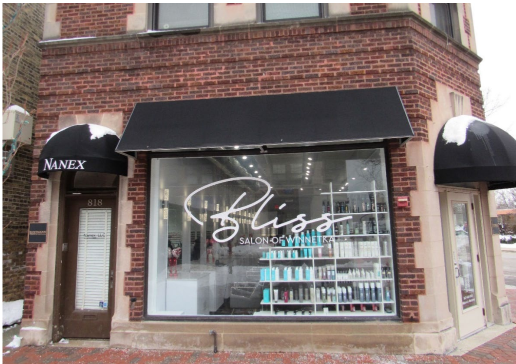
Figure 2 – Subject Property – North façade along Elm Street (February 2021)
