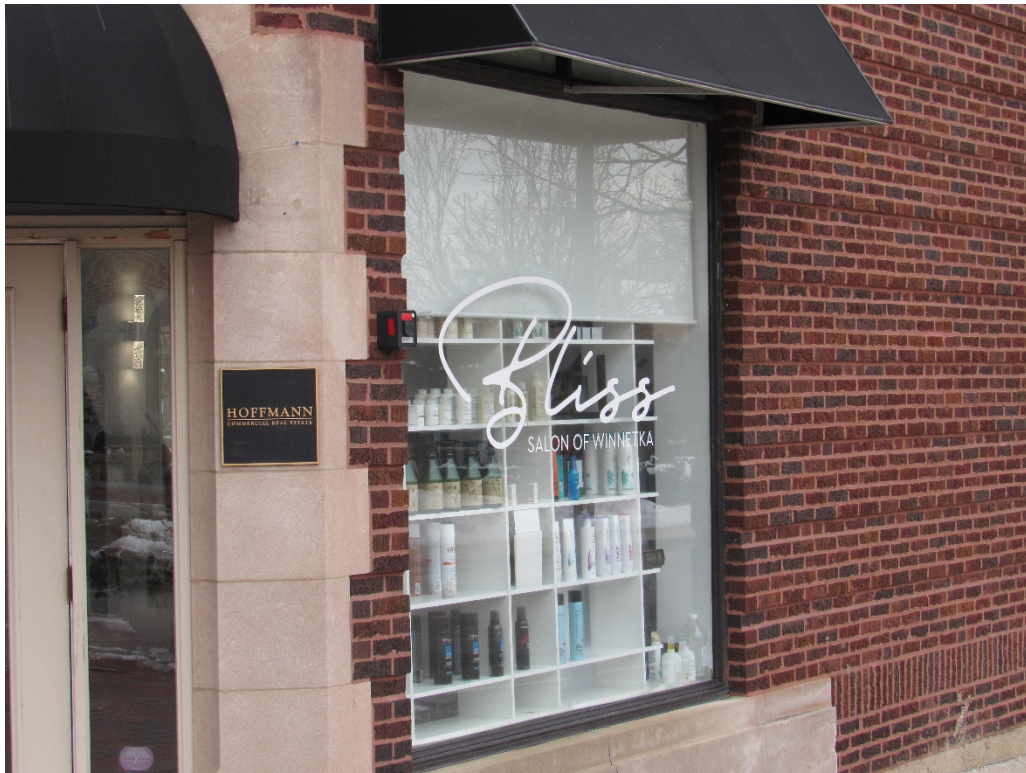
Figure 3 – Subject Property –West façade along Chestnut Street (February 2021)
