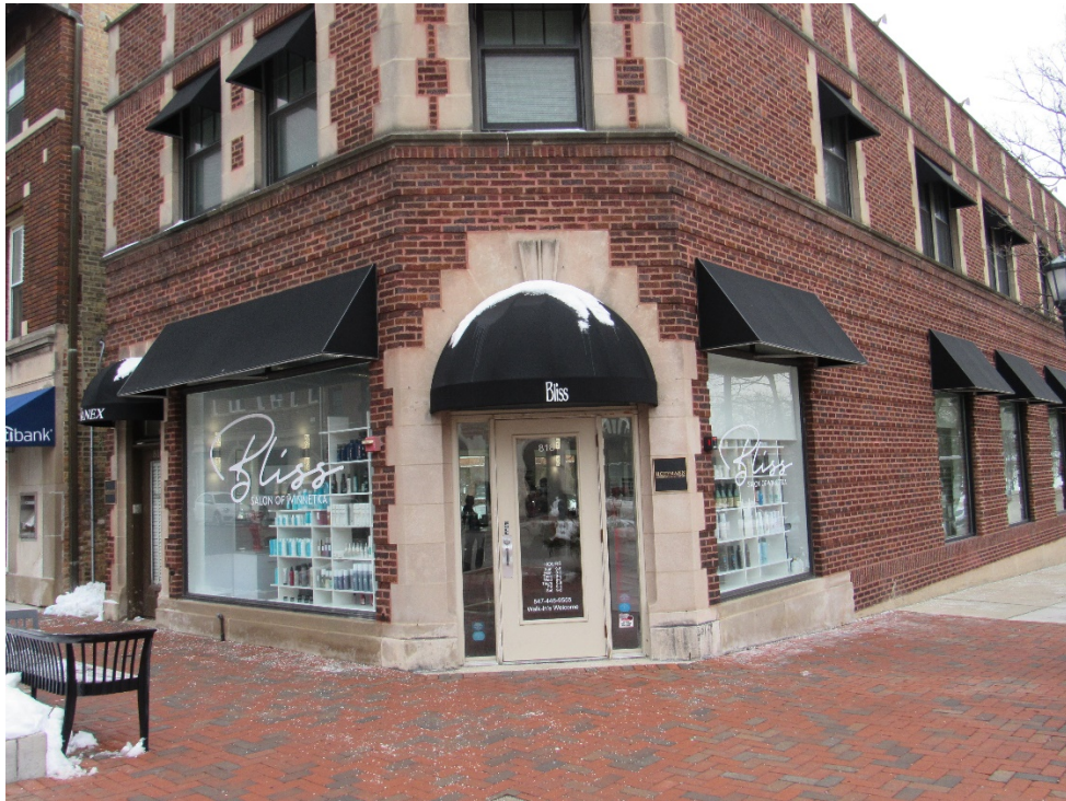
Figure 1 – Subject Property – Chestnut and Elm Street intersection, north and west facades (February 2021)
