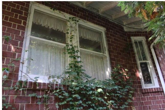
East elevation windows.
