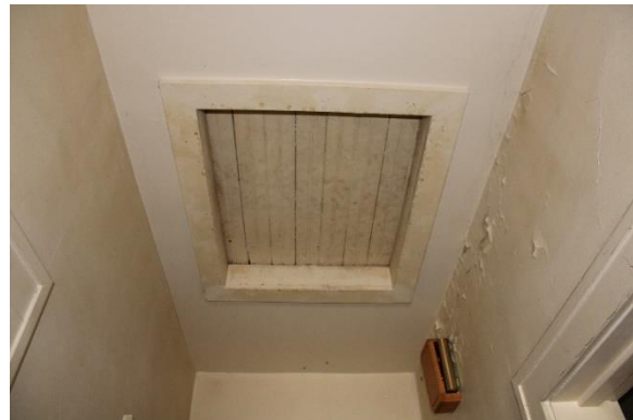
Trapdoor to attic in hallway ceiling.
