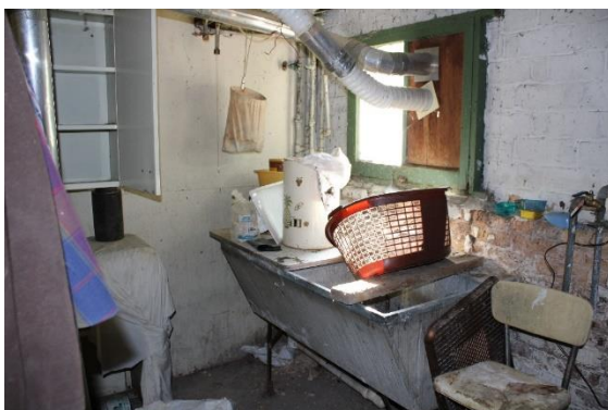
Original basement sink.
