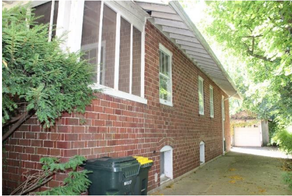
West elevation, view southeast.
