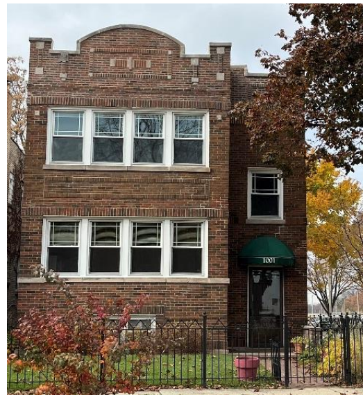
Representative two-flat designed by Lyman Allison, located at 1001 S. Humphrey, Oak Park.
