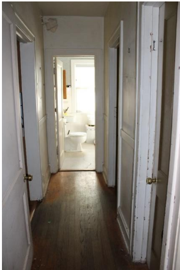
Hallway, view toward bathroom.
