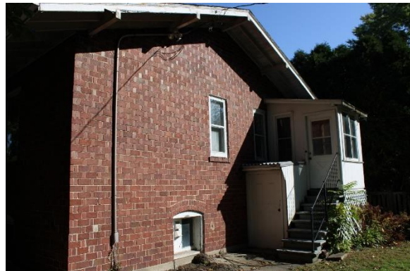
Rear elevation, view northeast.
