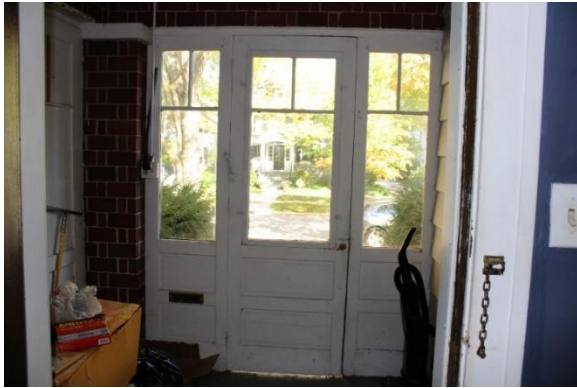
Front storm door.
