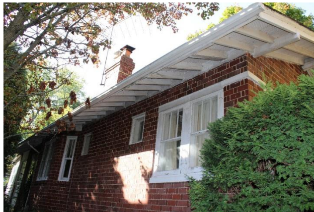
East elevation, view southwest.
