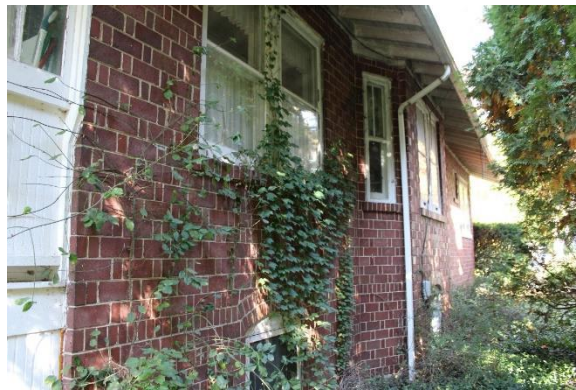
East elevation, view northwest.
