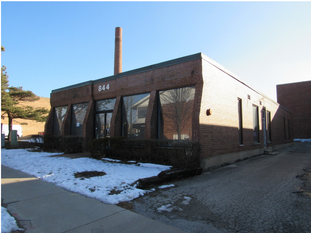
Figure 2 – Subject Property – North and west façades along Spruce Street (January 2021)
