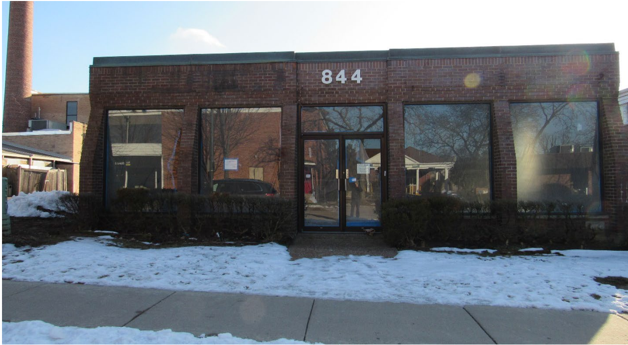
Figure 1 – Subject Property – North façade along Spruce Street (January 2021)
