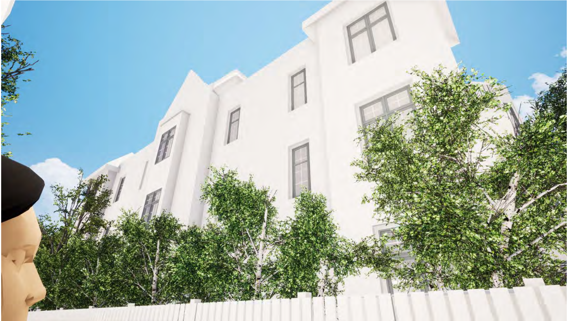
View Perspective from the north neighbor looking to the SE
