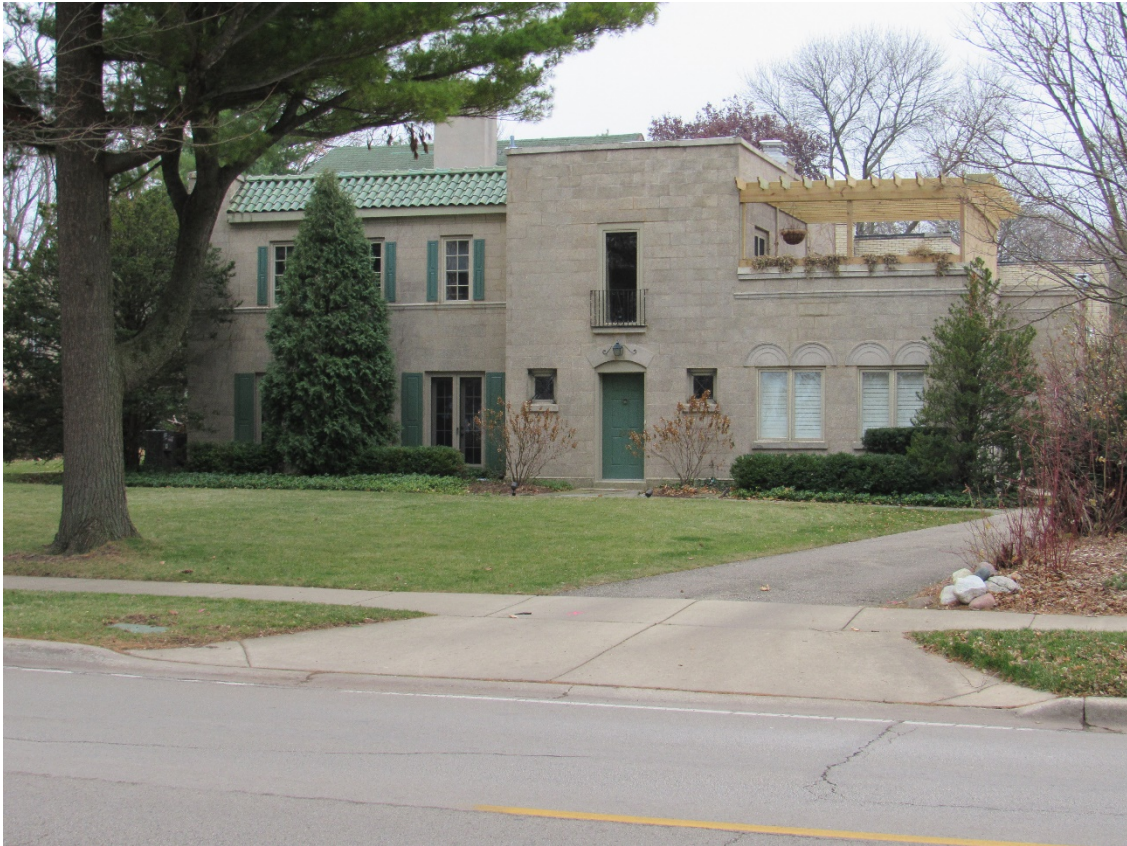
Figure 4 – Subject Property (Front Elevation – Sheridan Road)
