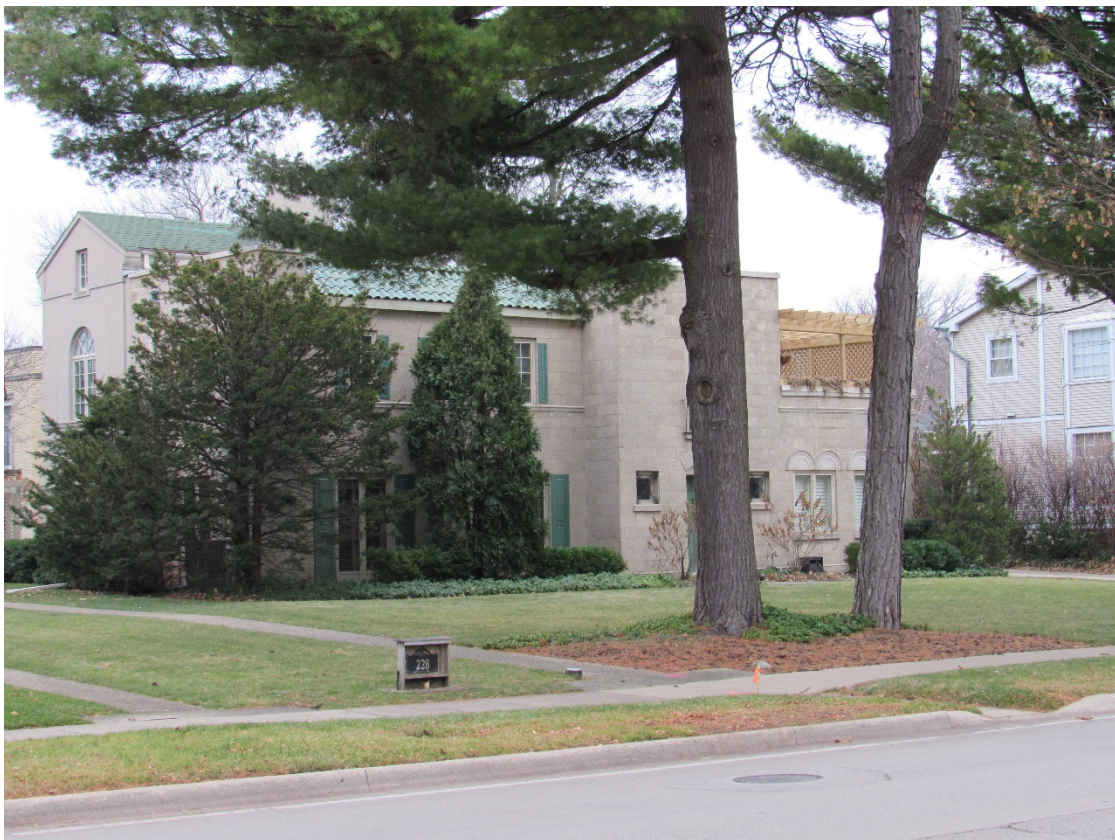
Figure 5 – Subject Property (Southerly Front Elevation)
