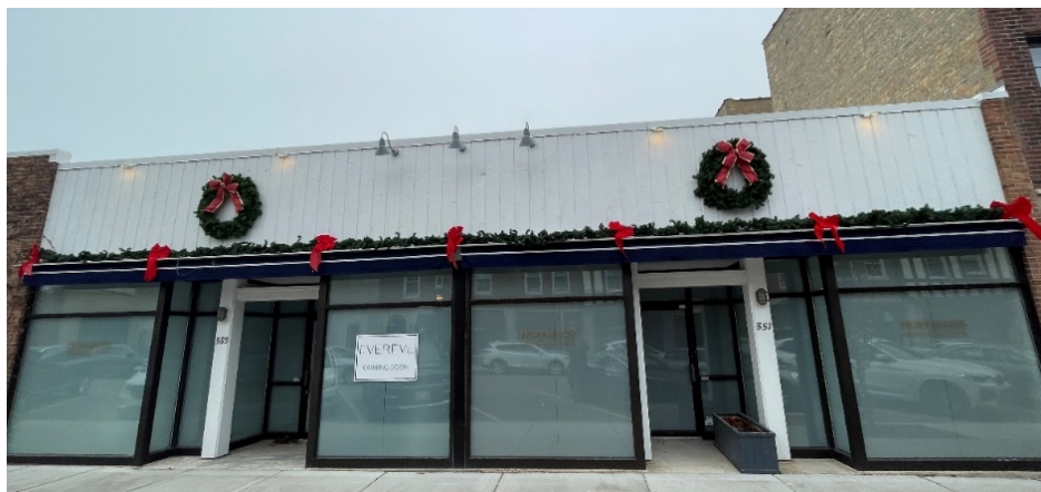
Figure 1 – Subject Property – Street frontage of building along Chestnut Street
