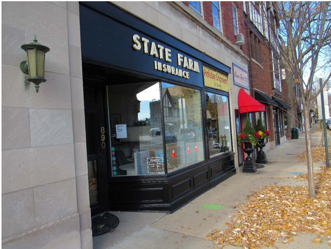
Figure 3 – Storefront façade along Green Bay Road facing Northwest
