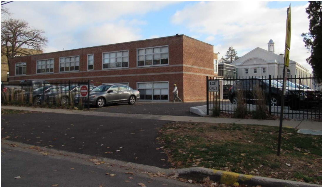
Figure 1 – Subject Property – Middle school building along Forest Street, facing east
