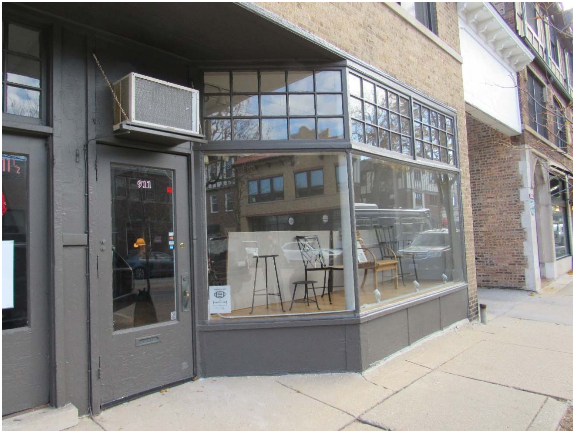
Figure 1 – Subject Property – Street frontage along Green Bay Road
