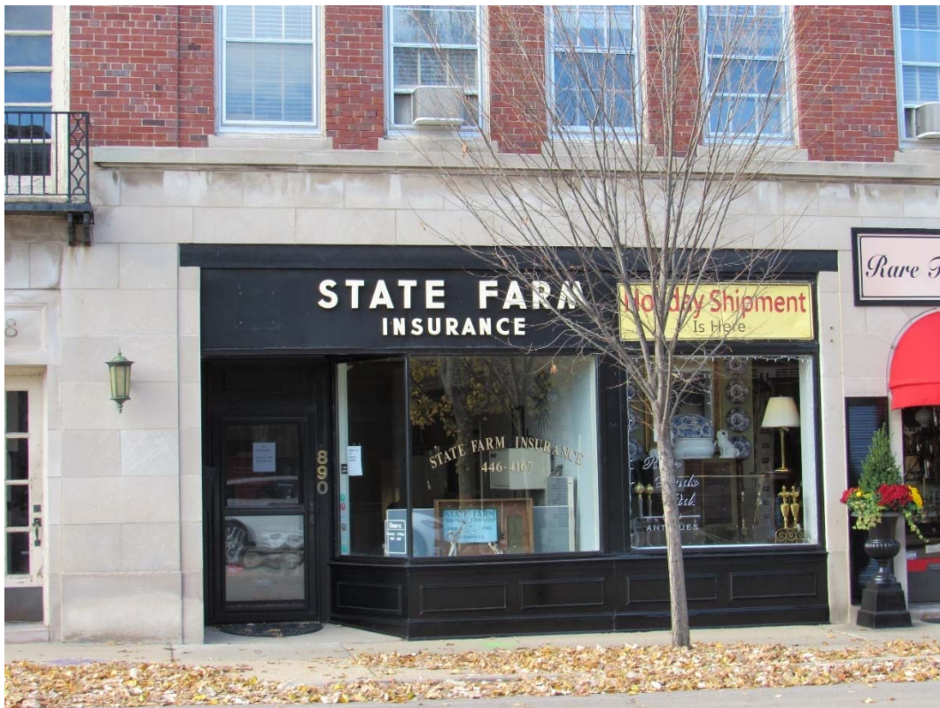
Figure 2 – Subject Property – Applicant's street frontage along Green Bay Road
