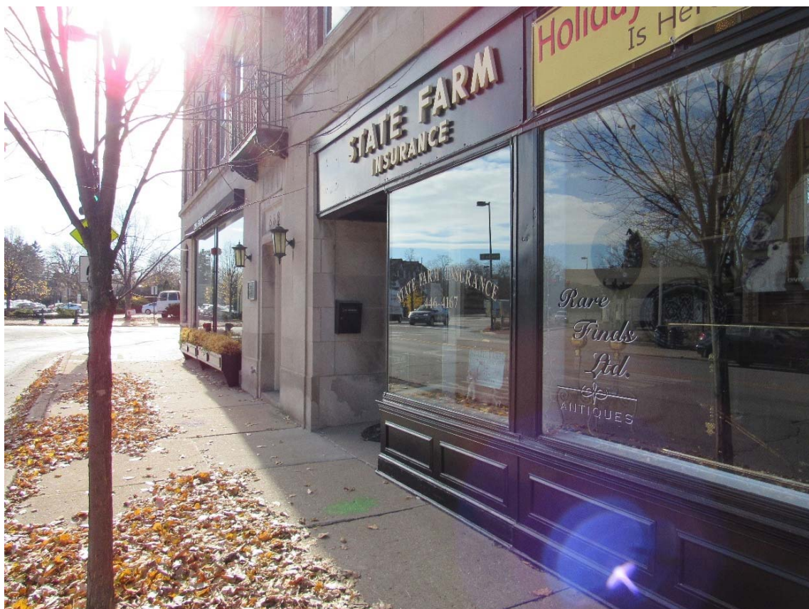
Figure 3 – Storefront façade along Green Bay Road facing Southwest
